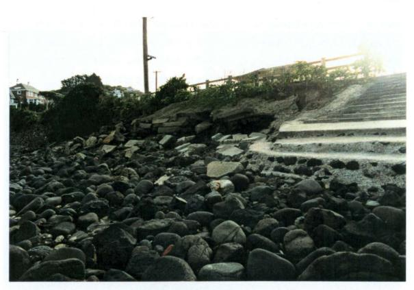
Plate 5.14: March 21. Toe of structure has eroded.
