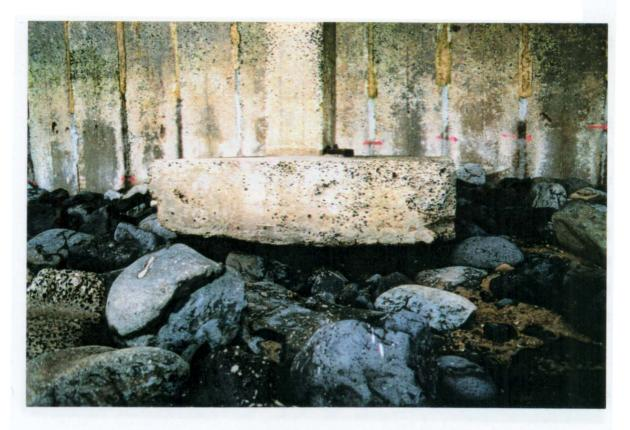
Plate 5.16: Seawall in the vicinity of Profile 2. April 30. Note replastered cracks at base of seawall.
