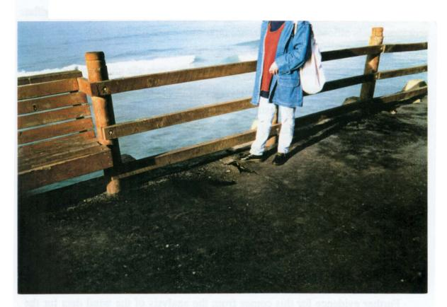
Plate 5.10: Development of a hole in the footpath atop the seawall at <u>St. Clair.</u>
