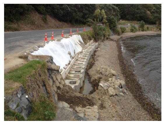
Figure 3.1: Example of the concrete block wall to be constructed at the toe of the slope face as a sediment control measure (Source: AECOM, 2015)
