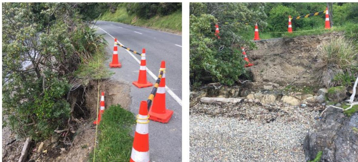
Figure 2.4: Photographs of Landslip 2 along Shelly Bay Road. Photo on left: View of the head scarp looking north. Photo on right: View of the slip face from the base of the slope in the CMA. (Source: T+T, 2016)
