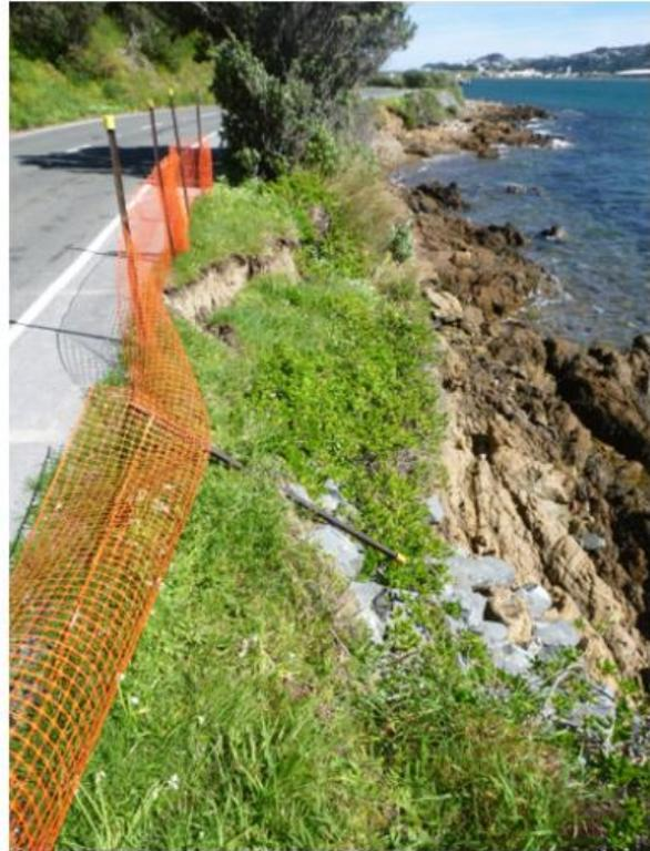
*Photographs 1 and 2: Photographs of Landslip 1 along Shelly Bay Road. Photograph on left: View of the head scarp looking north. Photograph on right: View of the head scarp and landslip debris looking south (Source: T+T, 2016)*
