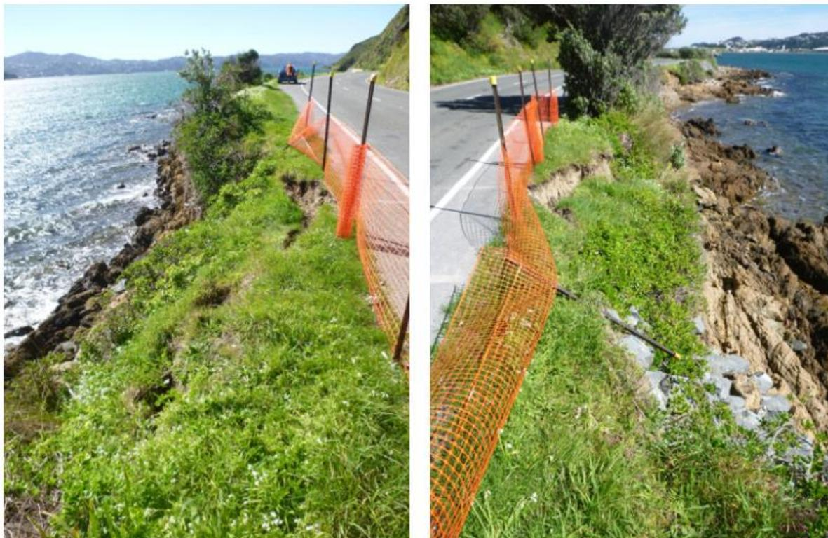
Figure 2.3: Photographs of Landslip 1 along Shelly Bay Road. Photo on left: View of the head scarp looking north. Photo on right: View of the head scarp and landslip debris looking south (Source: T+T, 2016)
