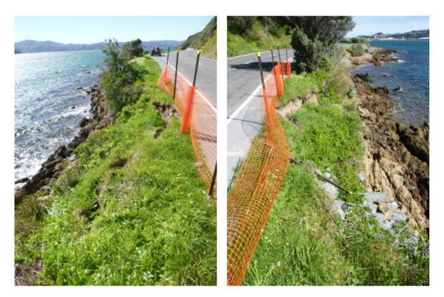
Figure 2.3: Photographs of Landslip 1 along Shelly Bay Road. Photo on left: View of the head scarp looking north. Photo on right: View of the head scarp and landslip debris looking south (Source: T+T, 2016)
