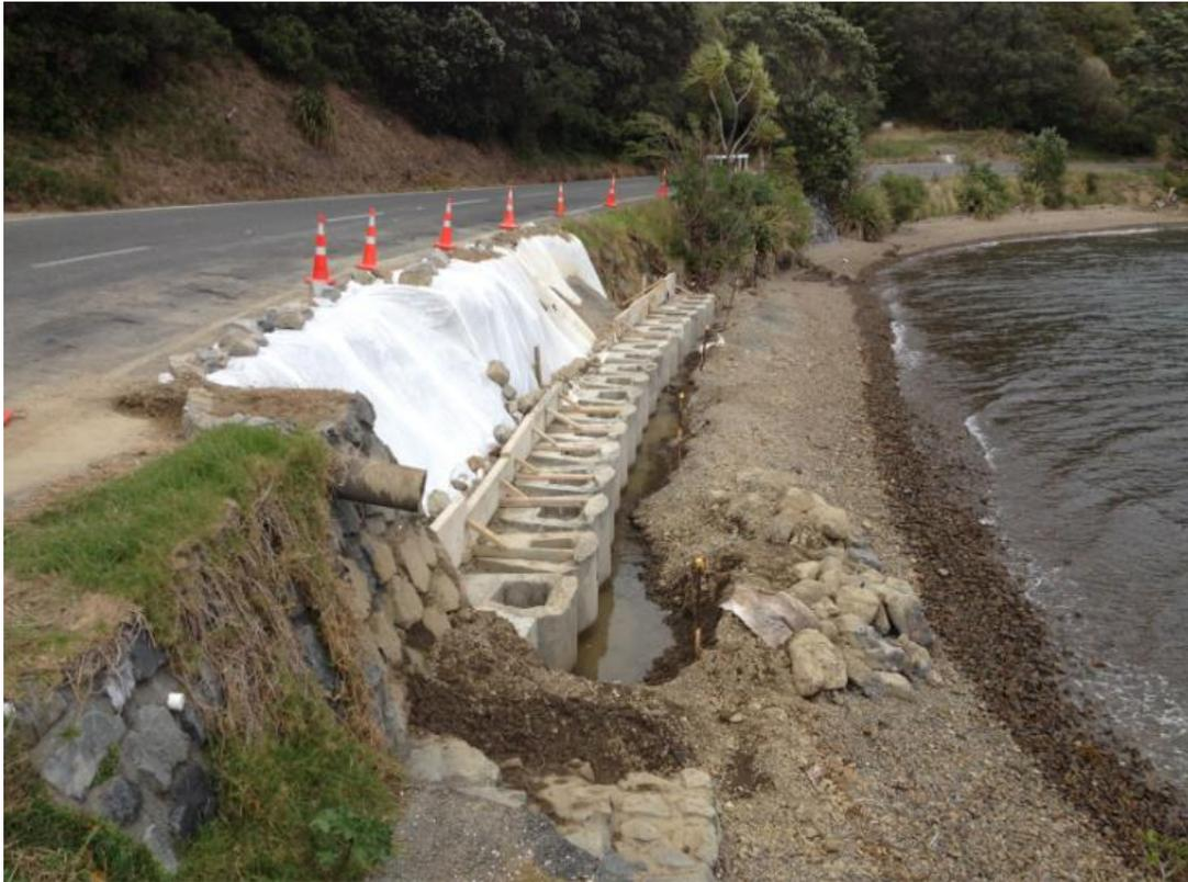
Figure 3.1: Example of the concrete block wall to be constructed at the toe of the slope face as a sediment control measure (Source: AECOM, 2015)
