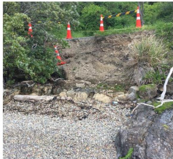
*Photographs 3 and 4: Photographs of Landslip 2 along Shelly Bay Road. Photograph on left: View of the head scarp looking north. Photograph on right: View of the slip face from the base of the slope in the CMA. (Source: T+T, 2016)*
