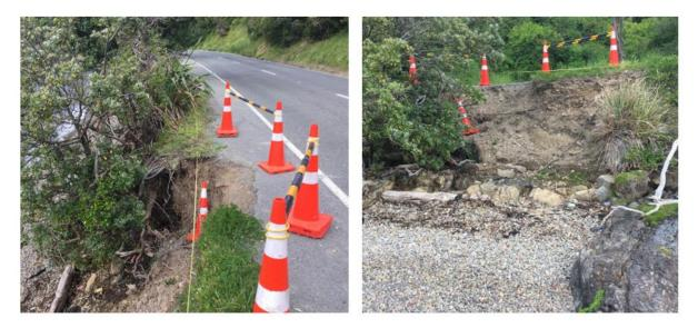
Photographs 3 and 4: Photographs of Landslip 2 along Shelly Bay Road. Photograph on left: View of the head scarp looking north. Photograph on right: View of the slip face from the base of the slope in the CMA. (Source: T+T, 2016)
