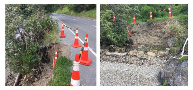
*Figure 2.4: Photographs of Landslip 2 along Shelly Bay Road. Photo on left: View of the head scarp looking north. Photo on right: View of the slip face from the base of the slope in the CMA.* (Source: T+T, 2016)
