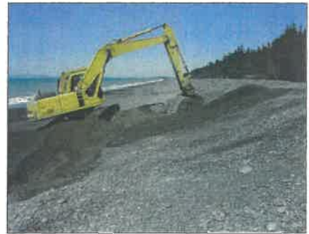
Repairing damage...a regular exercise at Amberley Beach over the years.
