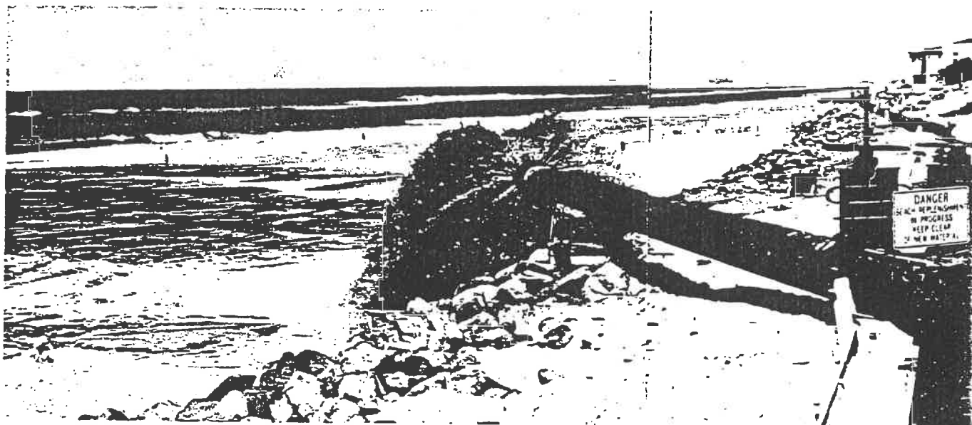
Beach and dune in the early stages of being rebuilt by dredging sand from the nearby estuary.
