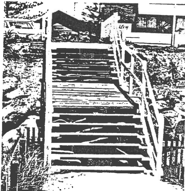
Steps providing access to and from the beach.
