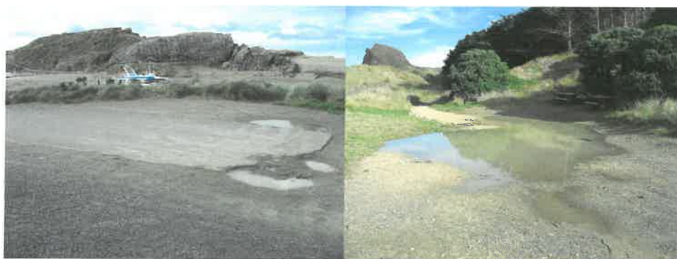
Photos 2 and 3. Current car-park at Castlepoint.
