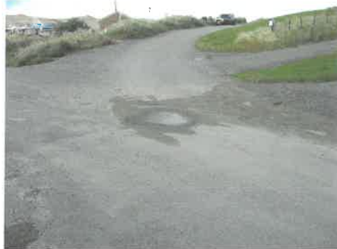
Photo 4. Current road access to Castlepoint car-park.
