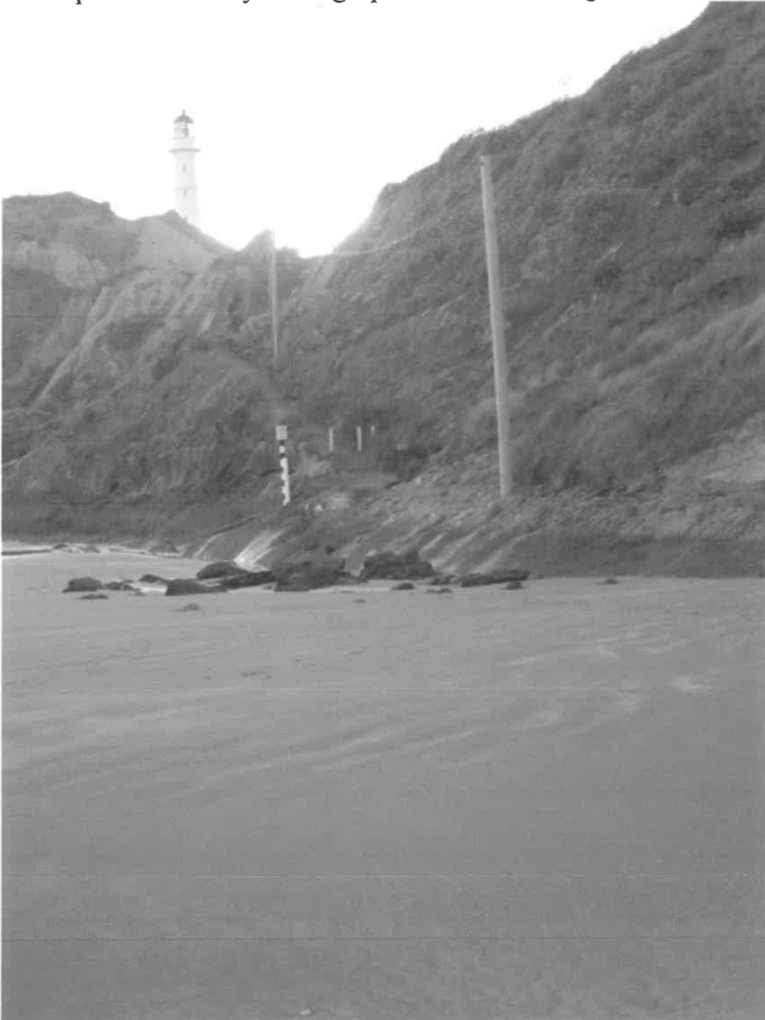
Figure 1: Photograph showing existing path and area where extension is to occur
