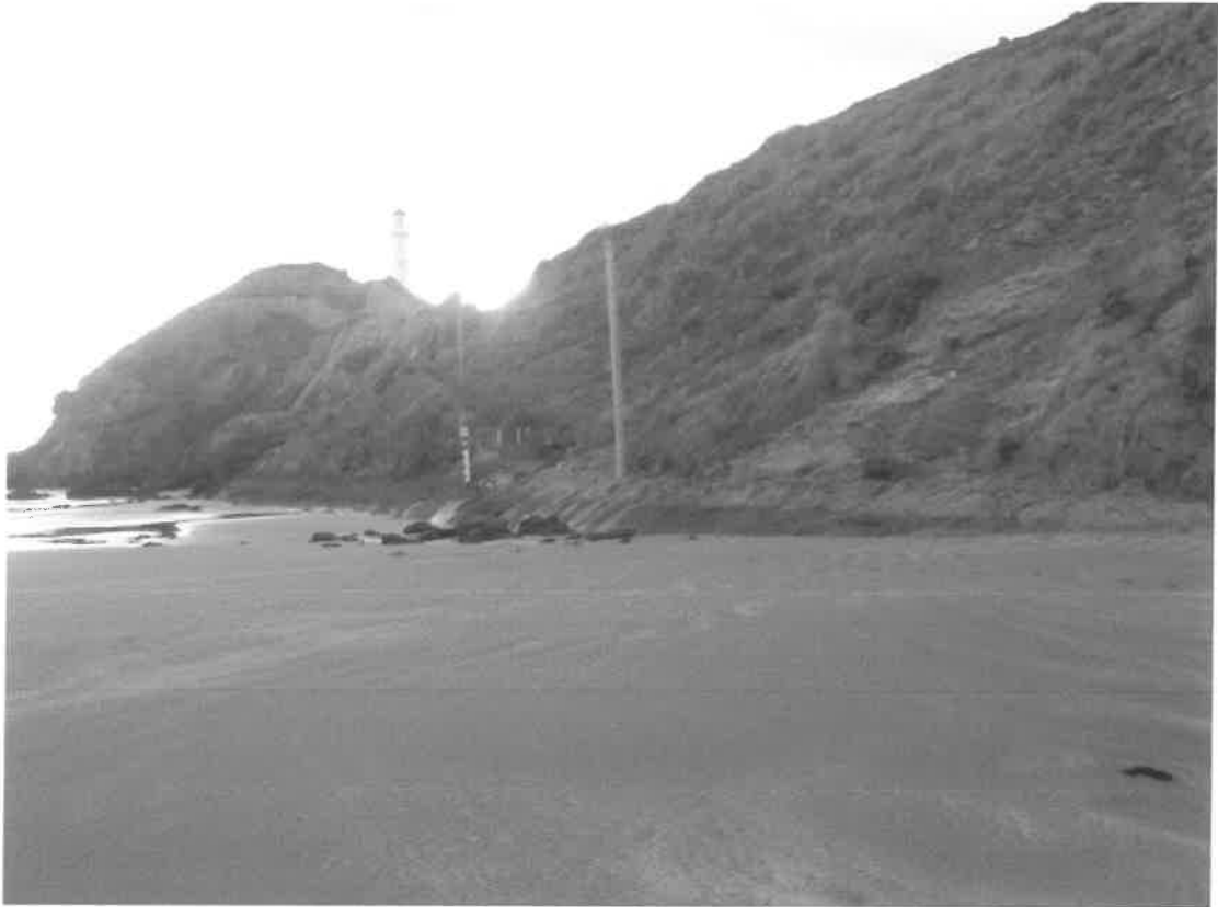
Figure 2: Photograph showing the existing path and extent of the proposed footpath extension
