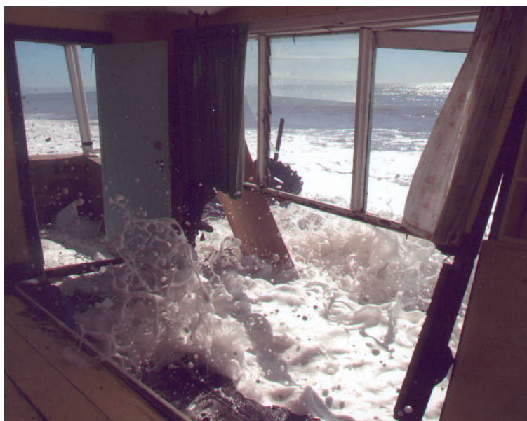
Figure A3.3: Damage caused to a coastal property at Haumoana (Hawke’s Bay) by waves overtopping the gravel barrier in the Easter storm of 3–4 April 2002, assisted by high perigean-spring tides. [Source: Hawkes Bay Regional Council].
