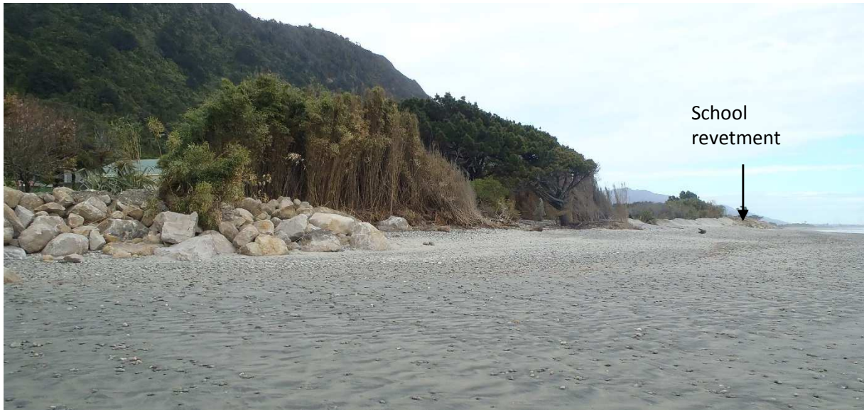
Figure 3-4: Unprotected section of coastline between Granity Stream revetment (centre left) and Granity school revetment (centre far-right). Photograph looking south along-beach towards school from Granity Stream (100 Torea St, Granity). [22 September 2015].
