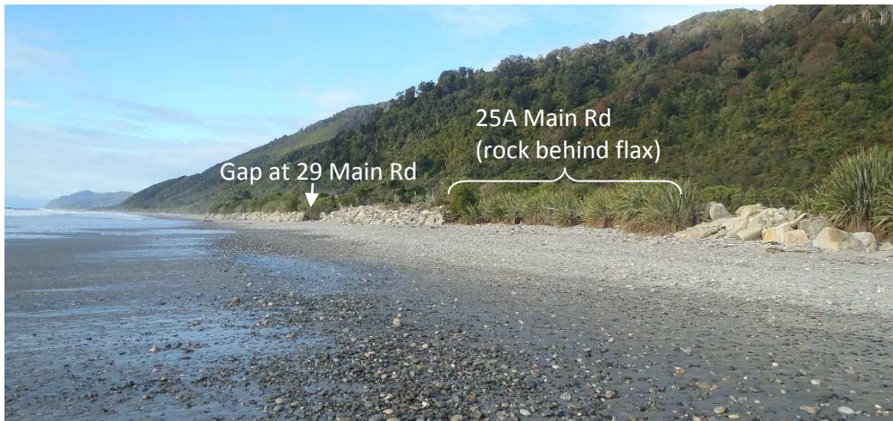
Figure 3-15: Intermittent defensive structure along beach at north Hector from 25A - 37 Main Rd. Gaps in beachfront revetment at 25A and 29 Main Rd. Note 25A has a small defensive line of rock behind beach front flaxes (annotation). Photograph looking north east from 25A Main Rd, Hector. [22 September 2015].
