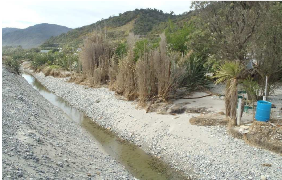
Figure 3-6: Overwash deposits and vegetation dieback behind mechanically cleared drain within private property. Berm approximately 1 m above beach level. Photograph looking northeast across diverted Bradley stream at approximately 155 Torea St, Granity. [22 September 2015].
