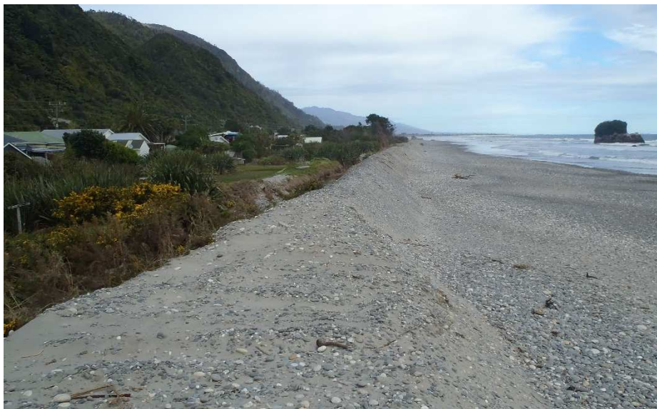
Figure 3-7: Narrow and low mechanically created gravel berm with diverted Bradley Stream and low-lying buffer space between houses at 155-165 Torea St. Photograph looking south towards Chair Rock (centre right) from 164 Torea St. [22 September 2015].
