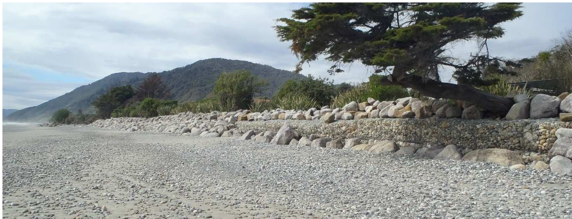
Figure 3-8: Coastal defence "Merrett's wall" along 11-14 Main Rd, Ngakawau. Privately funded structure built in 2007. Photograph looking north east along Ngakawau frontage from 11 Main Rd, Ngakawau. [22 September 2015].
