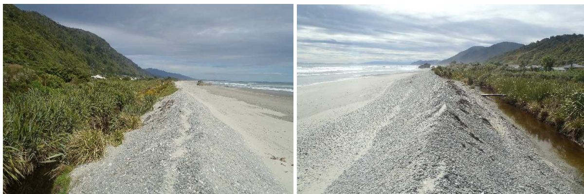
Figure 3-5: Example gravel barrier and wide vegetation/swamp buffer between beach and houses between Granity Stream to south (left, not visible) and Chair Rock (right, visible at centre). Photographs looking south (left) and north (right) at about 138 Torea St. [22 September 2015].
