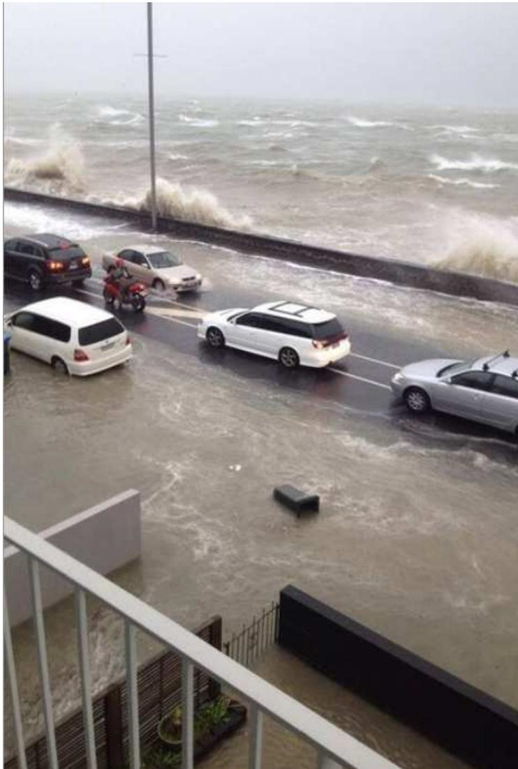
**Figure 3-1: Wave runup overtopping and flooding along Tamaki Drive, 17 April 2014.** Photo by Victoria Lowman obtained from New Zealand Herald on-line. The gale-force winds coincided exactly with high-tide, reducing the freeboard of the seawall, enabling waves to pump over enough water to inundate the road and adjacent low-lying coastal properties.
