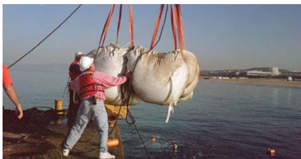
Figure 11 Placement of sandbags at Pratte's
