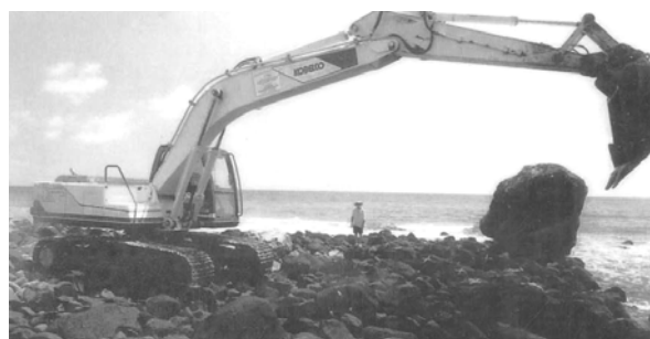
Figure 2 Excavator moving boulders at low tide (Source: Greg Redgard)
