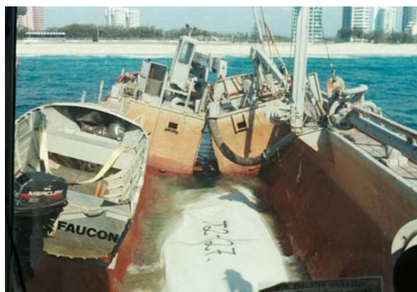
Figure 8 Placing containers from a split hull hopper dredge at Narrowneck
