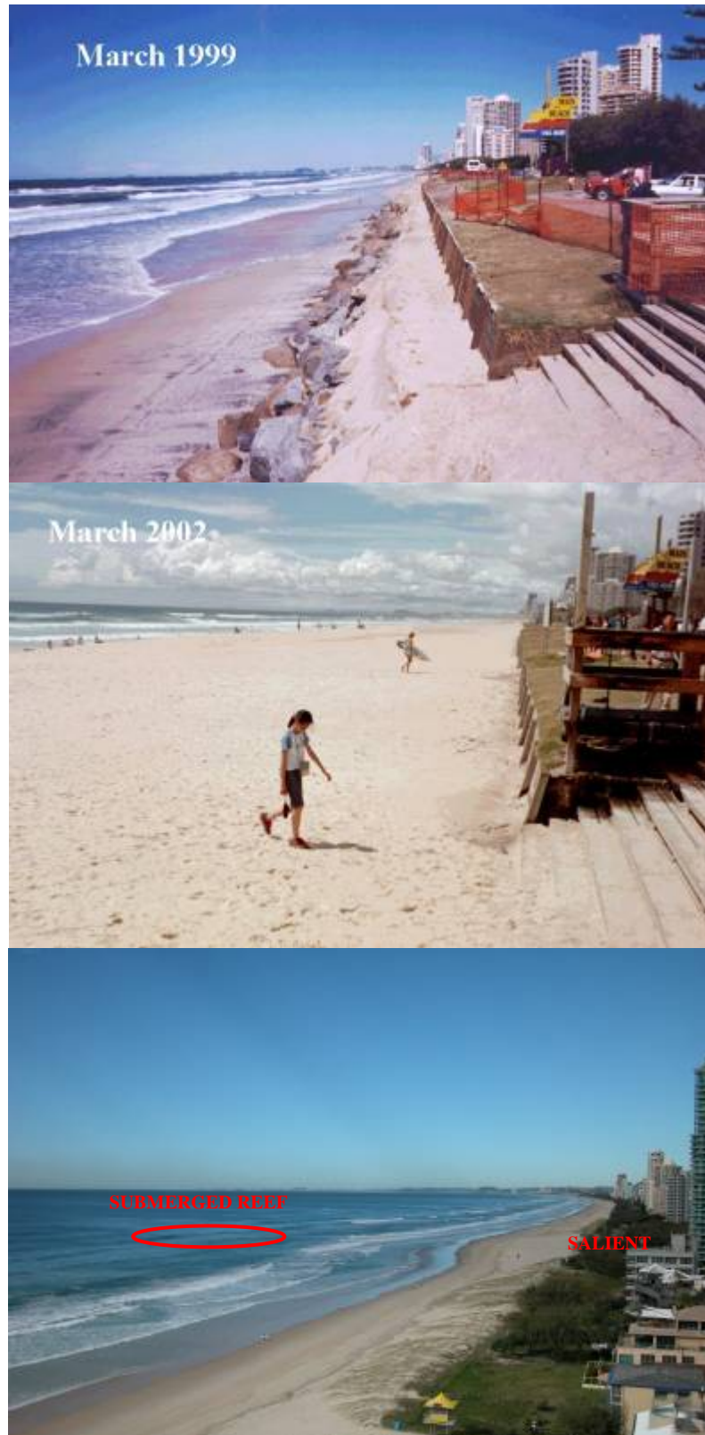
Figure 4. Coastal protection with the Narrowneck submerged reef. Top to Bottom: Before reef construction (construction commenced in August 1999); After reef construction; The view looking south showing the wide salient in the lee of the reef.
