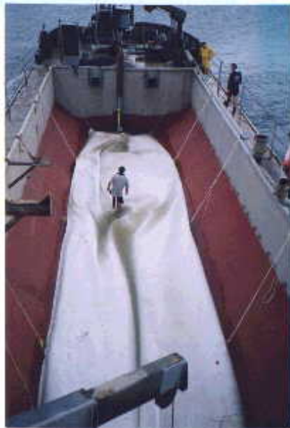
SPLIT HULL HOPPER DREDGE FILLING SANDBAG
