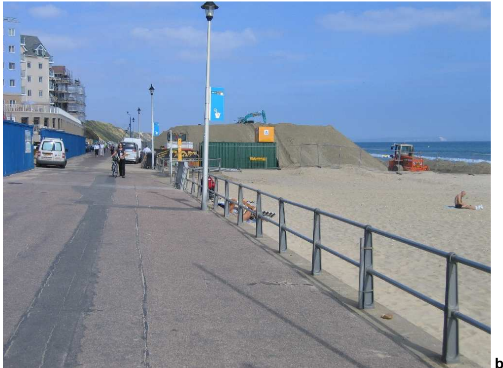
Figure 4.9. Schematic overview of the work area required for construction of the Orewa Multipurpose Reefs (A). The lower photo shows the typical beach/land construction set-up, with the sand stockpile, containers with 550 hp pumping system and construction fencing to keep out the public during construction (Boscombe, England).
