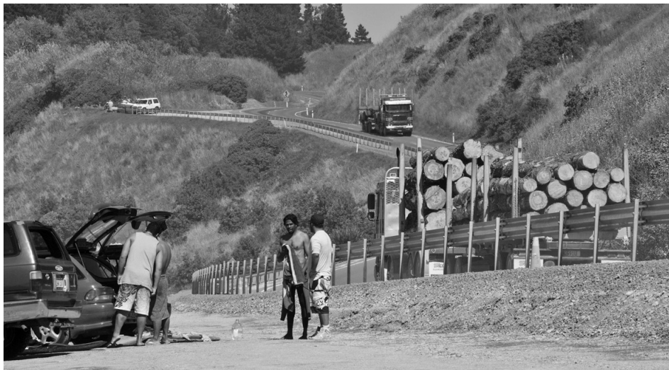
PROTECTED SPECIES: Surfers now park their vehicles behind the “safety” of steel crash barriers after traditional access to the surf at Makorori was blocked by recent road works.
