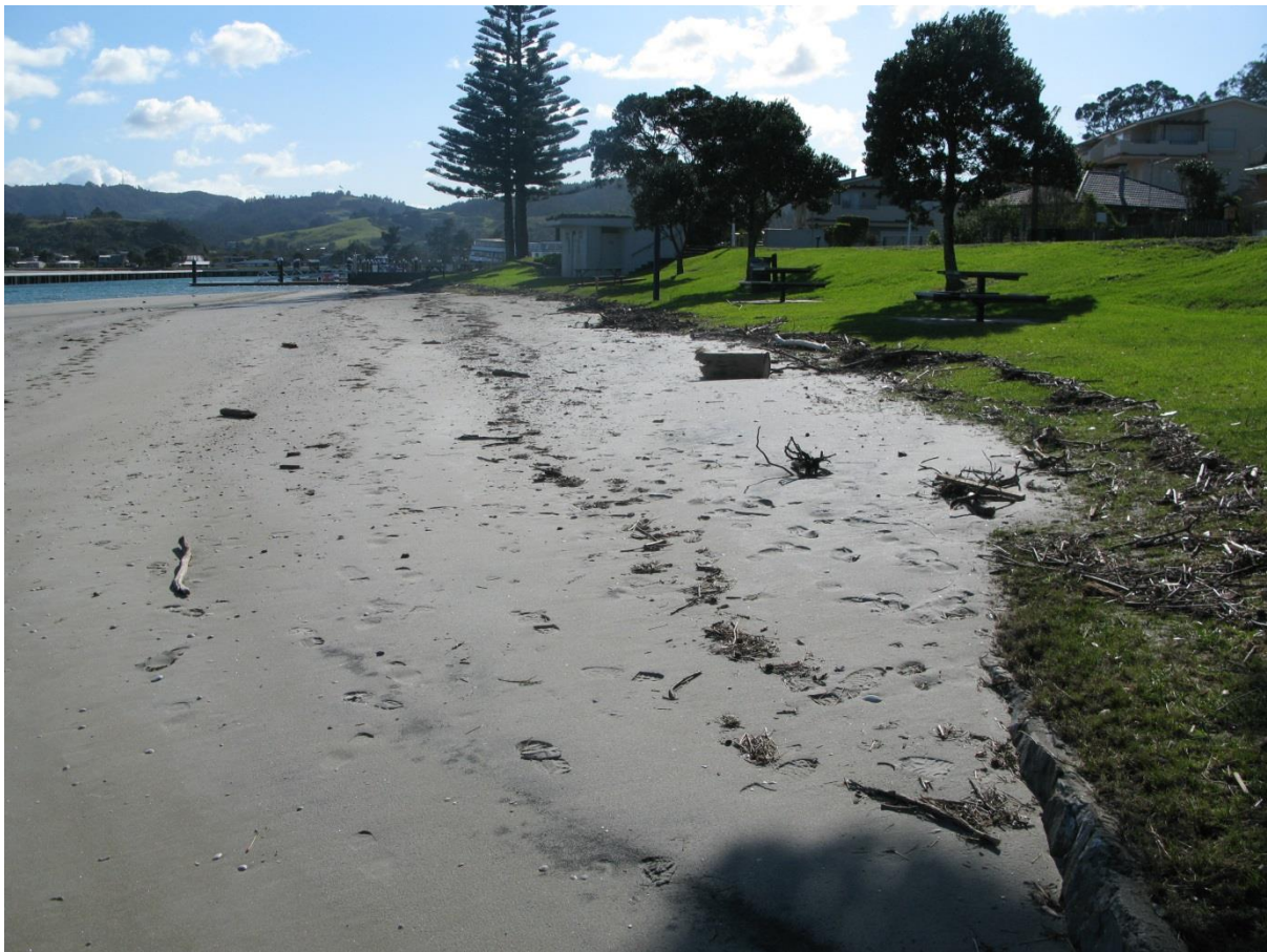
Figure 15: Esplanade beach, Tairua Harbour. Recent beach nourishment has significantly raised the beach level and improved the amenity value of the area.
