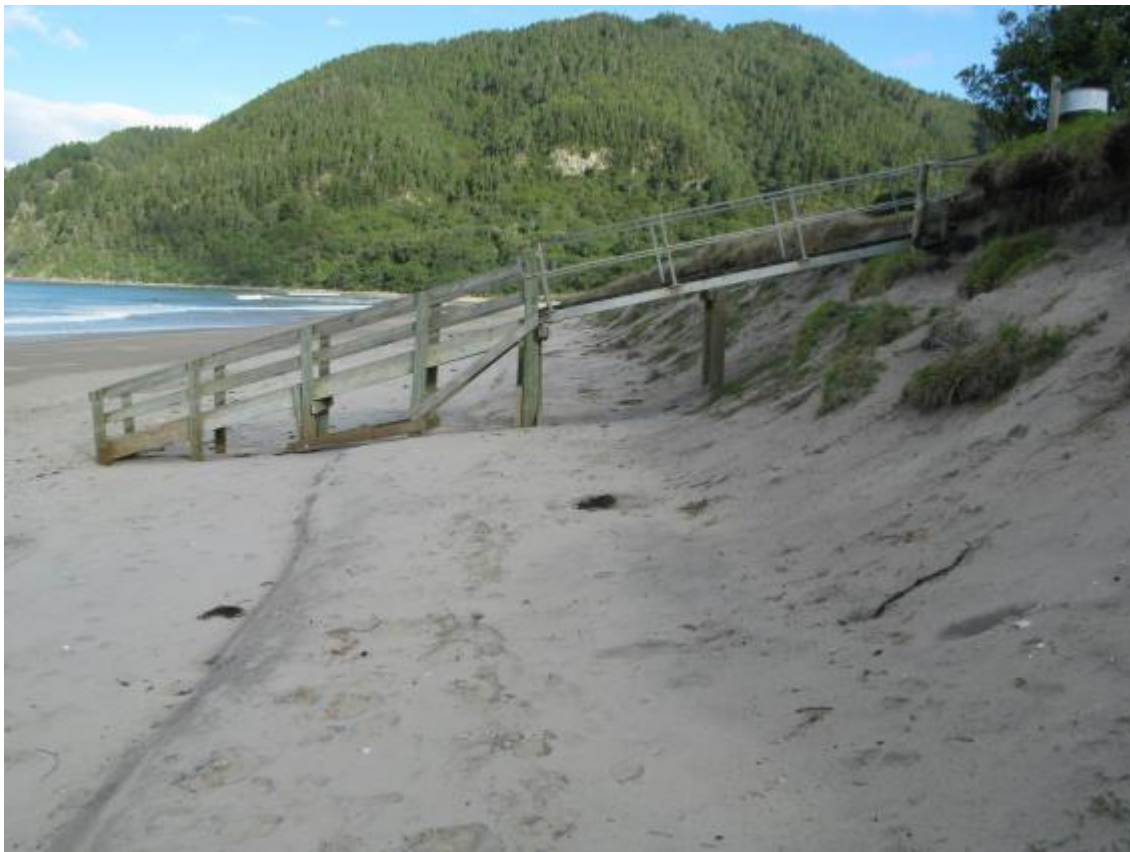
Figure 7: View of beach accessway 9 located towards the southern end of Pauanui Beach in 2012. In 2009, the seaward edge of the dune toe was approximately 8m further seaward. These changes are typical of the natural shoreline fluctuations which occur over time and the erosion will naturally recover.
