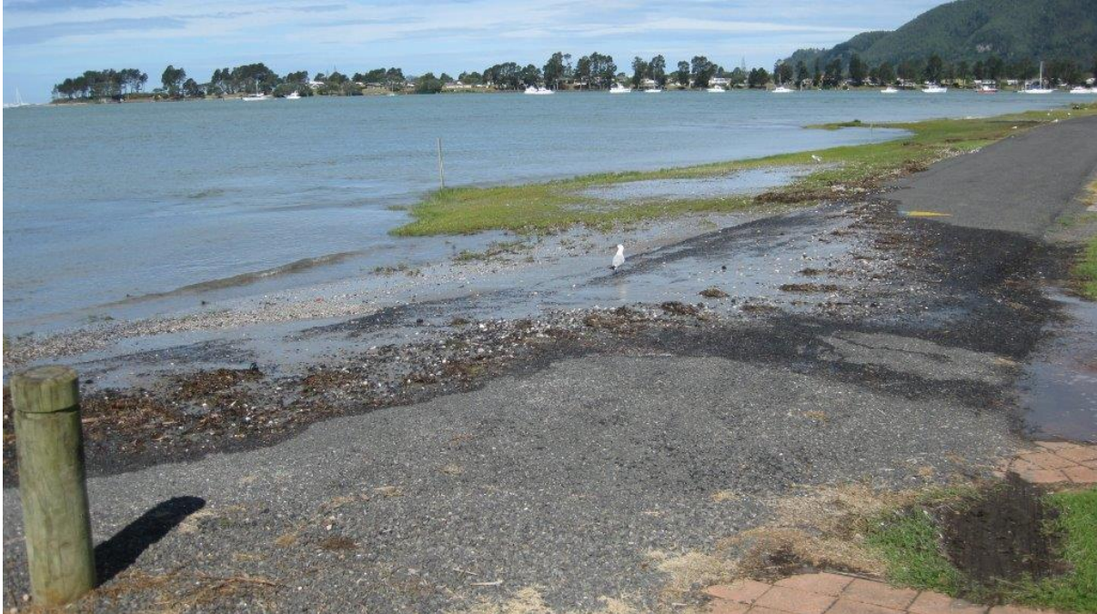
Figure 21: Recent (16 March 2015) flooding of Bayview Road.
