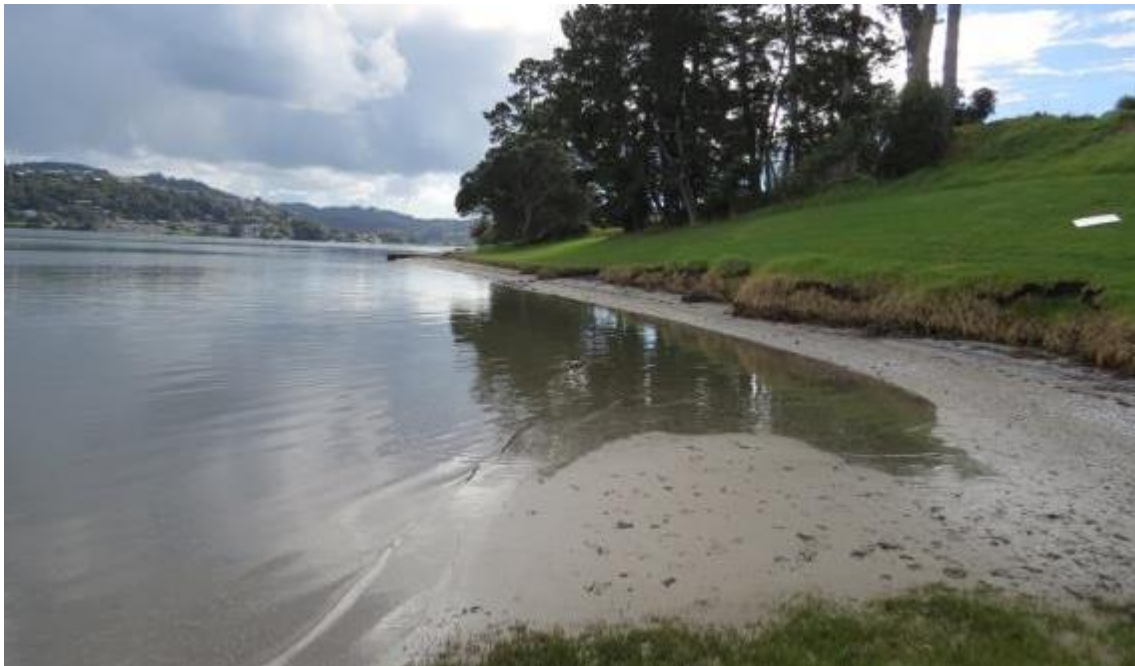
Figure 25: Area of past beach nourishment between Pleasant Point and Ajax Head. The sloping grassed reserve was constructed using dredged material from construction of the Waterways access channel in the 1990s. Monitoring indicates that the placed sediment performed well and much of the placed sediment is still present, even though slow erosion is occurring.
