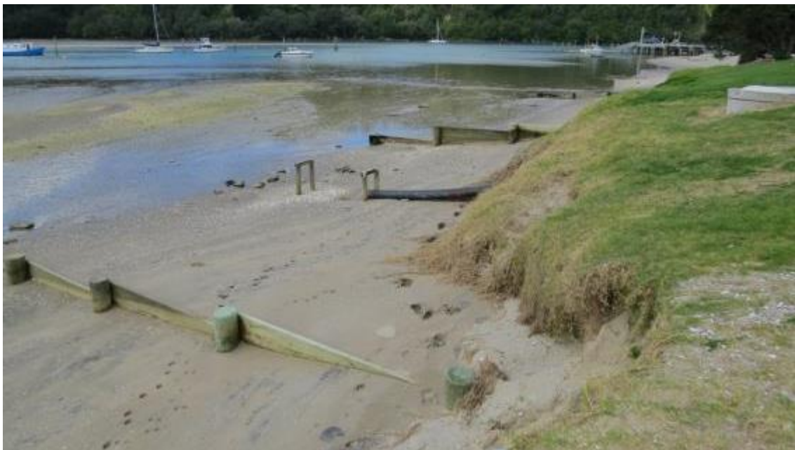
Figure 28: The shoreline adjacent to Beach Road, between Bond and Rutherford Roads. Erosion in this area can be severe at times and may threaten Beach Road in the future.
