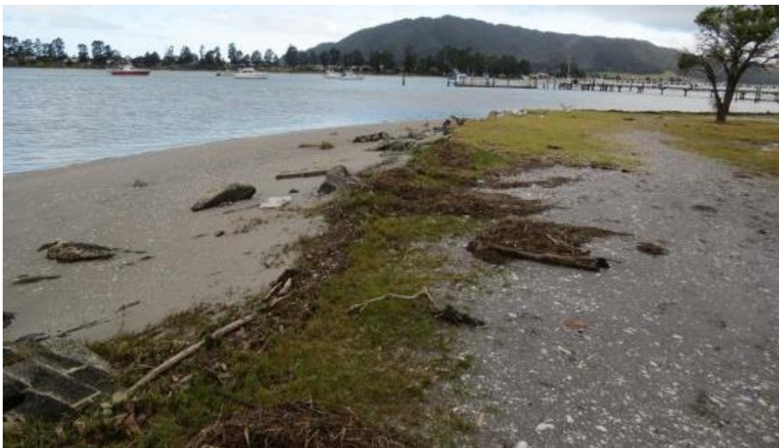
Figure 20: Rocks and remains of structures near Mary Beach. Removal of these materials would improve public safety and amenity, as well as the general appearance of the area. It is likely that erosion in this area can be successfully managed using beach nourishment as required.
