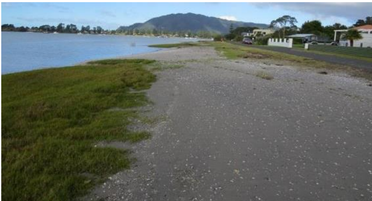
Figure 18: Shoreline at northern end of Bay View Terrace showing successful beach nourishment. Note that the beach is however gradually being covered by saltwater paspalum.
