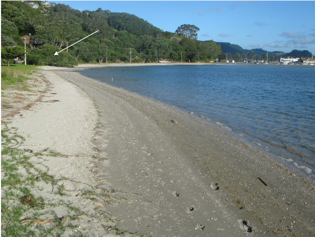
Figure 16: Paku Bay showing enhancement of the natural and amenity values by recent beach nourishment. The large pohutukawa tree near the centre of the beach (arrowed) is culturally significant and the nourishment has also enhanced protection of this tree which had been undermined by erosion and collapsed across the beach.
