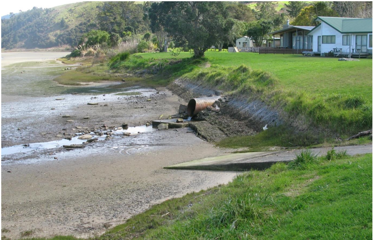
Figure 31: Stormwater outlets in Otahu Estuary near Kotuku Road
