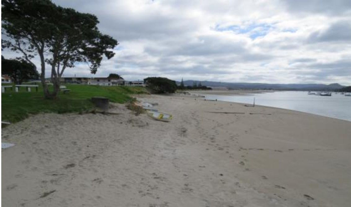
Figure 27: The shoreline immediately upstream from the Whangamata Wharf. The beach is presently in an accreted condition with the groynes buried. This relates to a natural pulse of sand passing through the area and the groynes have not played a significant role.
