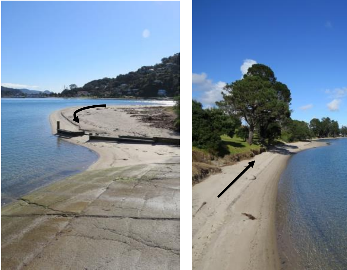
Figure 23: Sediment accumulation on eastern side of Pauanui Wharf boat ramp (left), and eroding beaches to the west (right), where sediment should be placed. Arrows indicate dominant natural direction of sediment transport.
