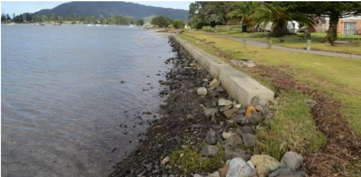
Figure 19: Block seawall south of Bay View Terrace
