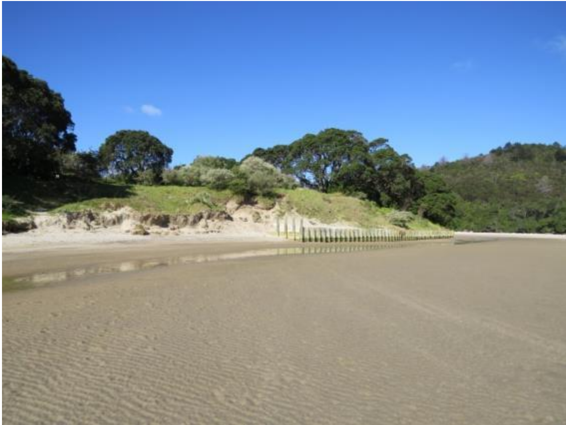
Figure 29: Wooden wall protecting the estuary shoreline of Otahu Point historic reserve at the entrance to Otahu estuary.
