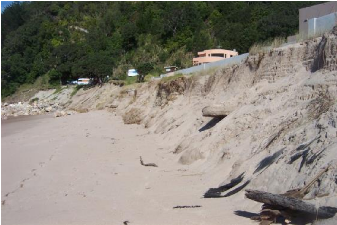
Figure 8: The south end of Tairua Ocean Beach following severe erosion in 2003.
