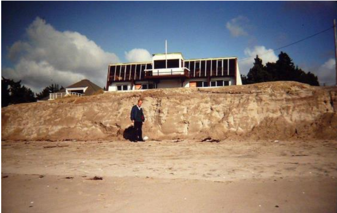
Figure 4: View of south end of Esplanade Drive near the surf lifesaving club showing severe dune erosion which occurred during a storm in July 1978. (Photo provided by Mr. Ray Madden).
