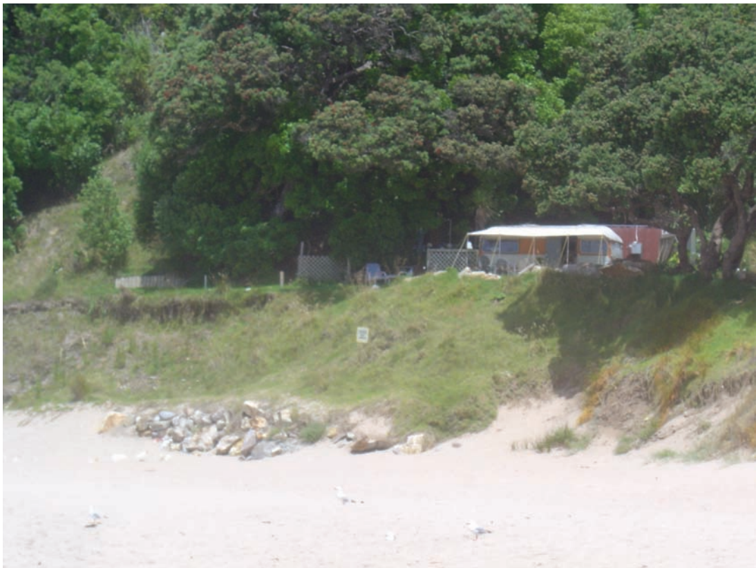
Figure 4.7 South end of Tairua's Ocean Beach showing rocks placed in an attempt to halt erosion
