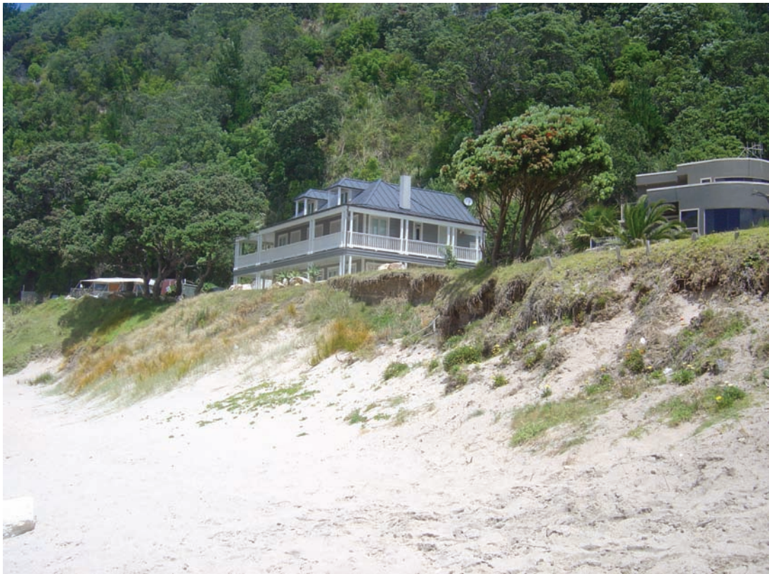
Figure 4.6 South end of Tairua's Ocean Beach showing houses close to beach and within hazard zone
