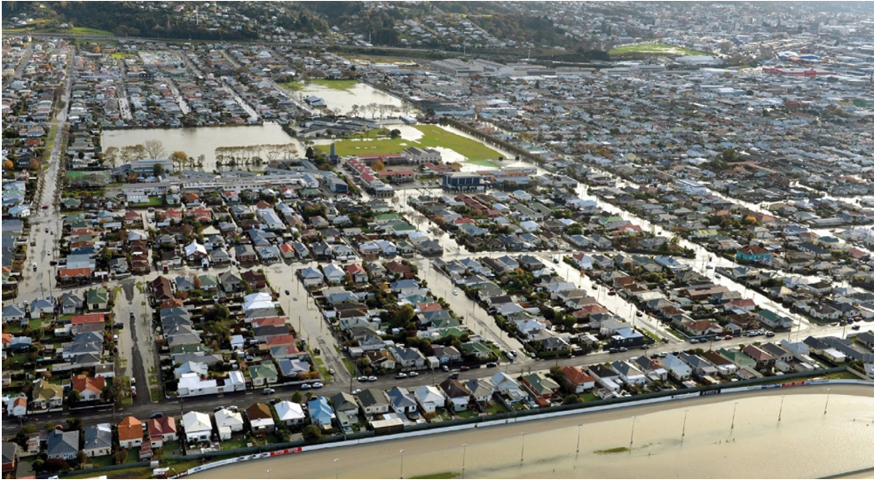
Figure 8: Flooding of South Dunedin June 2015 (source: Otago Daily Times ).
