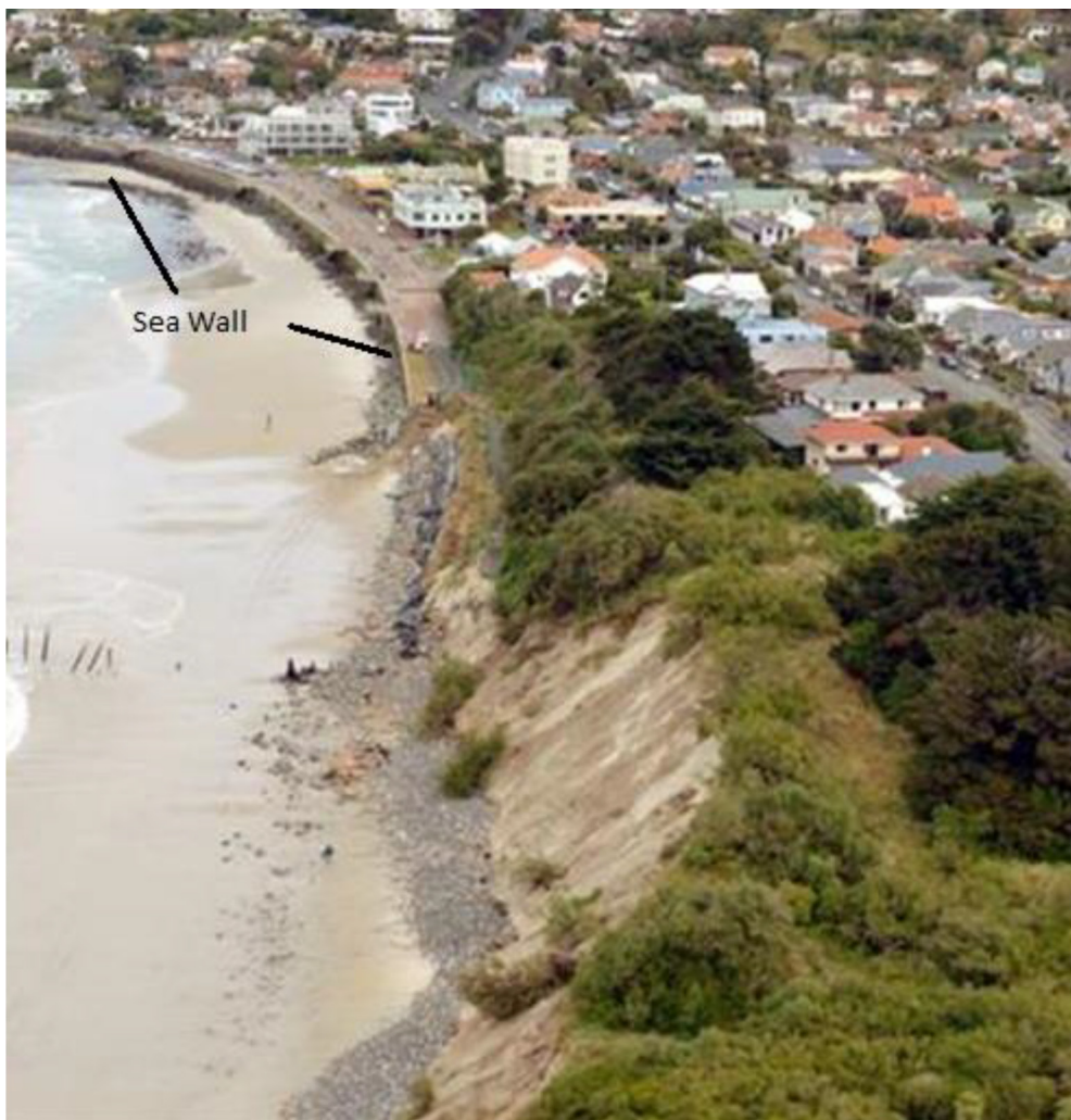
Figure 2: The St Clair sea wall and erosion beyond the eastern end of the wall (foreground). Poles which are remnants of past efforts to stop erosion here are visible in the surf zone (middle left) (Otago Daily Times).
