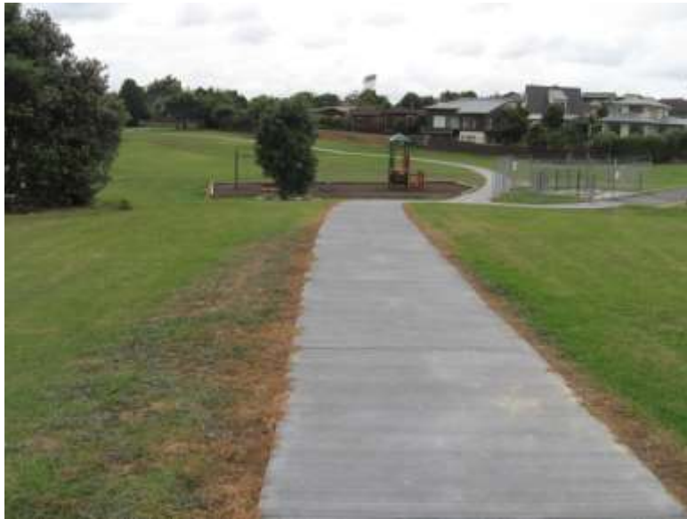
2m wide concrete walkway on grass
