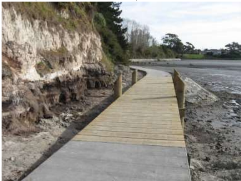
2m wide timber coastal boardwalk
