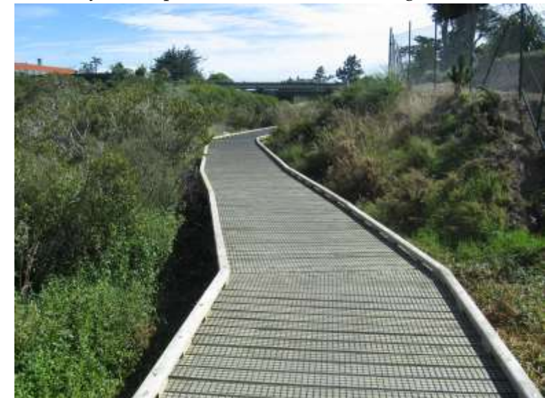
2m wide timber boardwalk with kerbs
