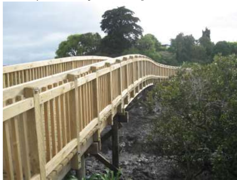
Coastal boardwalk and bridge with barriers
