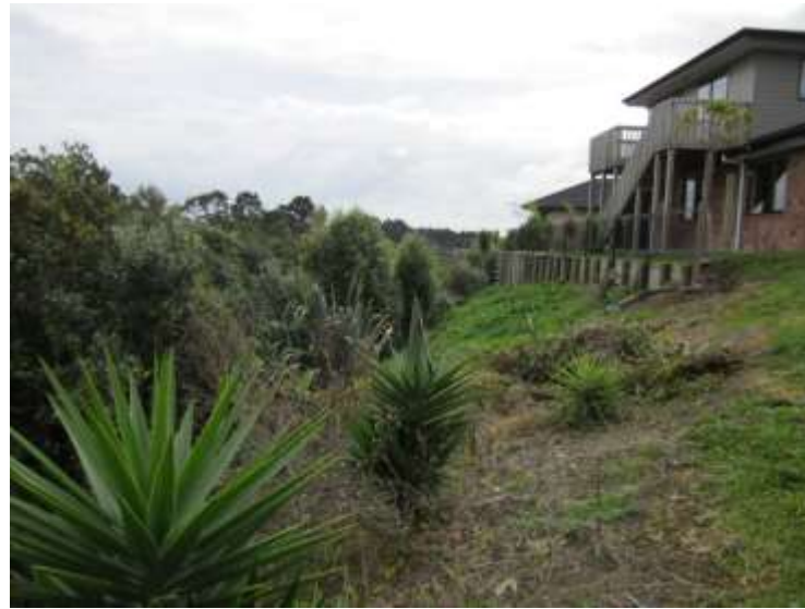
A3 – Form walkway below private retaining wall
