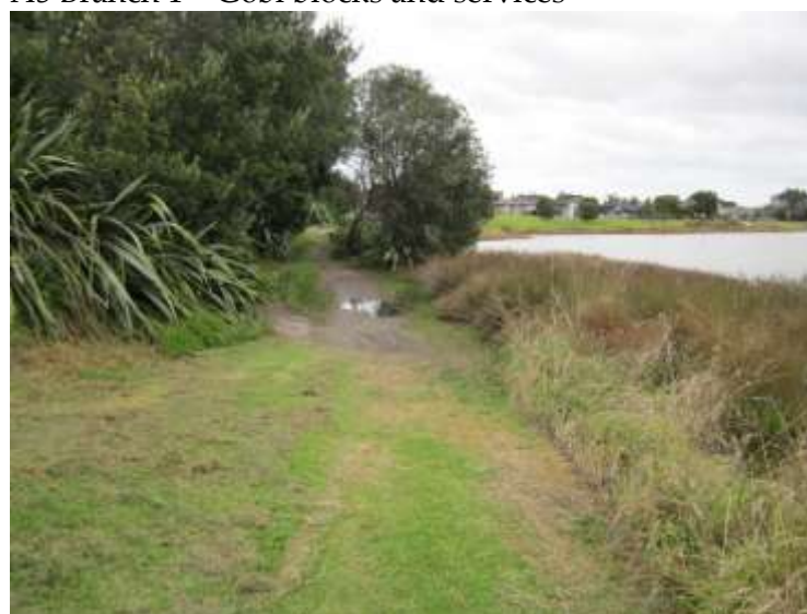
A7 – Fill low wet area and form walkway
