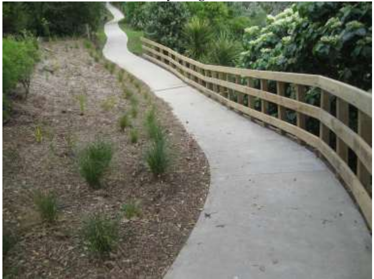
Walkway with downhill retaining wall and barrier
