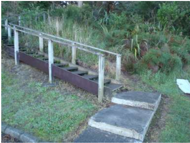
C1 – Remove concrete and staircase
