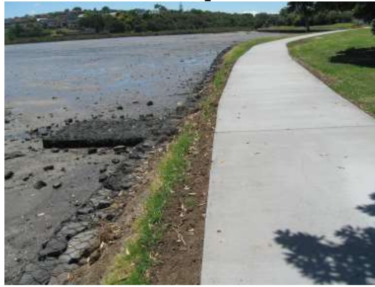
2m wide concrete walkway on coast
