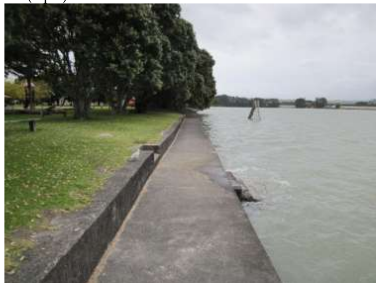
A10 (Op 2) – Existing seawall
