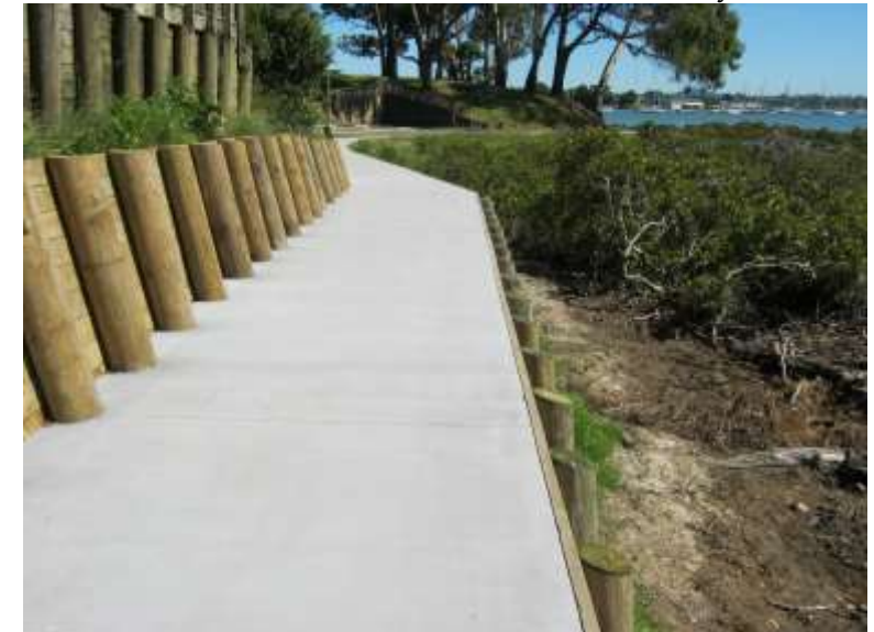
Walkway with uphill and downhill retaining wall
