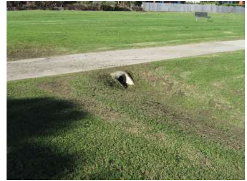
200mm diameter culvert under concrete walkway
