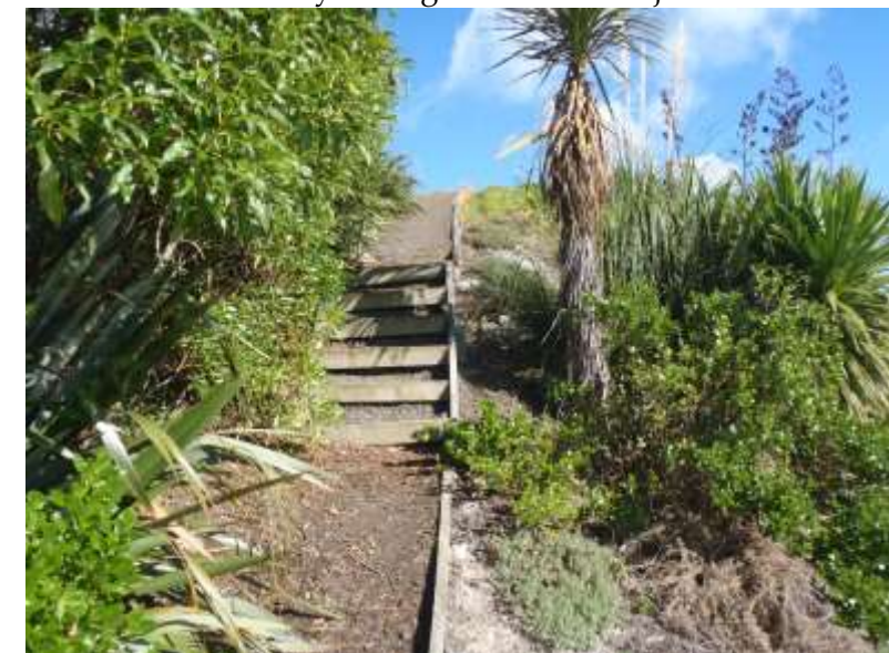
C21 Branch – Upgrade aggregate path and steps to concrete wall
