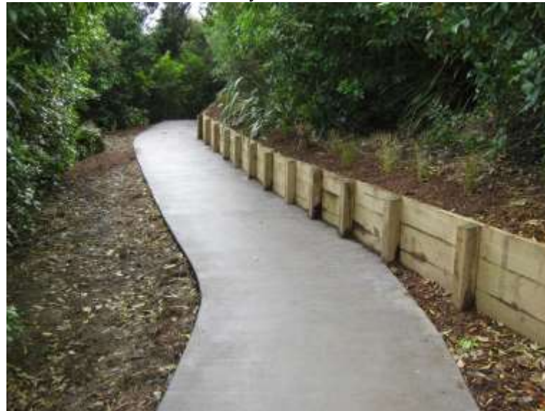
Walkway with low uphill retaining wall
