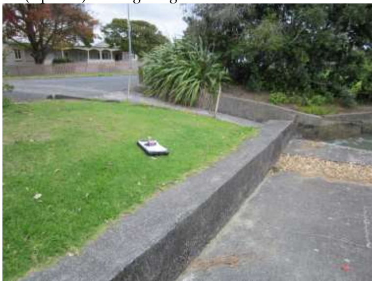
A9 (Op 2) – Boat ramp and seawall, benching required
