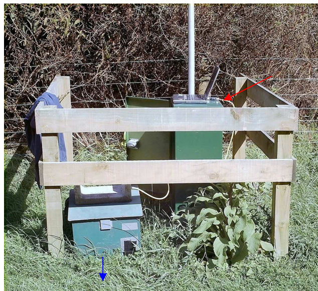
Figure 4.12 Site 1, showing the telemetered groundwater site that is monitored by GW (see red arrow). The baroTROLL used for this study was also located in this housing. This site also contains a set of TDR probes. The probes are buried at set depths towards the foreground of the photograph (see blue arrow).
