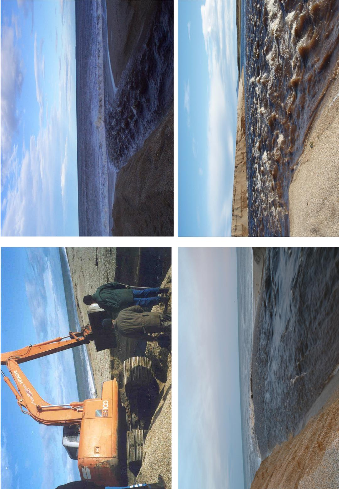
**Figure 3.1: typical opening of Waituna Lagoon (photos from 2002 and 2010). The top left and bottom right photos show the breach channel development within 6 hours of opening. The bottom right photo shows the established breach channel.**
