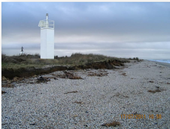
Figure 19: Bushy Point lighthouse foreshore facing east towards Waituna Lagoon, July 2011 showing the gravel accumulation on the upper beach.
