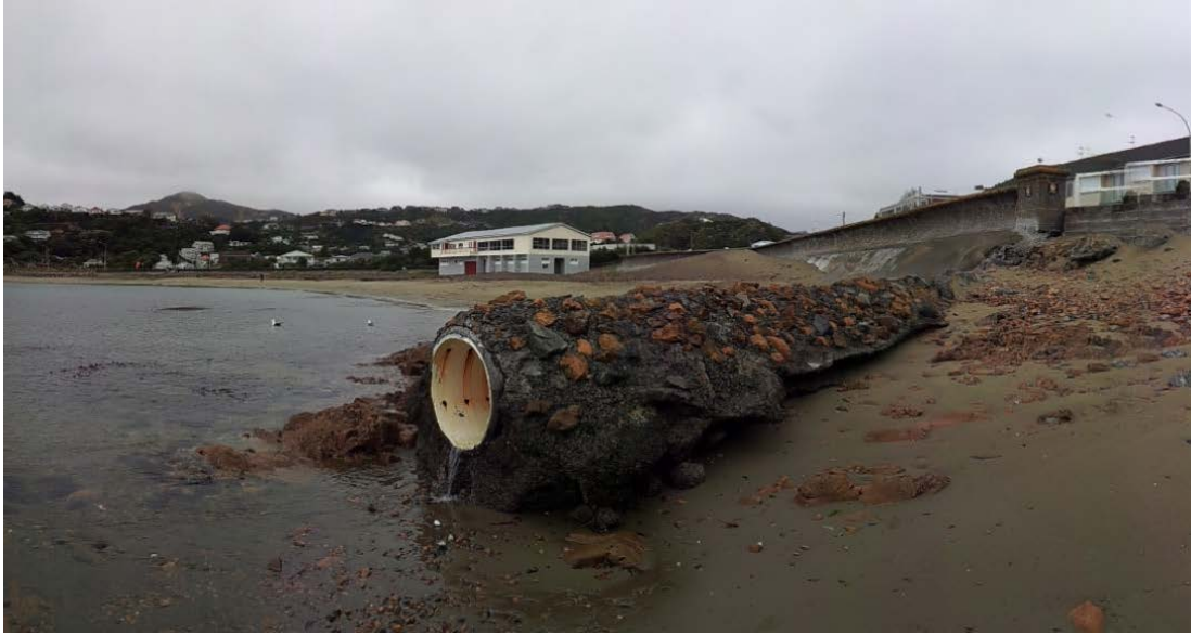
A-3 Grouted rock and concrete outfall on eastern side of bay
