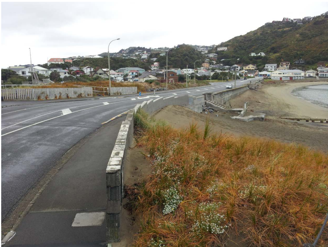
A-6 Wind-blown sand accumulating against seawall and detached dune system evident across road in Shorlanad Park
