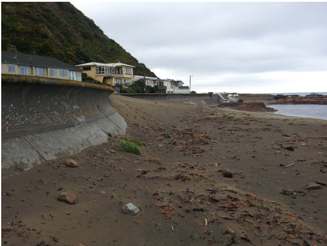
A-2 Wind-blown sand accumulating against the existing seawall on eastern side of bay
