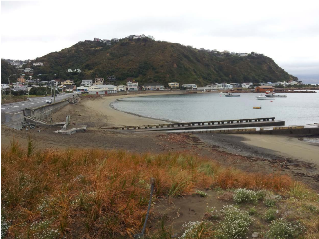
A-1 Island Bay overview showing crescentic beach planform backed by straight seawall
