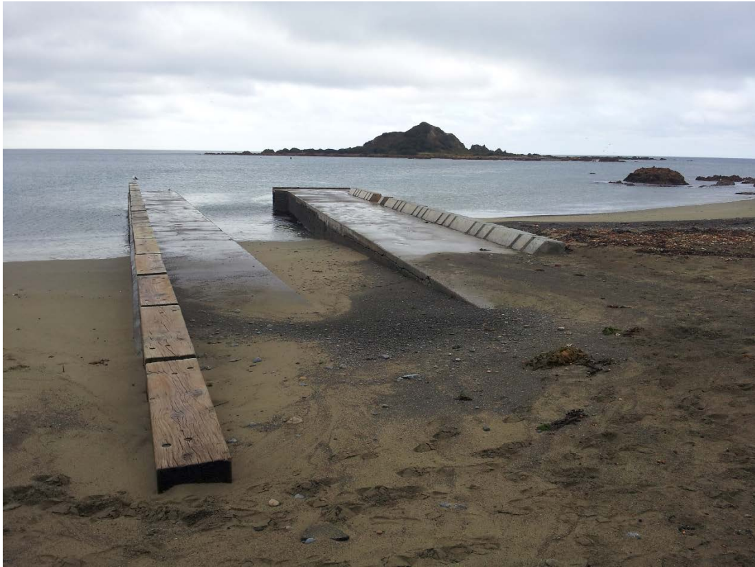
A-5 Stormwater outfalls at southwestern end of bay
