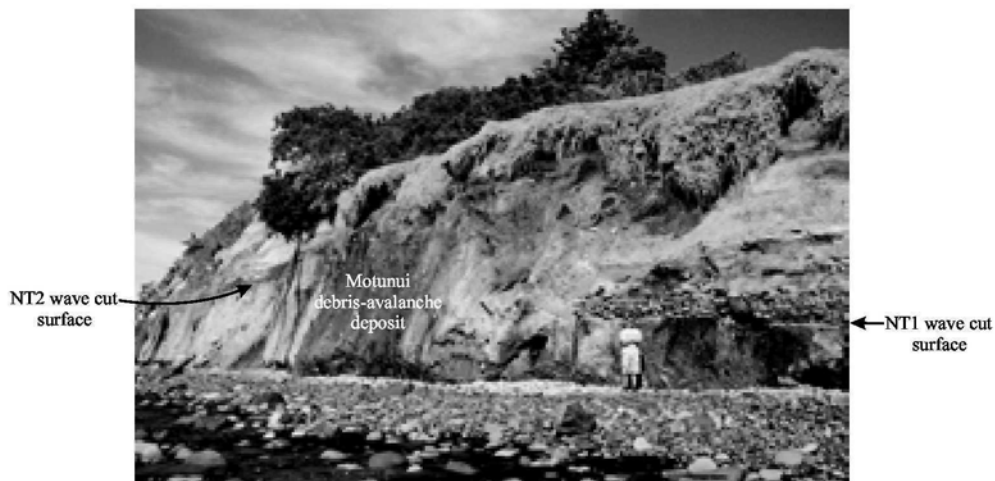
Fig. 19 Three wave cut surfaces truncating Motunui Formation are exposed c. 0.1 km east of the coastal end of Turangi Road. These are: the present day beach platform, NT1 (lower) and NT2 (upper) surfaces. The strandline of the NT1 surface can be observed just to the left of the person.
