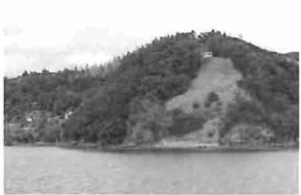
V762 Vegetation Removal
