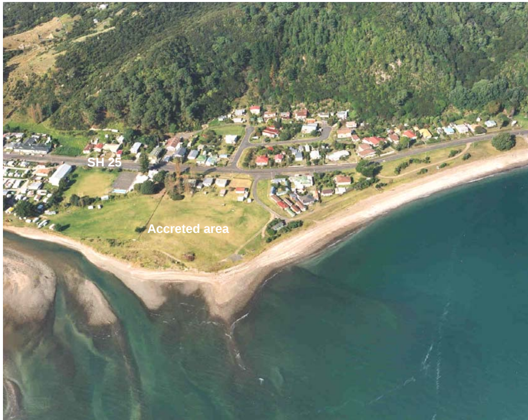
Figure 4-4: Tapu Stream deltaic fan in 1994, showing infilled embayment (accreted area). The maximum width of the accreted area is about 120 m. Wharf Road (referred to in text) is the branch road running seaward from SH25. In the early 1900's, this road led to a wharf located on the southern side edge of the embayment shown in Figure 4-3. The area south of Wharf Road (behind the trams and houses shown) has also accreted, by about 20 m over the last 60-70 years. (Photo 49348, Maps Ltd, Tauranga, flown 1/6/94).
