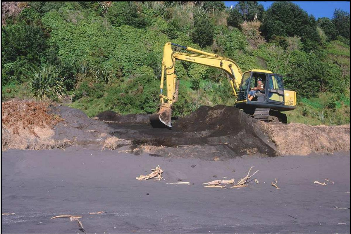
*Figure 6: Sand was taken from near high water mark and moved landward. Where practical, consolidated layers of clay or other compacted fill were placed towards the back of the dune.*
