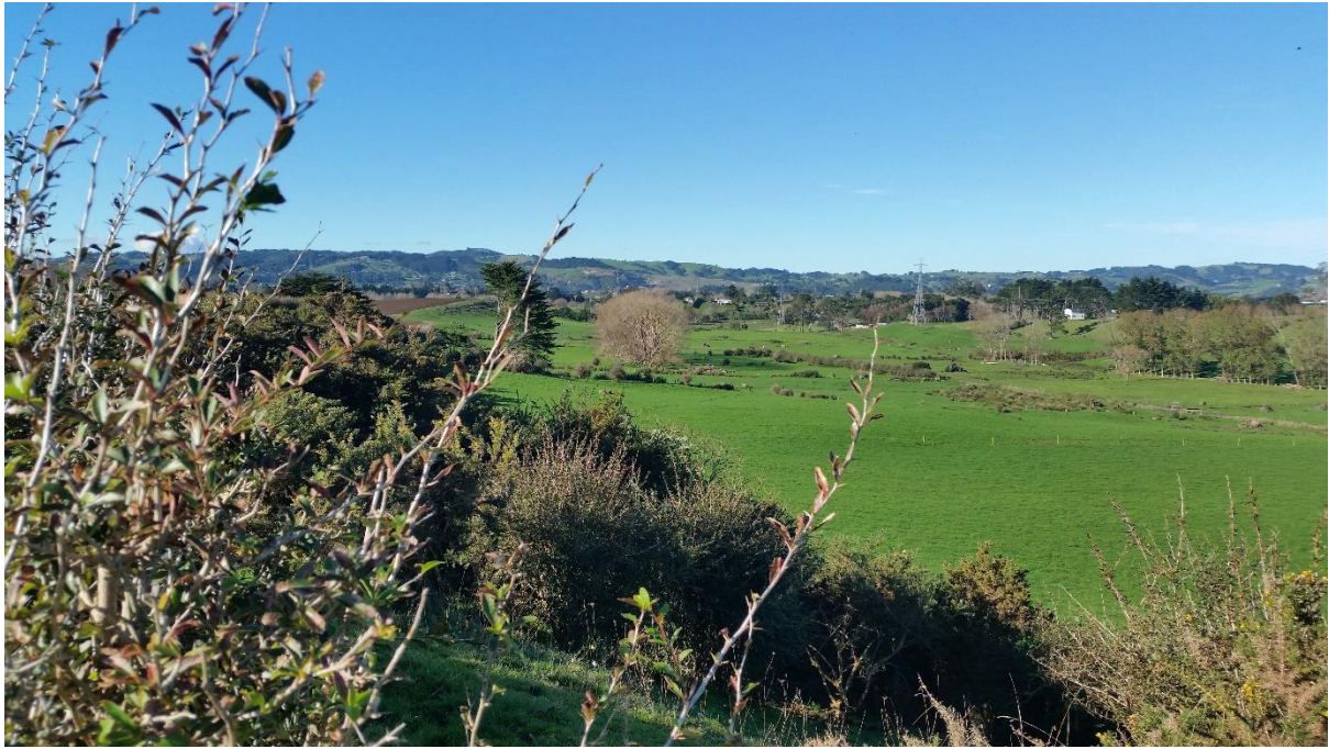
Photo 2: Looking east near the intersection of Cheriton Road and Burt Road. The slope in the foreground is mapped as being underlain by SAVF ash (note the steep contour) and has an assessed high slope instability potential. The flat land in the distance is mapped as being Puketoka Formation but is low lying and may have portions of Holocene Alluvium.
