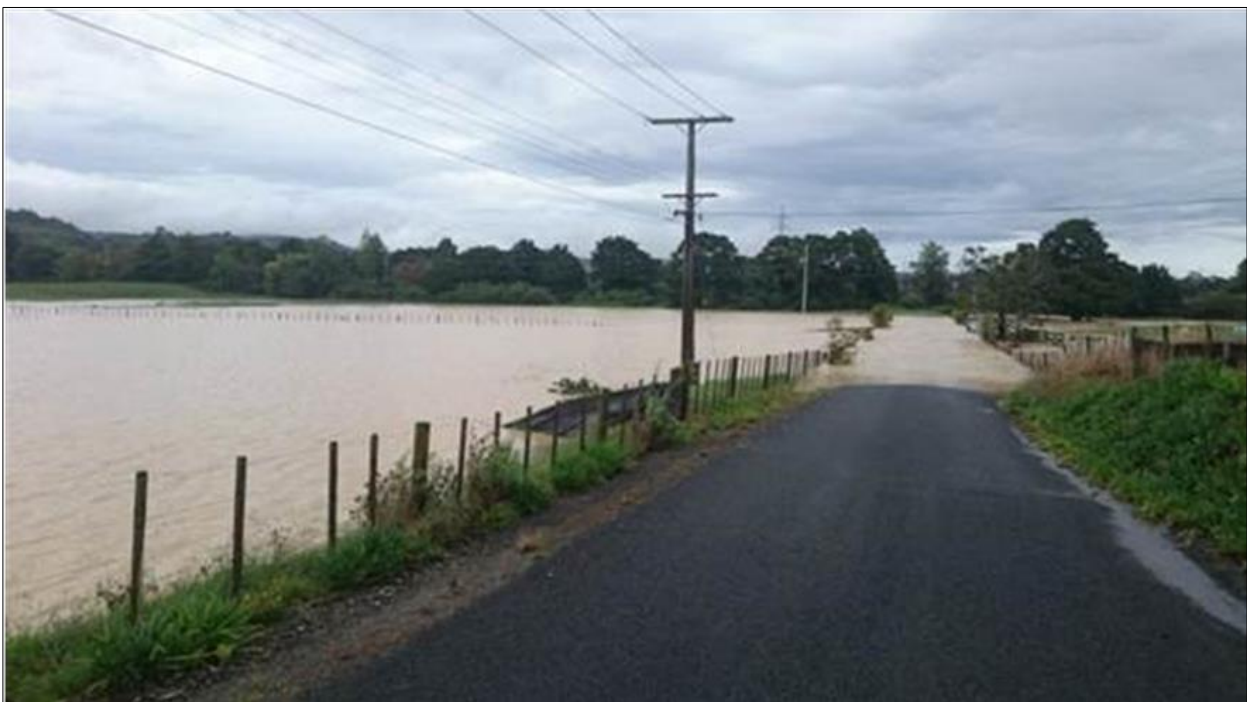
Figure 16 Flooding in the Hingaia Stream catchment 2017
