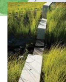
L: Grass bunding to along edge of grass slope to restrict flow of stormwater and damage to planting on lower slopes
