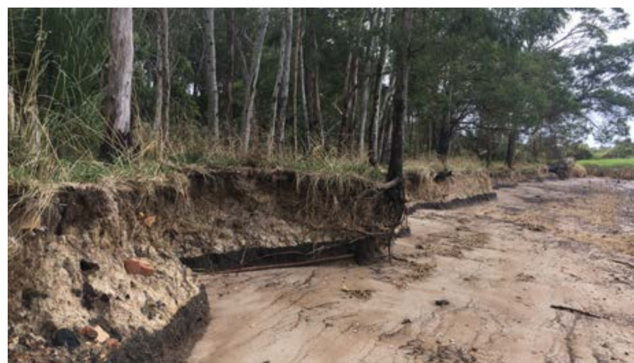
Coastal erosion at the southern end of the park at the historic brickworks site
