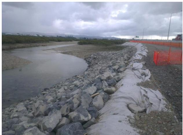
**Figure 130: Examples of geotextile filter layer beneath a rock revetment and use of rip rap**
