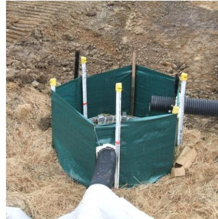
**Figure 97: Good use of a silt fence installed to protect a new stormwater catchpit where impounded water will not create a flooding hazard**
