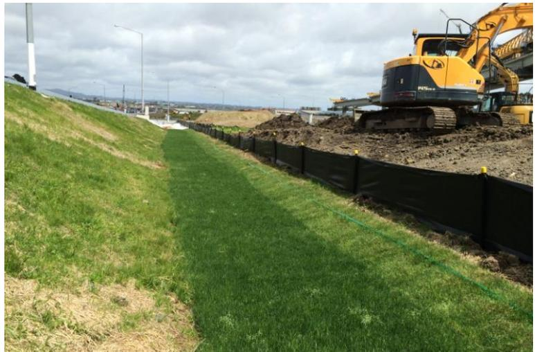
**Figure 52: Turf used to provide instant stabilisation of the swale allowing for early commissioning of the device**
