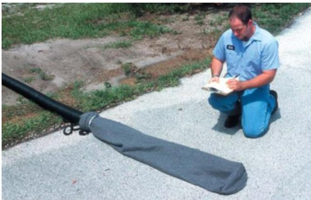
Figure 105: Dewatering bag and pipe sock
