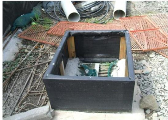
**Figure 96: Stormwater inlet protection silt fence within a construction yard**
