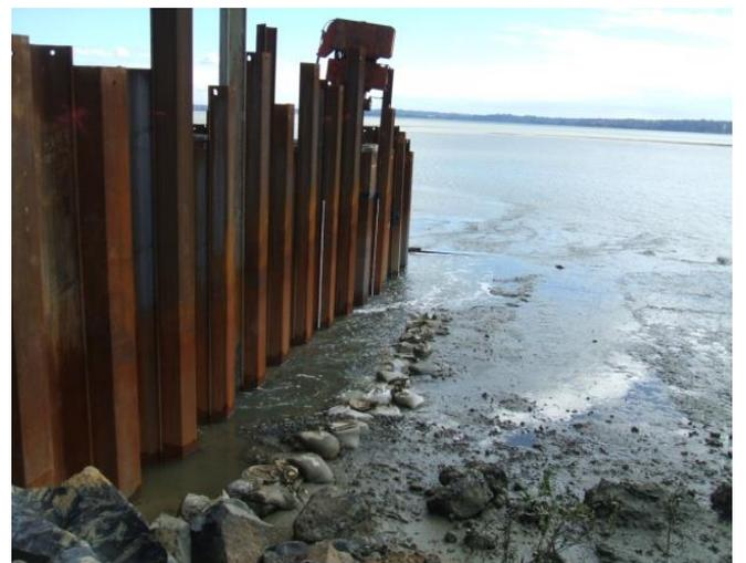
**Figure 132: Water draining from a sheet pile coffer dam**
