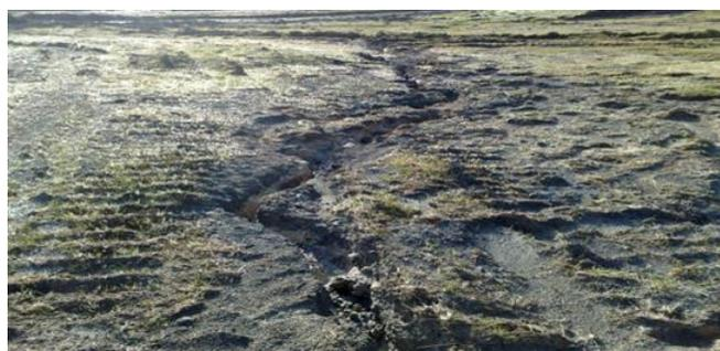
**Figure 46: Loss of topsoil and grass seed after heavy rain event. Will require stabilisation and reapplication**
