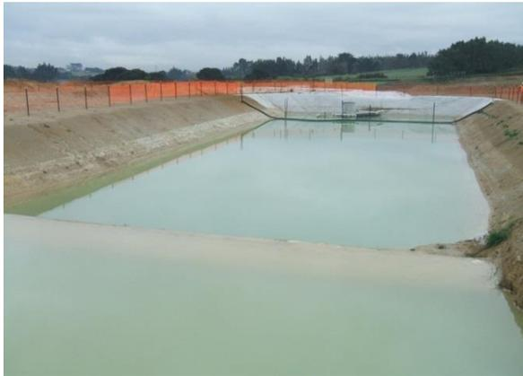
**Figure 75: Level spreader across the full width of the pond**
