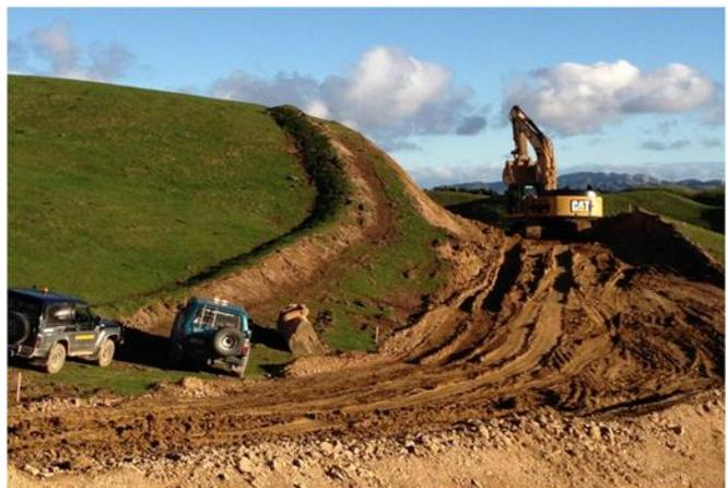
Figure 14: Clean water diversion used to isolate upper clean water flows from the works area
