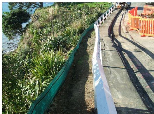
**Figure 79: Silt fence installed on edge of works**
