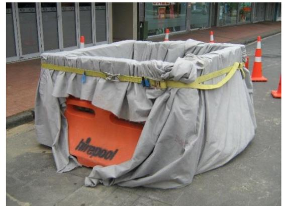
Figure 106: Example of a mobile 'turkey nest' used for dewatering
