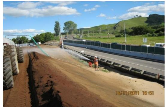
**Figure 127: Dust suppression using soil binders/polymers**
