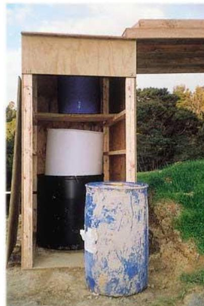
**Figure 99: rainfall activated flocculant treatment device**
