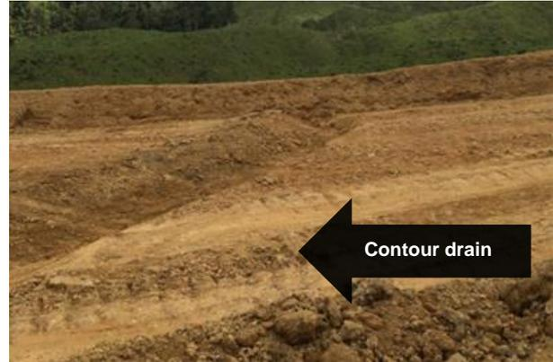
Figure 21: Contour drain
