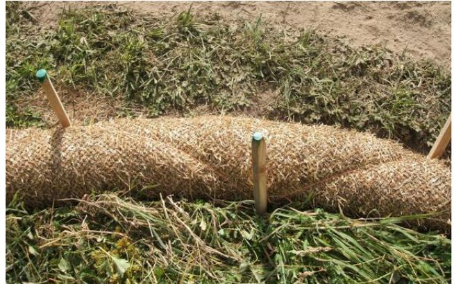
**Figure 93: Straw sock secured in place using stakes and bale twine; note the stakes are placed every 600 mm**
