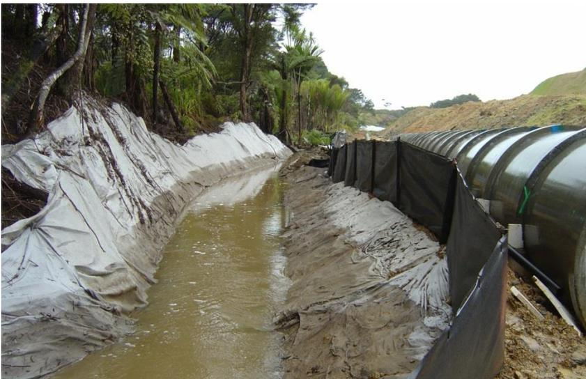
**Figure 111: Temporary stream diversion to allow for the installation of a new culvert**
