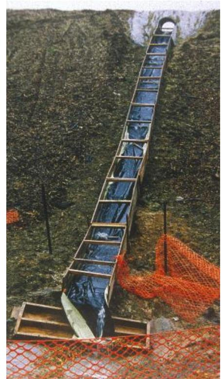
**Figure 31: Wooden flume lined with impervious material**
