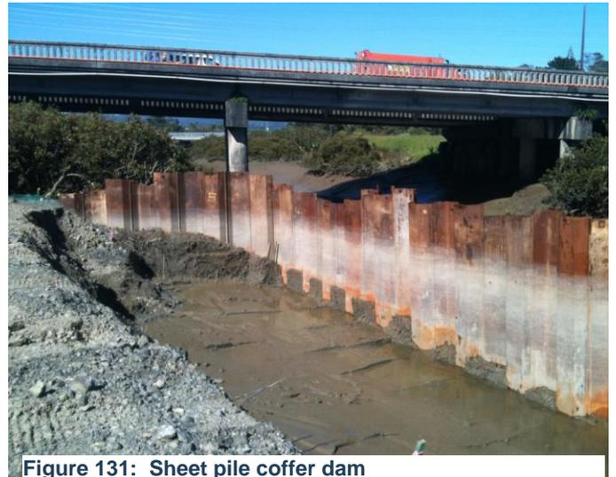
**Figure 131: Sheet pile coffer dam**
