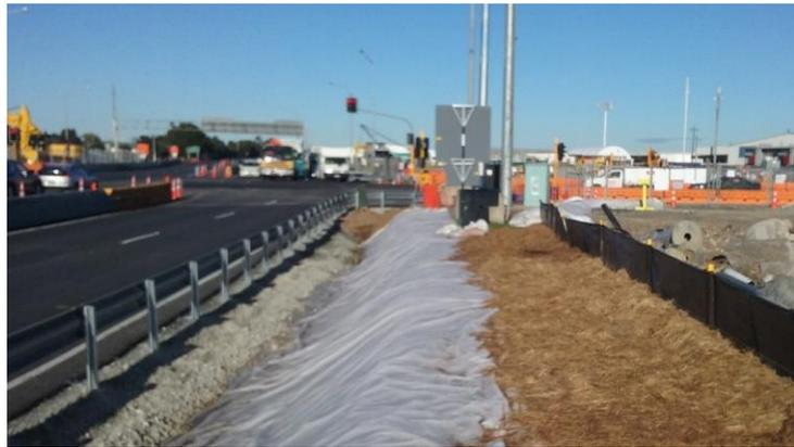
**Figure 108: Progressive stabilisation in limited space**
