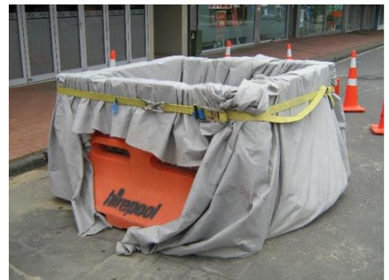
Figure 106: Example of a mobile 'turkey nest' used for dewatering
