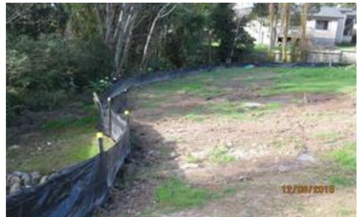
Figure 107: Silt fence
