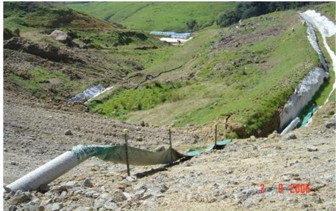
**Figure 11: Flume installed to protect steep slope**
