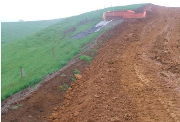
**Figure 123: Decanting earth bund and diversion bund installed during a farm track construction**
