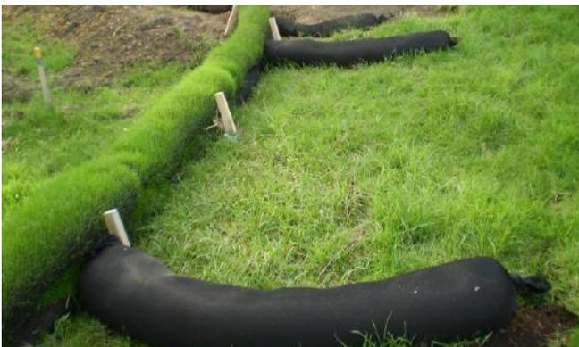
Figure 90: Compost silt socks with returns installed
