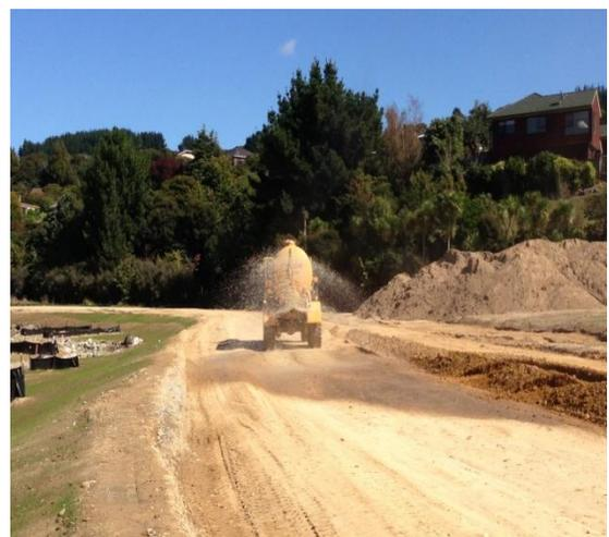
**Figure 125: Dust suppression using a water cart**
