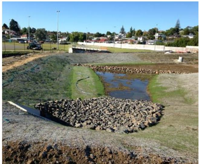
**Figure 49: Recently applied hydroseed on a stormwater wetland**
