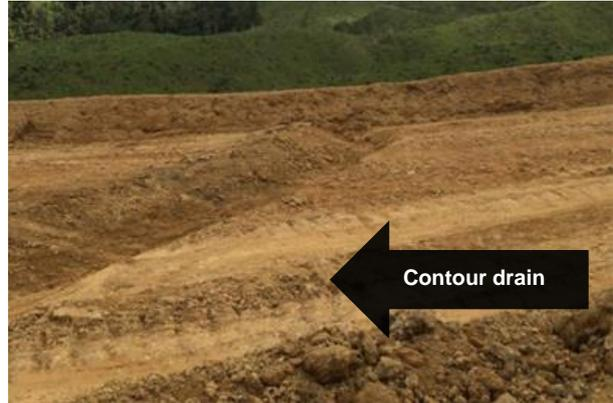
Figure 21: Contour drain
