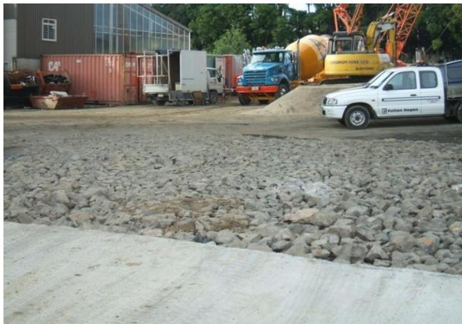
**Figure 34: Stabilised entranceway**
