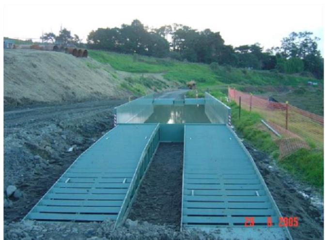
**Figure 37: Example of a shaker ramp**
