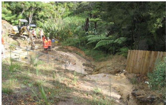
**Figure 12: Sediment discharge as a result of not protecting the watercourse**
