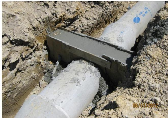
**Figure 70: Example of an anti-seep collar**
