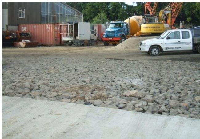
Figure 34: Stabilised entranceway
