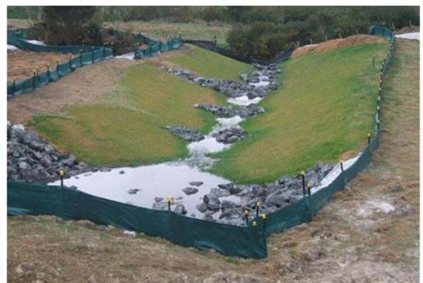
Figure 25: Check dams installed in series to act as a permanent water velocity control measure
