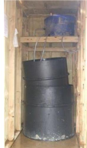
**Figure 103: Flocculation shed**
