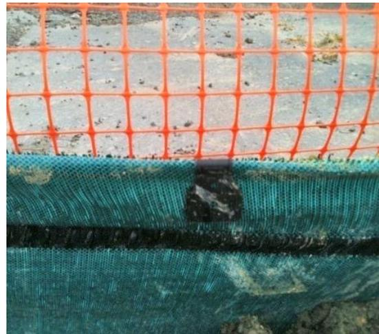
**Figure 85:** Use of silt fence clips
