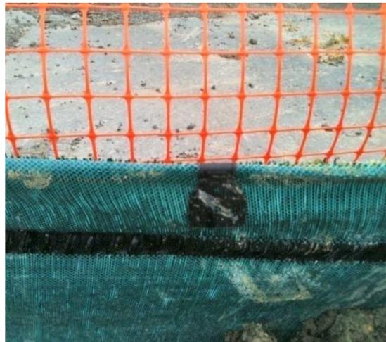
**Figure 85: Use of silt fence clips**
