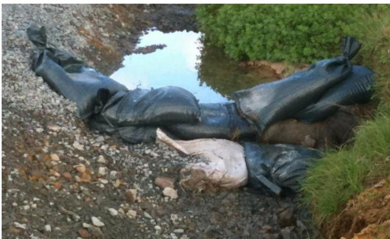
Figure 27: Check dams installed with a spillway to direct flows over the centre of the structure. Sand bags placed directly below spillway provide a protective apron below the dam
