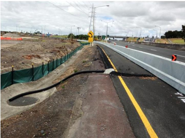
**Figure 17: Hotmix bund diverting the motorway runoff to the catchpit**
