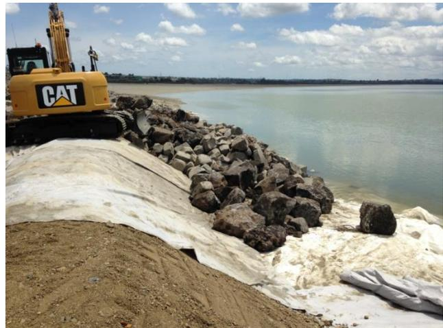
**Figure 133: Use of geotextiles and coastal protection rock**
