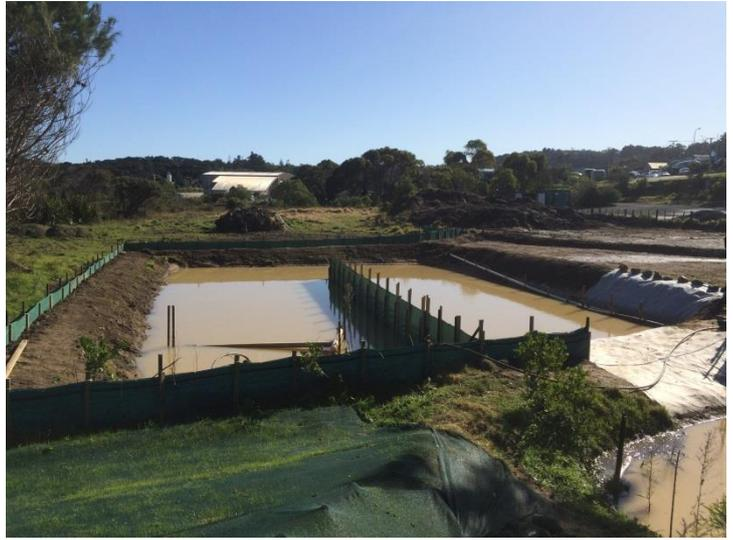
**Figure 67: Example of baffles**
