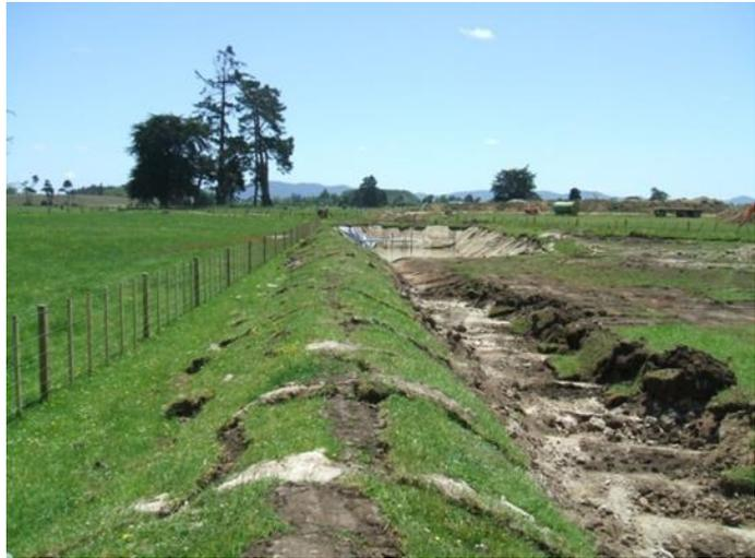
**Figure 15: Turfing scraped from within the site to stabilise the perimeter bund. The perimeter bund provides both clean and dirty water control**
