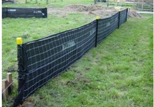
Figure 86: Super silt fence
