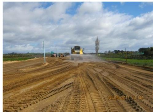
**Figure 128: Water truck dampening down the works area**
