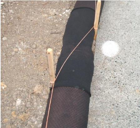
**Figure 92: Silt sock joined using a sleeve and pegged and secured using bailing twine with 1 m overlapping joint**
