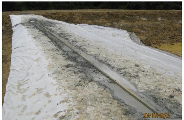
**Figure 68: Example of a level spreader**
