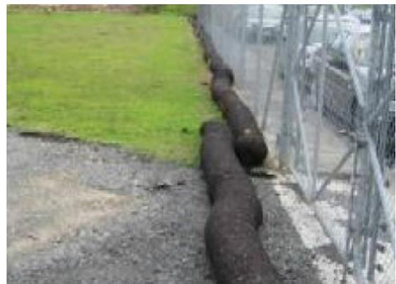
Figure 91: Silt sock with 1 m overlapping joint
