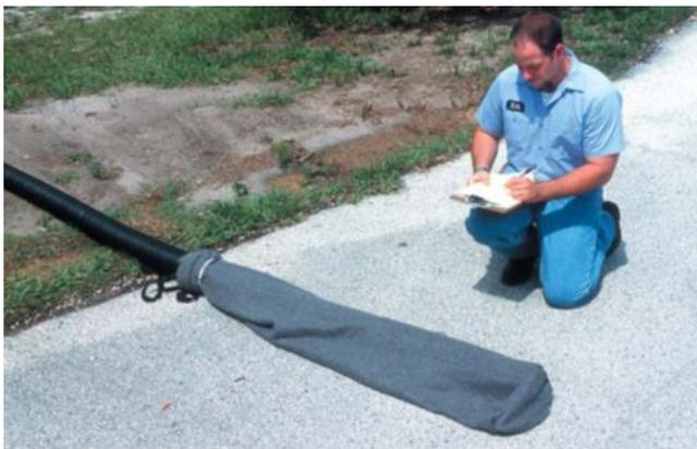
Figure 105: Dewatering bag and pipe sock
