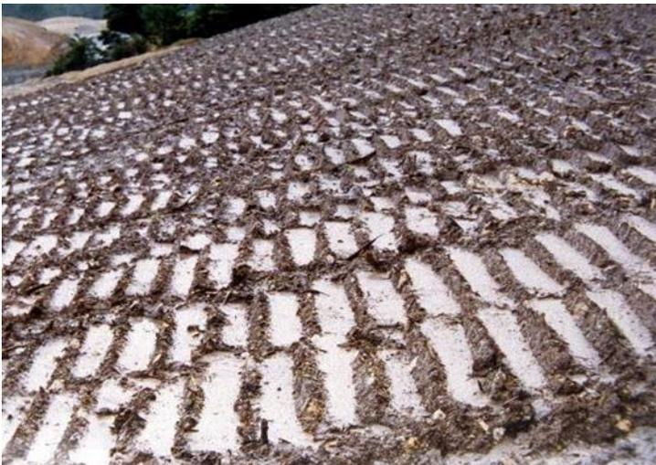
Figure 39: Surface roughening of a slope. Note the hollows acting as "micro" sediment traps
