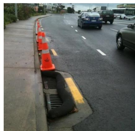
**Figure 98: Installation of a silt sock to provide some protection to the catchpit**
