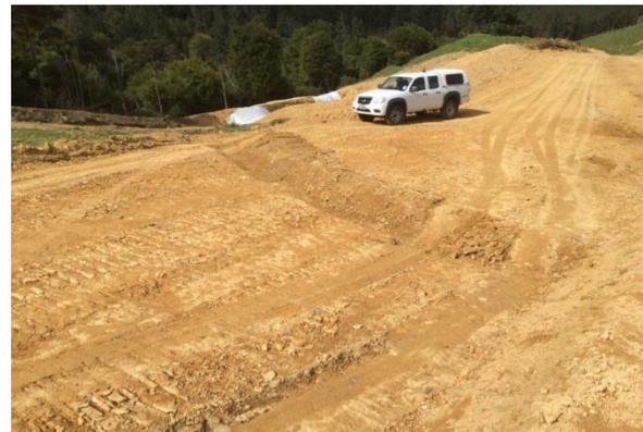
Figure 22: Contour drain installed across access track
