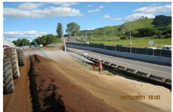
**Figure 127: Dust suppression using soil binders/polymers**
