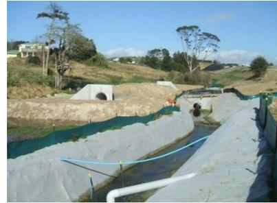
**Figure 112: Stabilised clean water diversion and temporary culvert to divert streamflows while a new culvert is being constructed**
