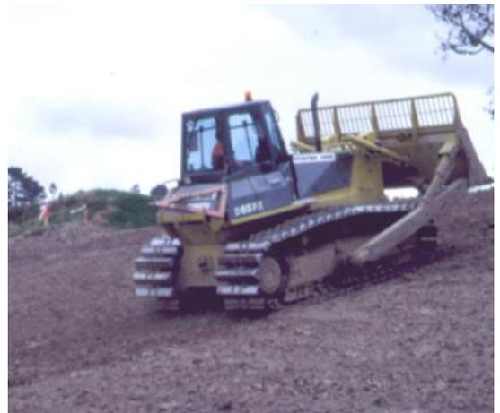
Figure 38: Surface roughening with bulldozer
