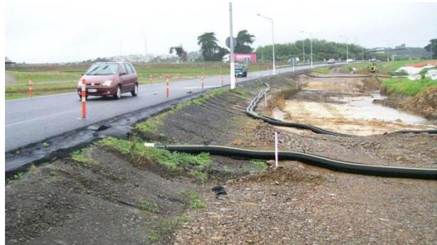
**Figure 29: Flume conveying clean water over the works area**
