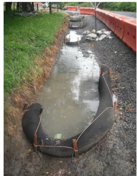
**Figure 26: Silt socks can be used as a check structure on a low gradient channel**
