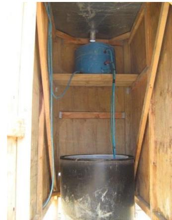
**Figure 102: Header tank**
