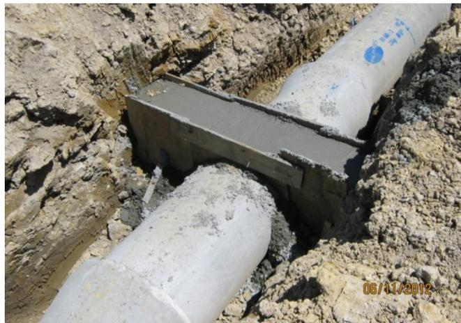
**Figure 70: Example of an anti-seep collar**
