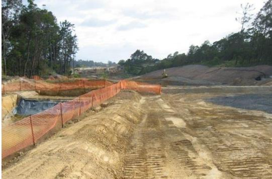
**Figure 19: Dirty water diversion bund directing site water to a sediment retention pond**
