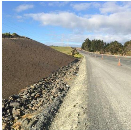
**Figure 56: Woodchip to stabilise the finished batter slope**
