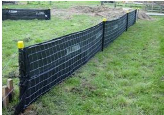
Figure 86: Super silt fence
