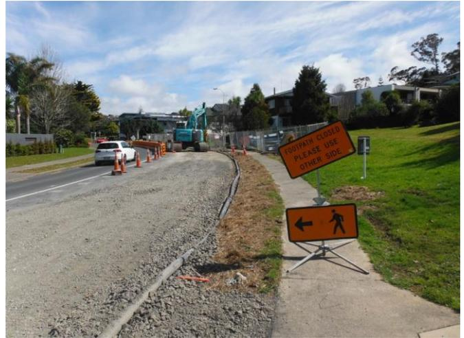
**Figure 109: Use of stabilisation products and progressive stabilisation**
