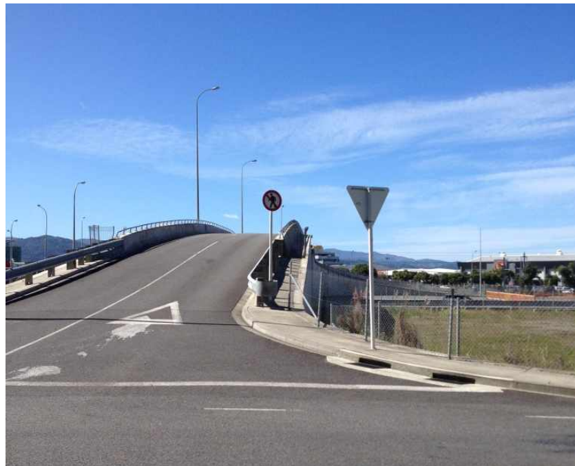
Figure 15 McKenzie Road Overbridge
