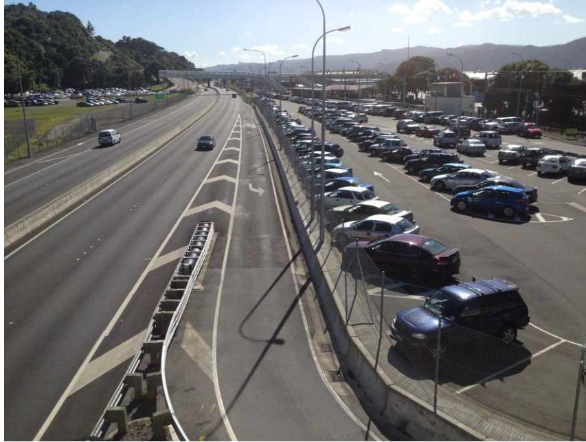
Figure 14 Shared path along Hutt Road, south of Petone Train Station
