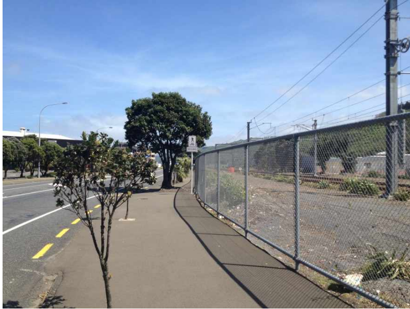
Figure 12 Shared path along Hutt Road, south of Petone Train Station
