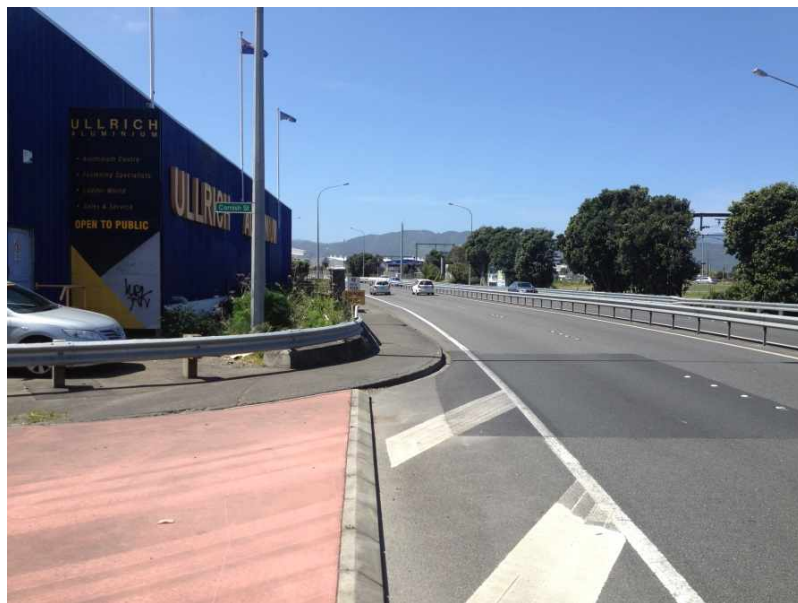
Figure 13 Shared path along Hutt Road, south of Petone Train Station
