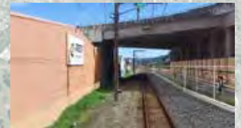
Dowse interchange overbridge
