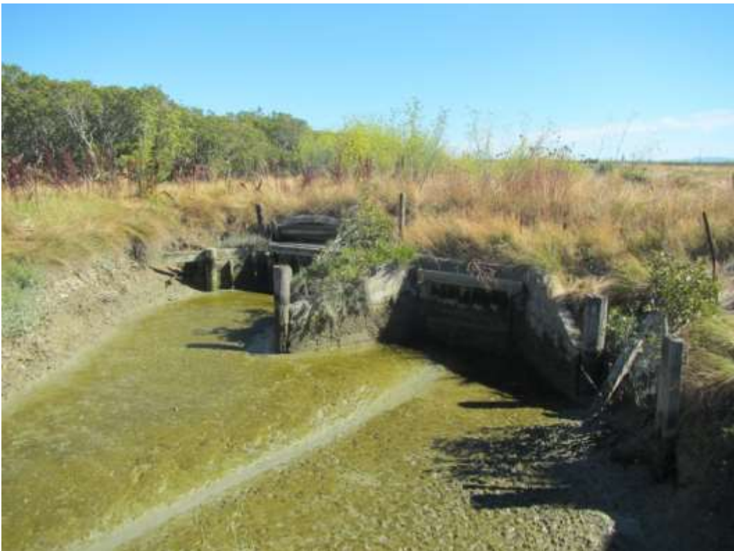
Plate 2: Culverts and flap-gates on the Pukorokoro Stream (Unit 6).
