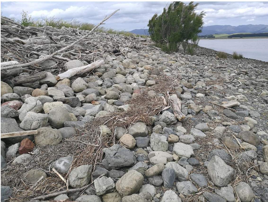
Figure 18: Wooden debris deposited on the exposed margin of the causeway road (Paul's Bank).
