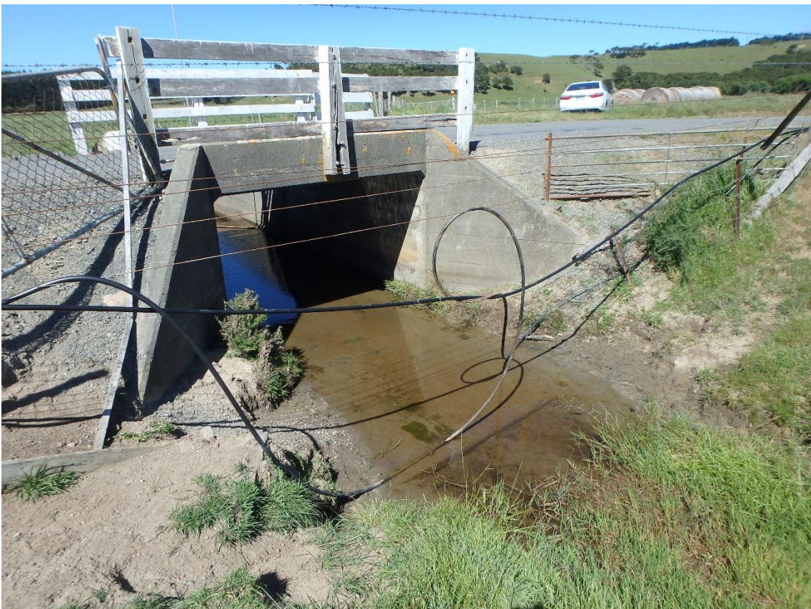
Figure 27: The box culvert under Western Lake Road. Note this culvert does not provide ideal fish passage but īnanga were seen upstream. 8/11/2017
