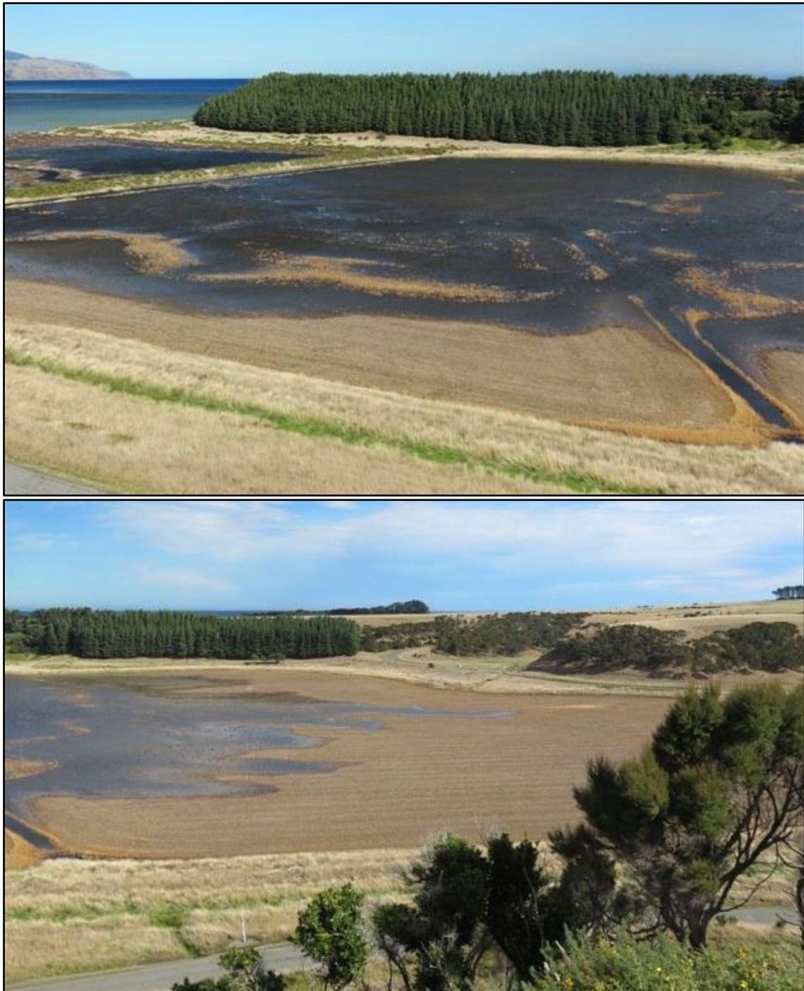
Figure 9: Views of the project area showing a flood event in April 2016. (Photos: Dougal MacKenzie)
