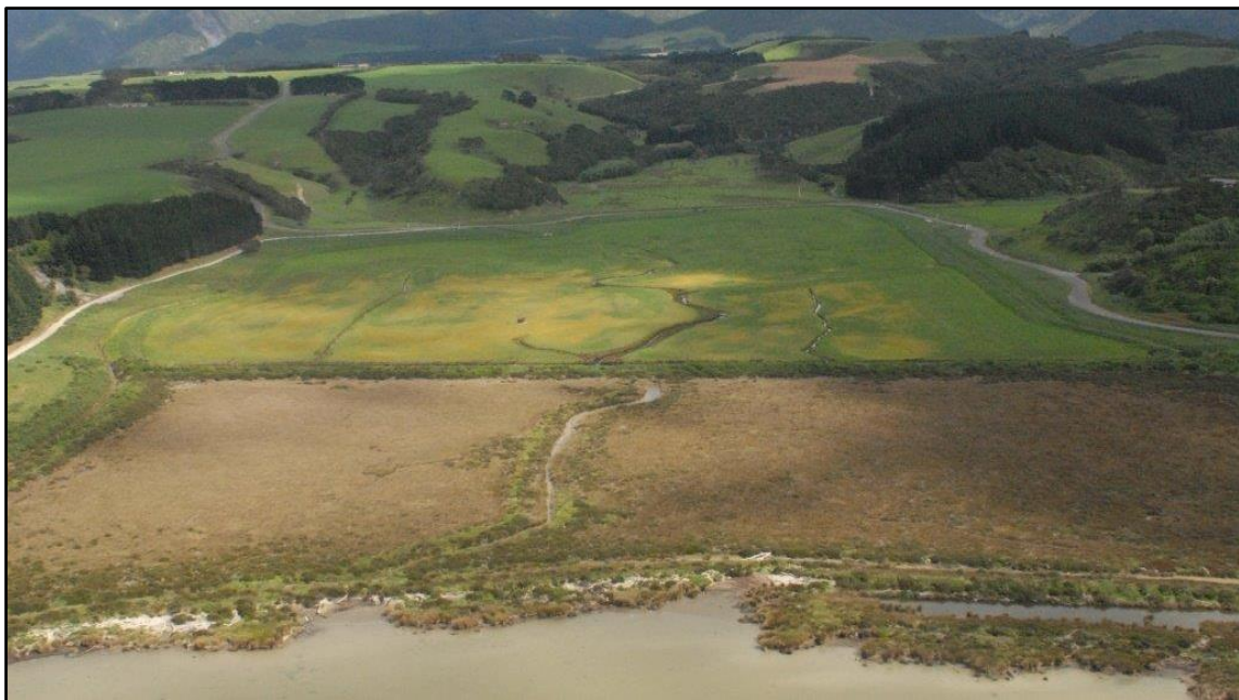
Figure 8: Recent oblique aerial view of the project area looking west showing the seaward and inner stopbanks 2/11/2017 (Photo: Tony Silbery, DOC).
