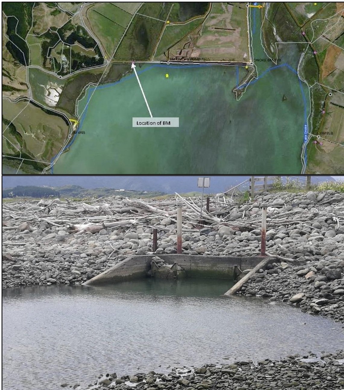
Figure 12: Location of former Wairarapa Catchment Board benchmark (BM) levelled during the field investigations. The elevation of this former WCB benchmark is not presently known but it can be readily levelled using other nearby benchmarks of known elevation. This would enable more accurate correction of the surveyed bed levels to MSL if required.
