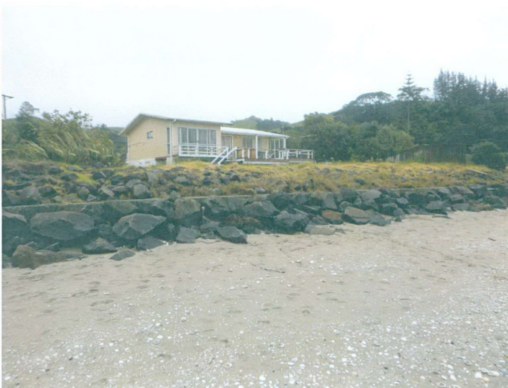
Photo 2: Typical profile for northern end of existing coastal protection structure
