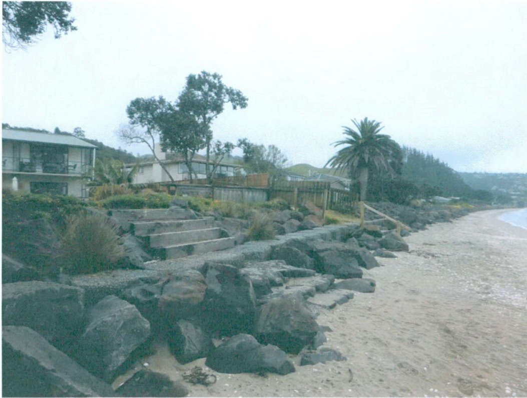
Photo 5: Typical section at southern end of the existing structure
