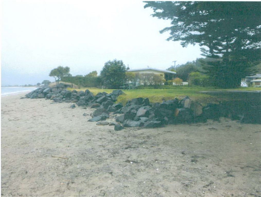
Photo 1: existing structure in Macrocarpa Reserve – administered by Thames-Coromandel District Council.
