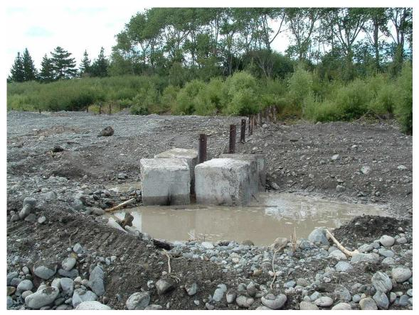
Figure 5-4: Completed debris fence (Otaki River)
