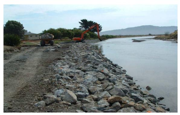
Figure 5-3: Rock rip rap construction on the Waikanae River at Otaihanga
