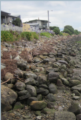
Erosion and flood protection adjacent to Foxton Beach settlement.
