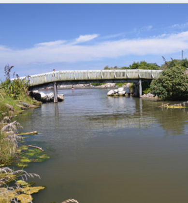
Mowhanau Estuary just upstream of bridge showing excessive algal growth
