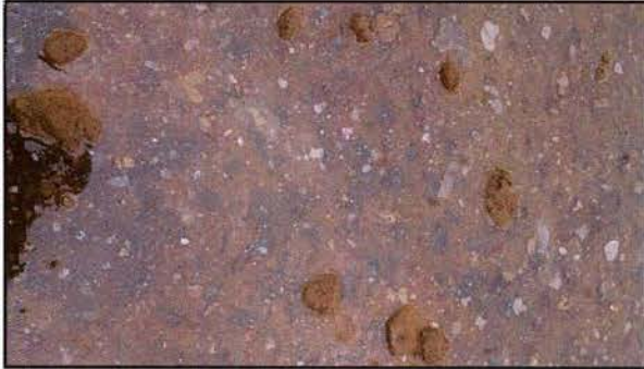
Photo 7: Surface water contained an oily film.
