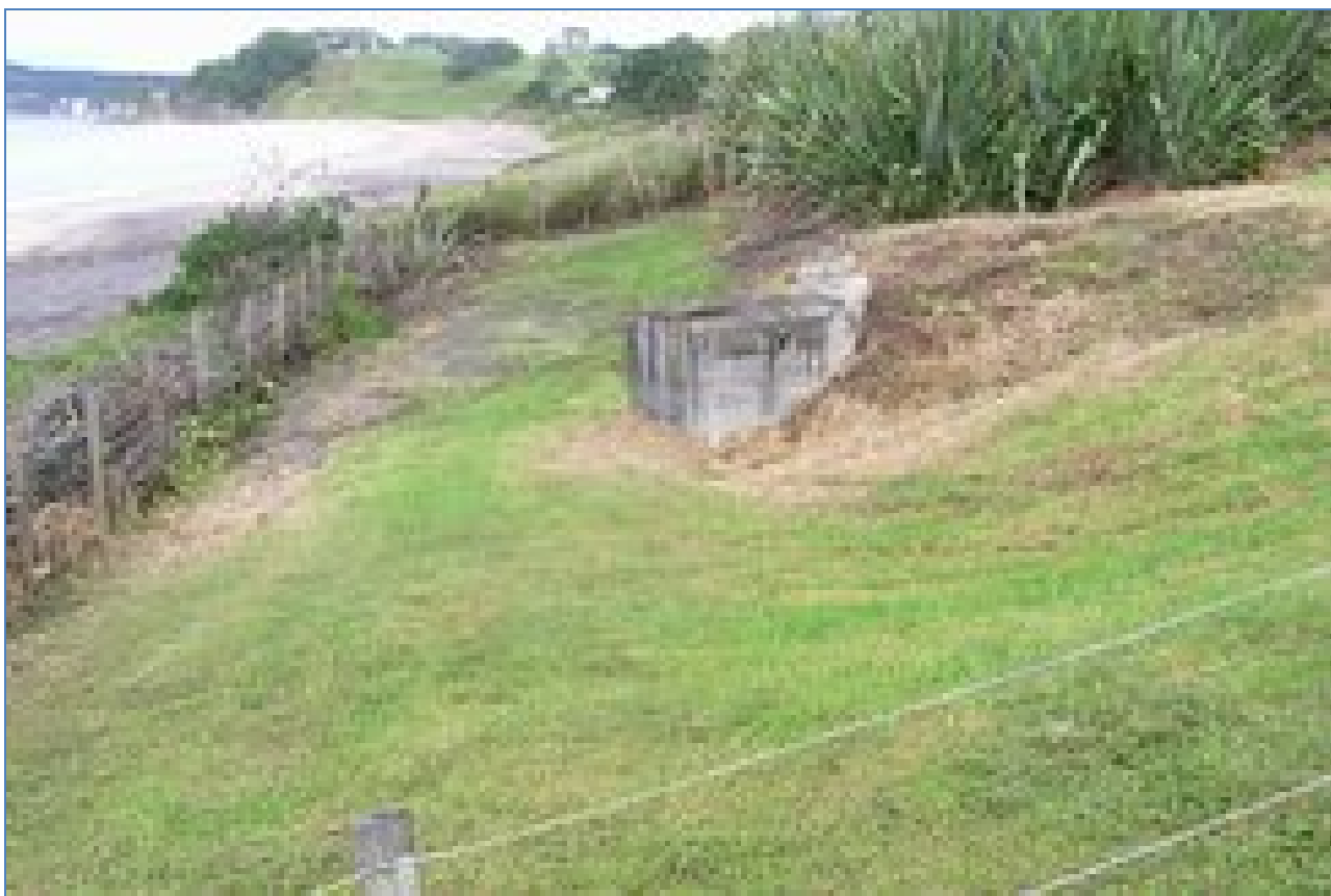
Figure 22: Concrete structure at beach profile site CCS22.
