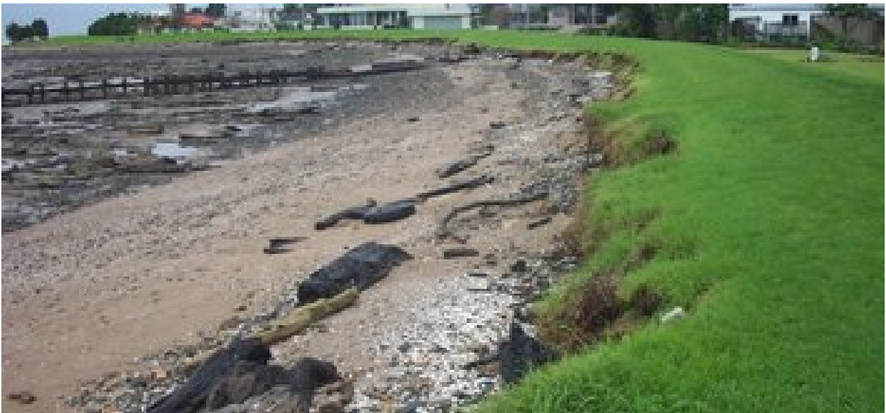
Figure 59: Erosion threatening flood protection embankment in July 2005
