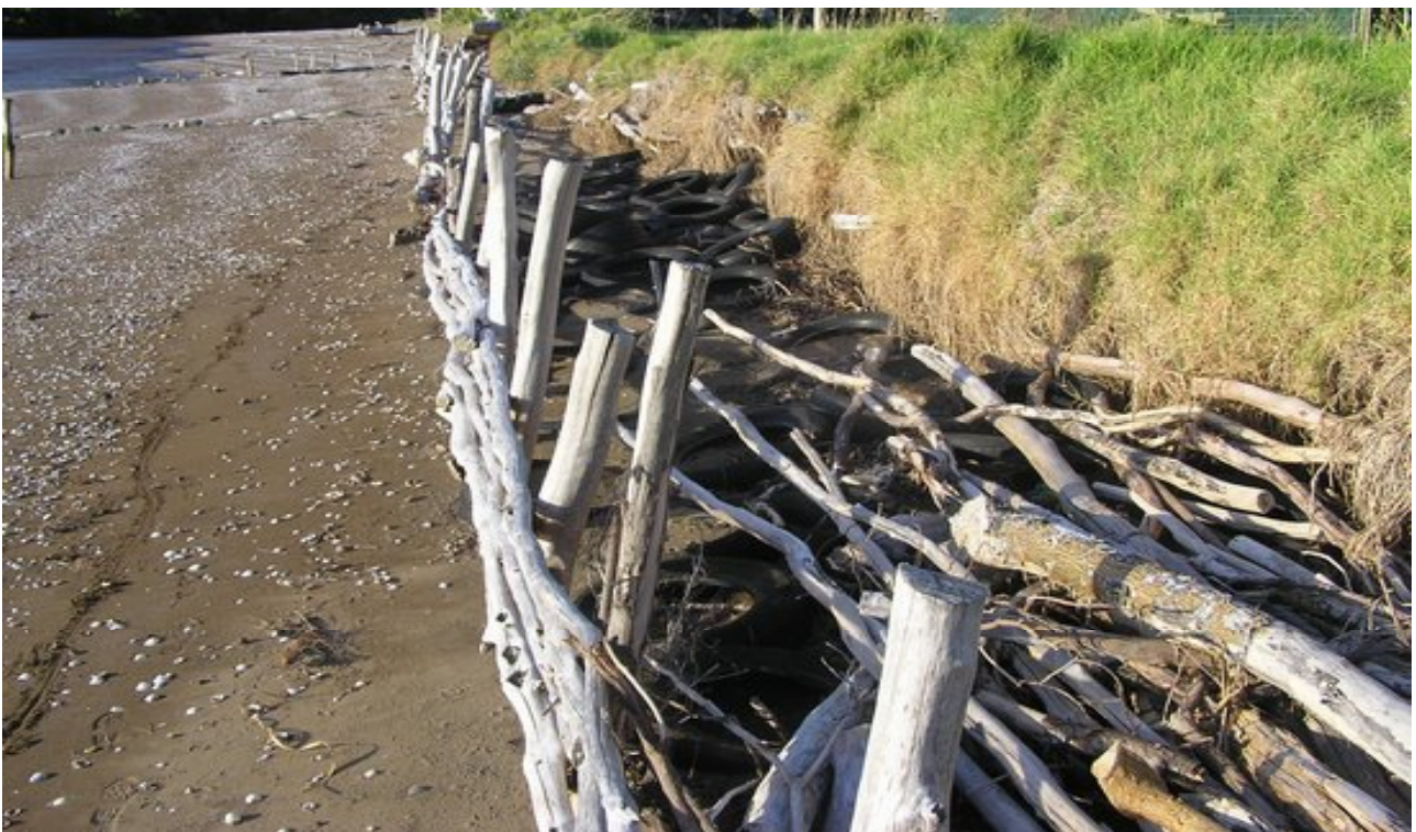
Figure 53: View of erosion at Port Charles east of CCS 6/1
