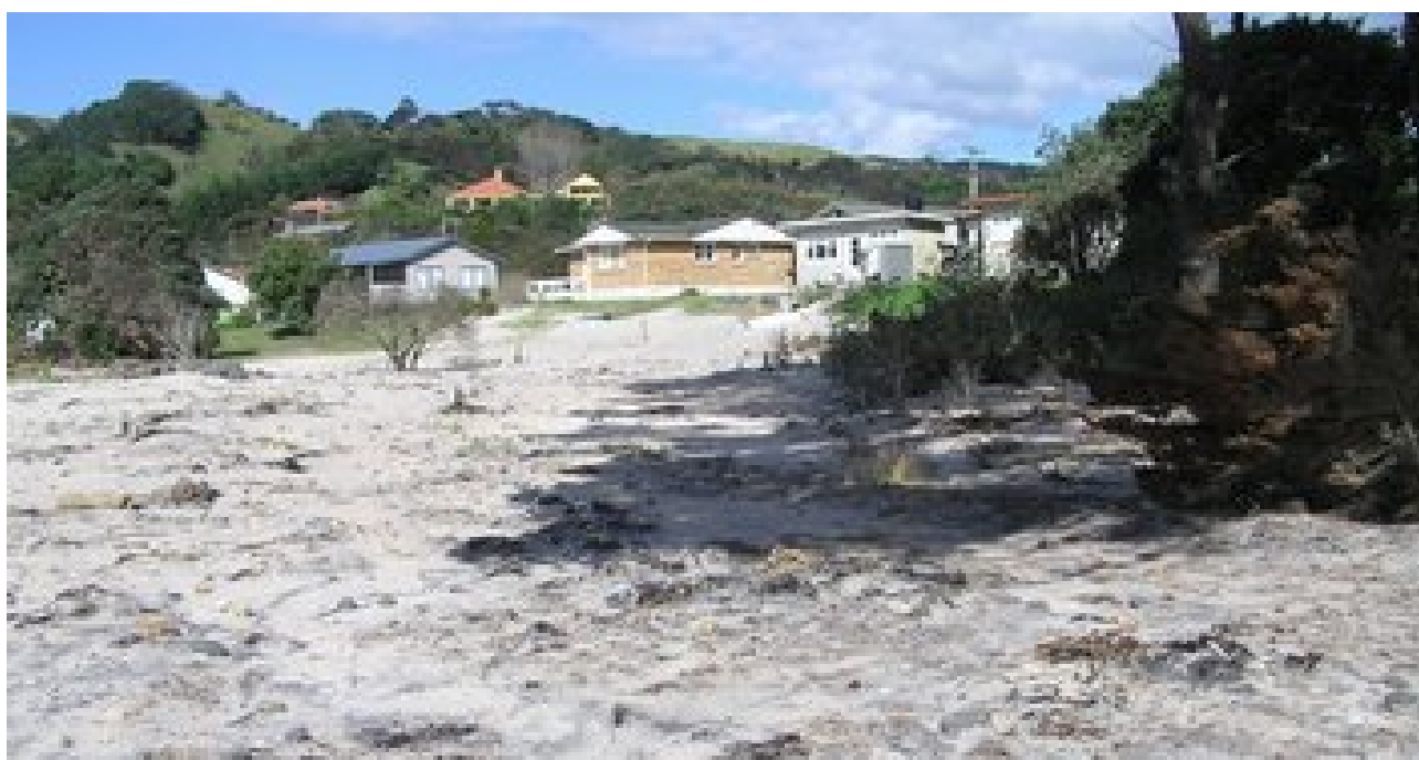
Figure 34: Eastern end of Kuaotunu Beach near Kuaotunu River mouth following storms of July and August 2008 showing areas subject to wave overtopping and run-up.
