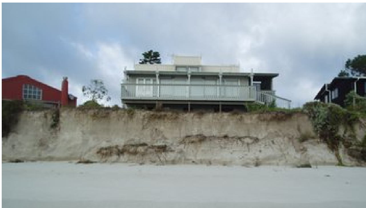
Figure 48: View of erosion scarp in central-southern beach following storms of July and August 2008 (Photo: Meg Graeme – taken August 2008).
