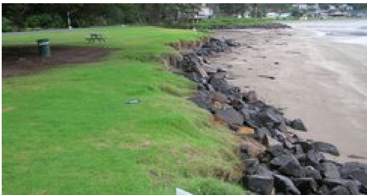
Figure 17: View in vicinity of CCS 25 (line of profile is approximately indicated by the tape measure evident centre-left). Tarapatiki Stream is evident in the middle background. The shoreline behind the photographer consists of a rock and concrete mass block seawall extending approximately 350 m alongshore (fronting private beachfront properties). The wall holds the shoreline seaward of the natural shoreline position with a high tide beach only rarely occurring. There are significant end
