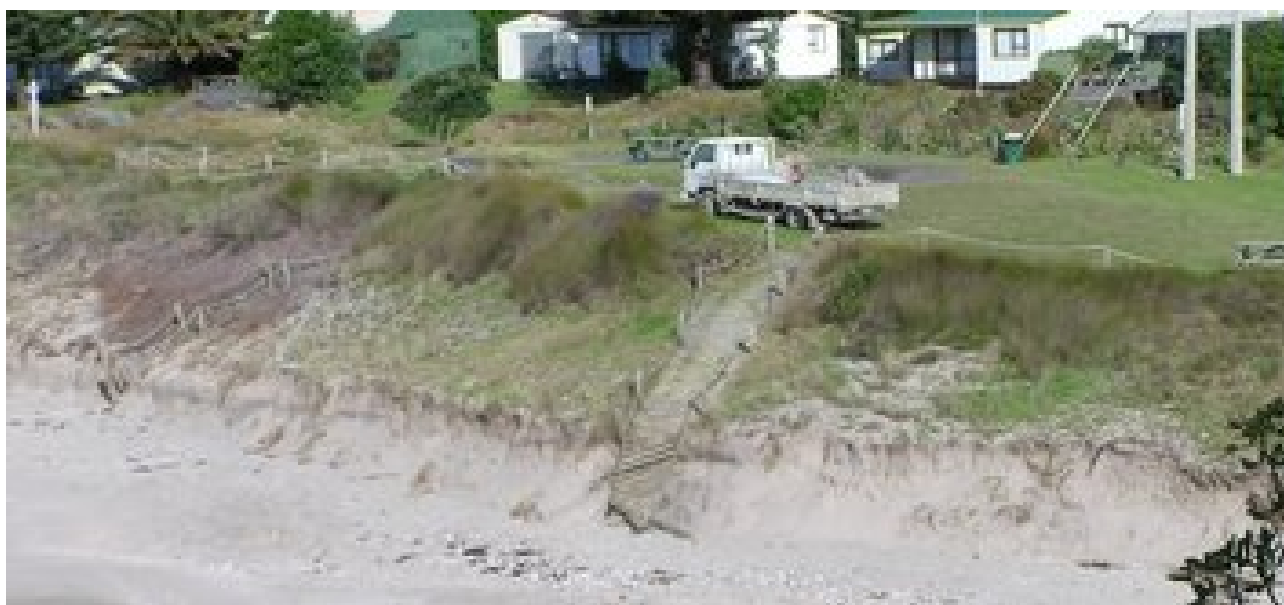
Figure 37: Dune toe erosion at very north end of Rings Beach following storms of July and August 2008
