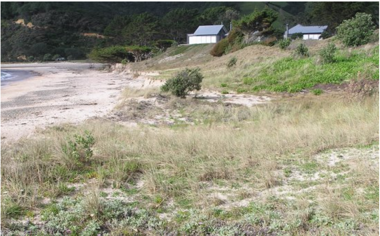
Figure 33: View along part of Kuaotunu East beach before and after mid 2008 erosion. The low dune areas landward of the 2008 erosion suggest this erosion is exceeded on occasions - probably extending back to the higher dune area behind.
