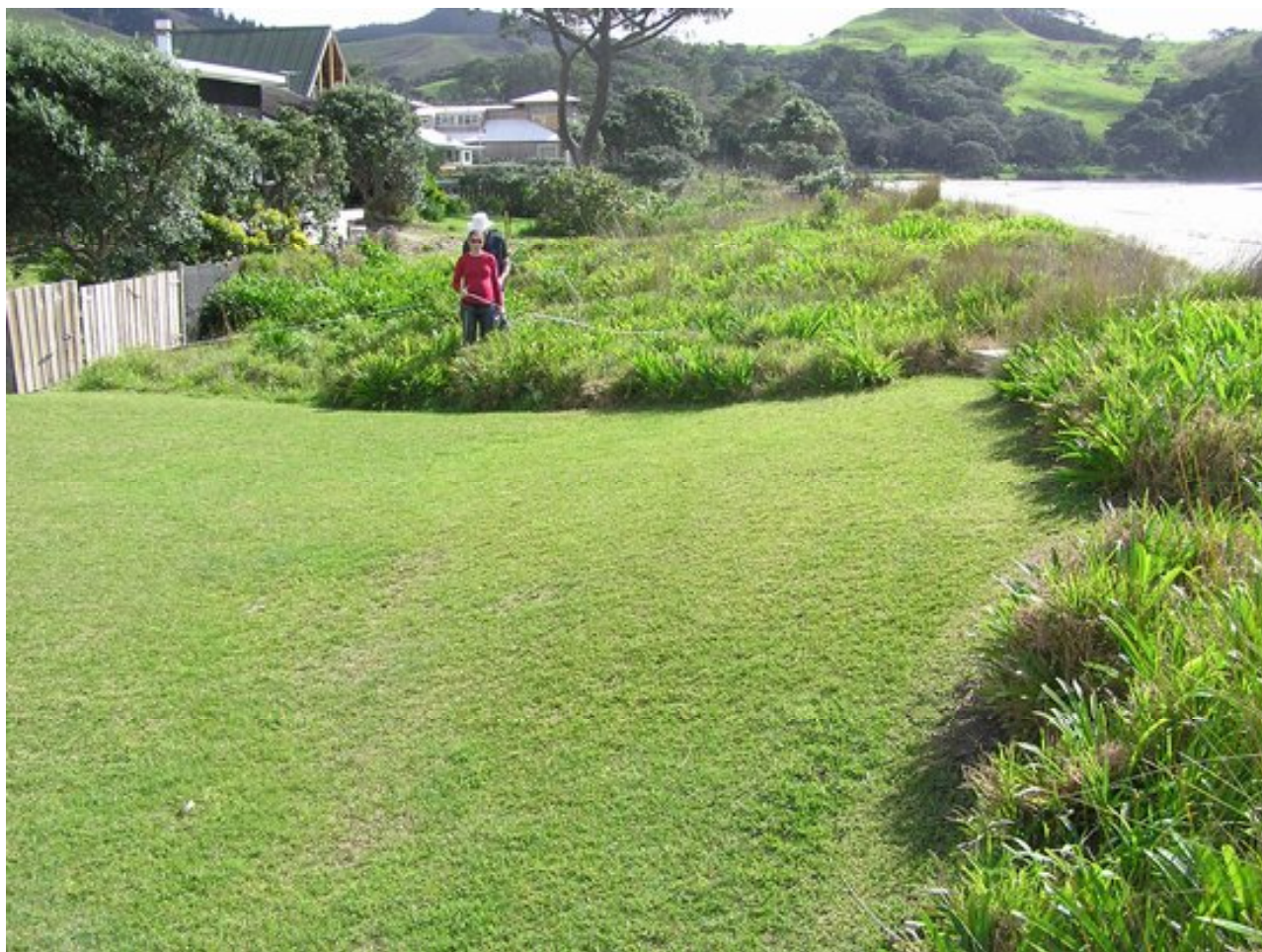
Figure 45: Location of worst estimated erosion in swale behind frontal dune.
