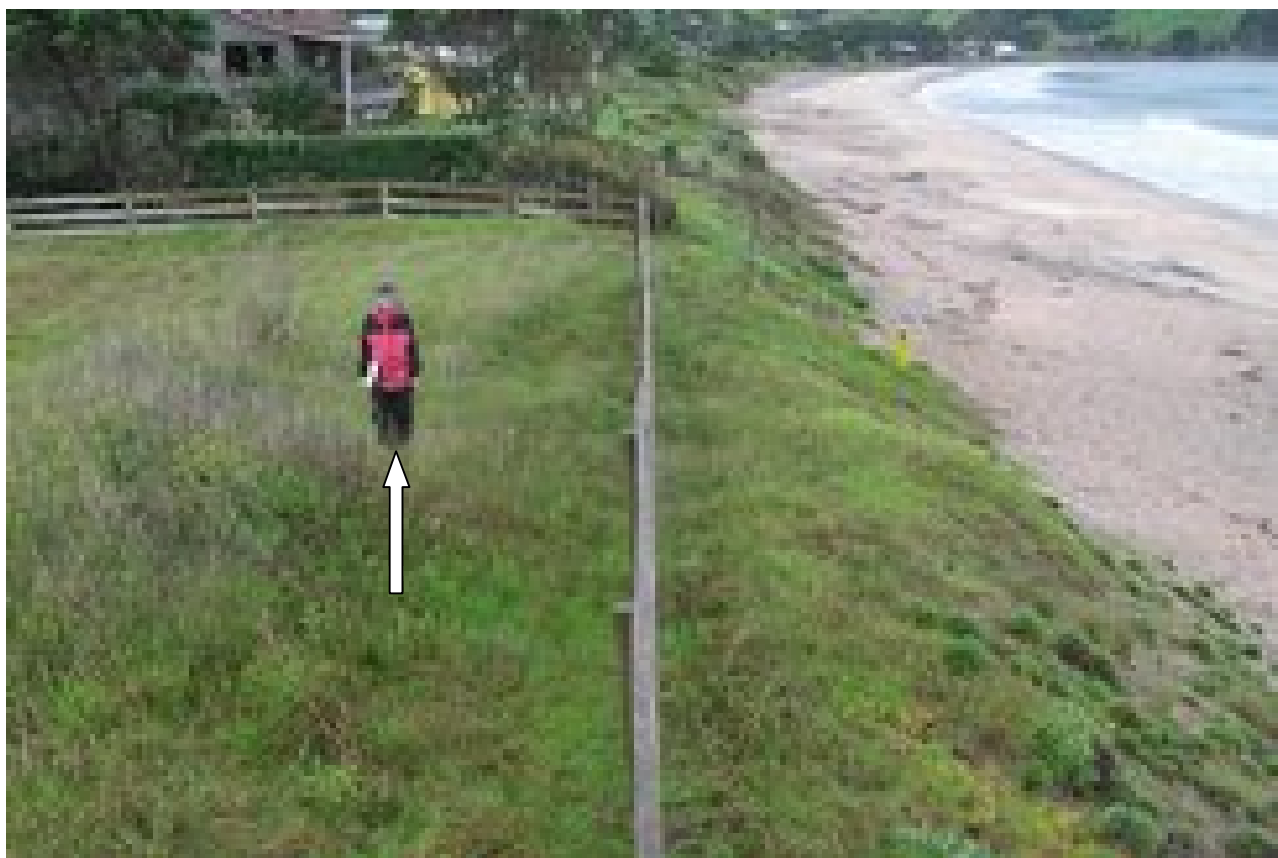
Figure 23: Most severe calculated erosion at ground level (arrow) at Wharekaho CCS23 (excluding safety factors).
