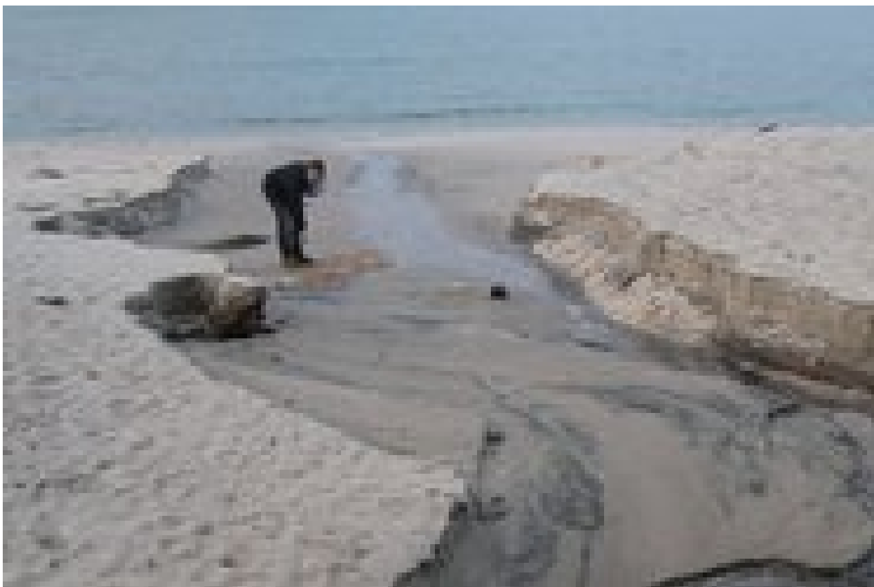
Figure 16: This creek bed at the southern end of Maramaratotara Beach contains erosion resistant materials under a thin layer of sand.
