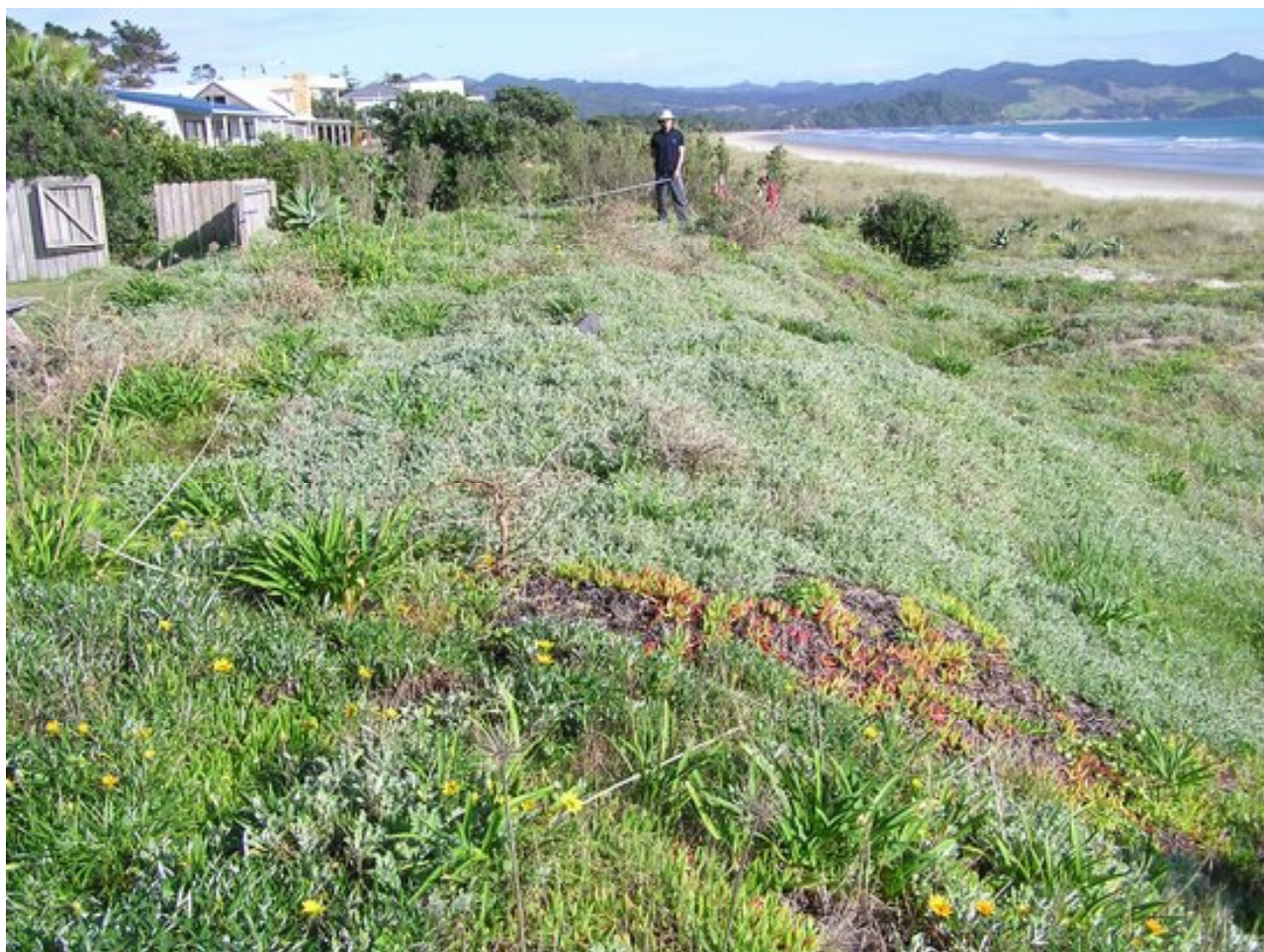
Figure 42: Location of worst estimated erosion (ground intercept excluding safety factors) at CCS 13. The estimate is close to (but landward of) historic erosion scarps but field evidence suggests the revised PDS (with the 10 m safety factor) is adequate.
