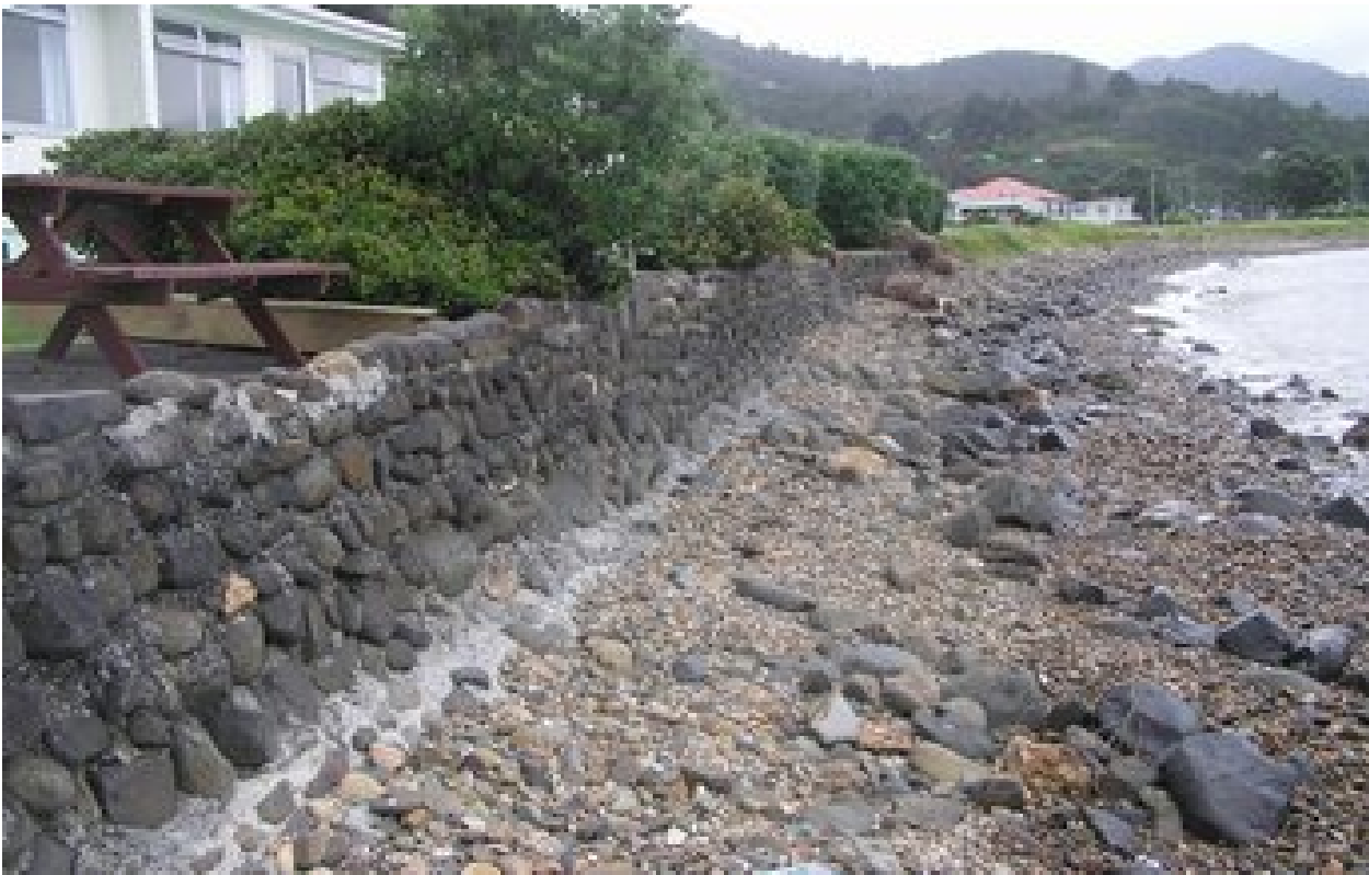
Figure 67: Seawall fronting motel south of Pohue Stream
