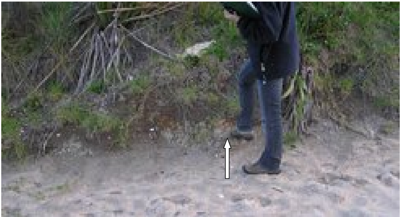
Figure 15: Erosion resistant material exposed in bank behind beach in the vicinity of profile site CCS28.
