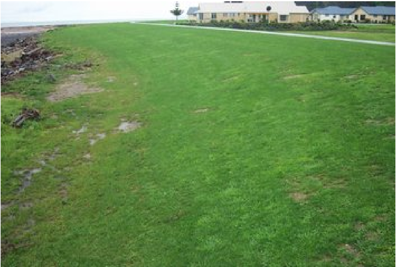
Figure 58: Flood protection embankment and footpath constructed north of Wilson Street
