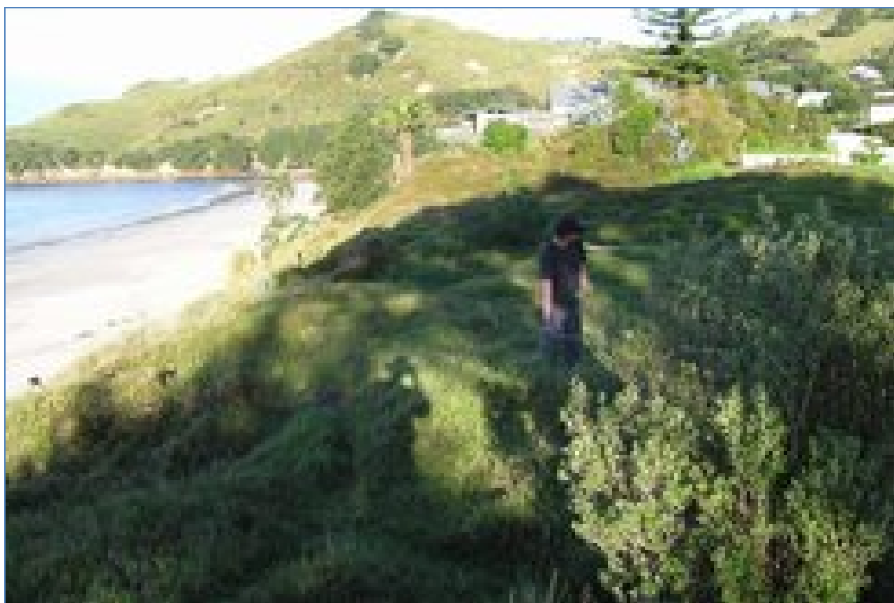
Figure 13: Worst estimated erosion at ground level at the south end of Hahei Beach (CCS33).
