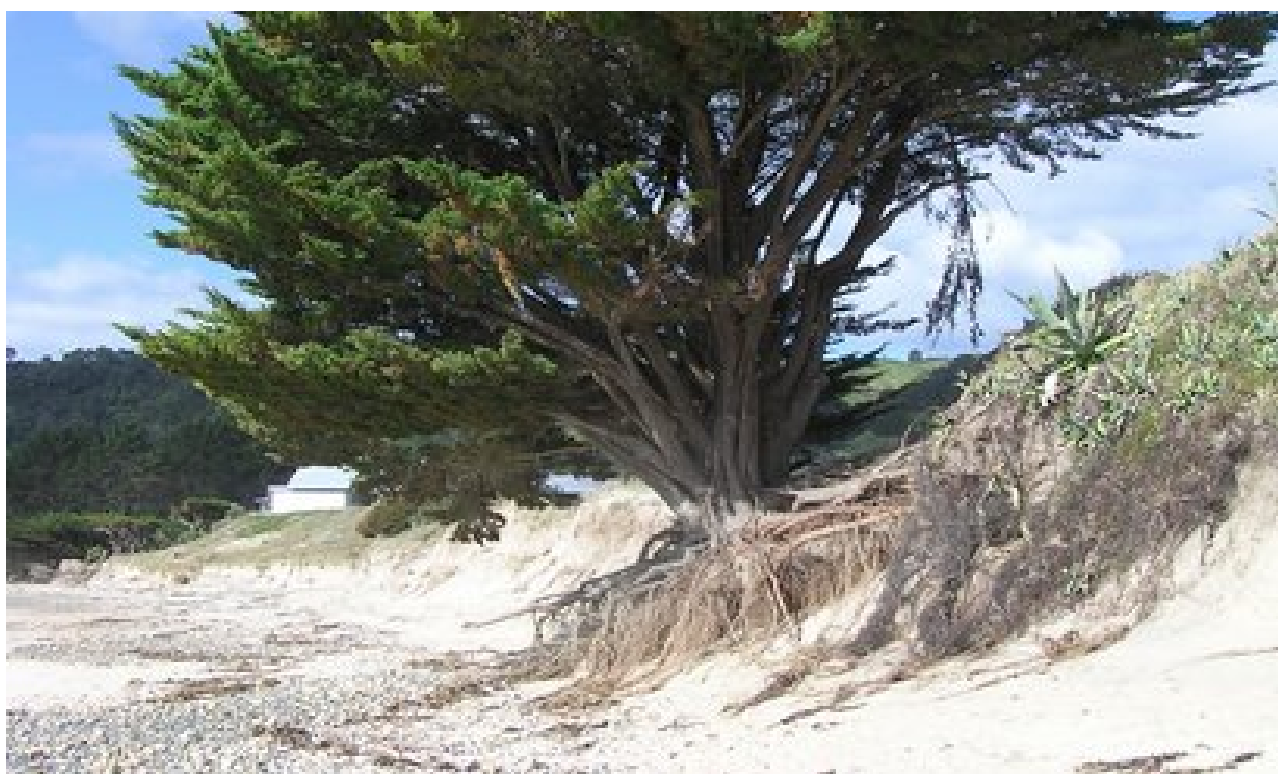
Figure 32: Large macrocarpa near top edge of dune face north of beach profile site CCS20/2 – before (top) and after (bottom) severe erosion of July/August 2008).
