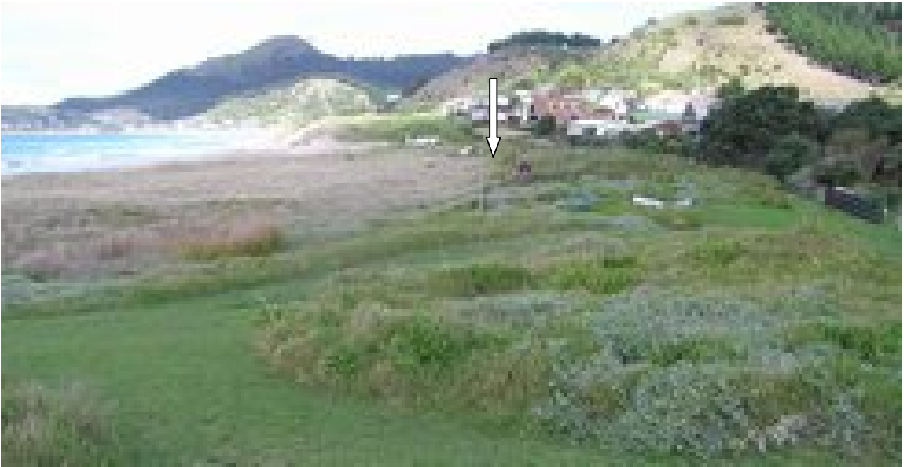
Figure 26: Photo looking south at CCS 49. Arrow indicates approximate location of worst measured erosion (old erosion scarp), largely relating to past stream changes.
