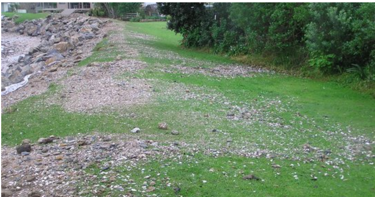
Figure 60: Overtopping and erosion September 2005, leading to placement of rock to protect flood embankment
