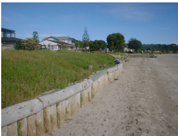
Plate 13: Cooks Beach has a range of examples of erosion protection structures
