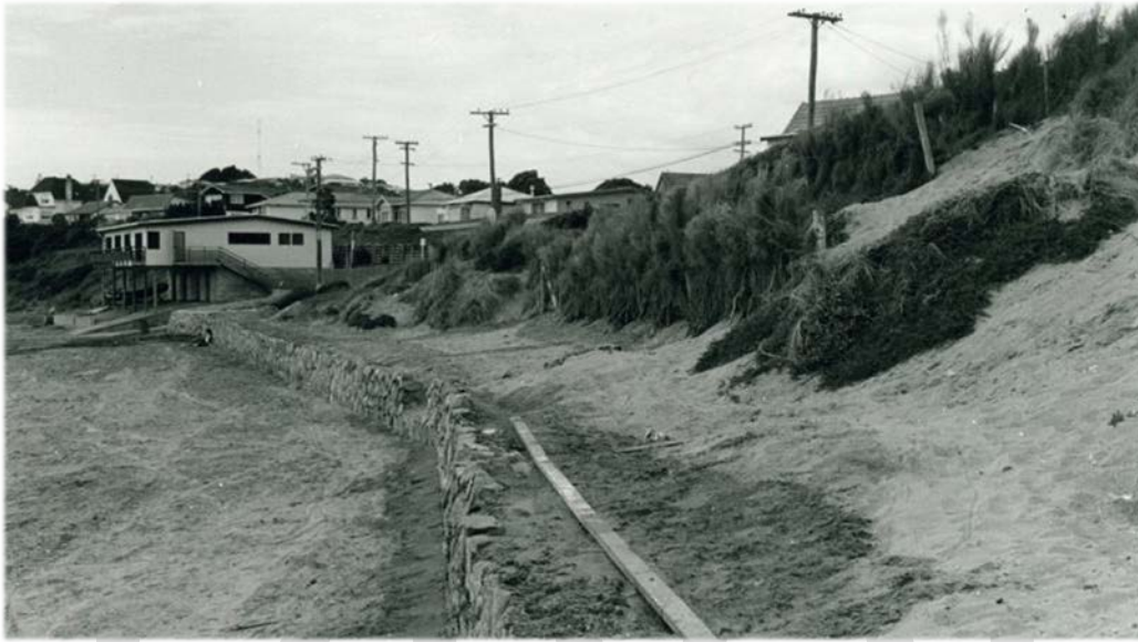
Figure 24: Titahi Bay seawall immediately following construction (photo GWRC).
