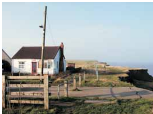
The house in this photo taken at Aldbrough at the end of 2005 has since been demolished for safety reasons when its front room was lost to the sea!
