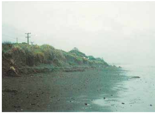
Storm damage at Paekakariki
