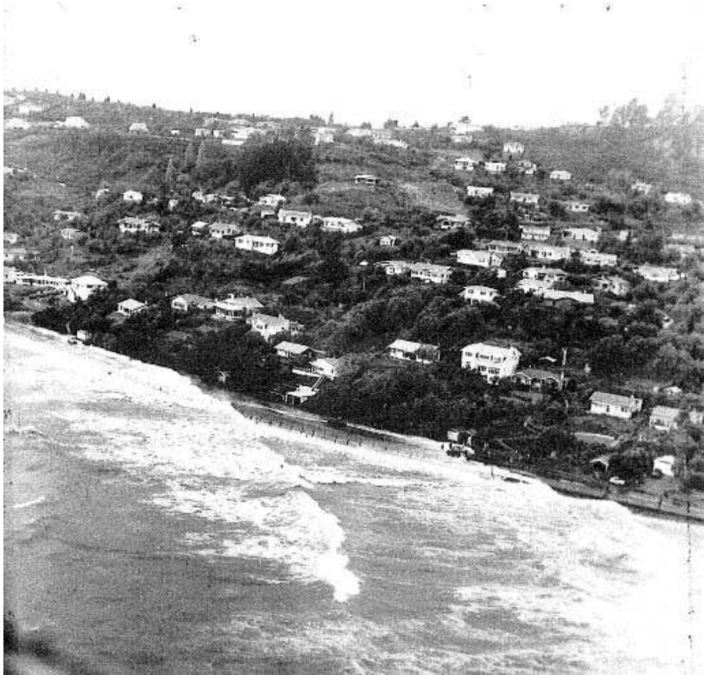
Figure 4-4: Aerial photograph of wave set-up and run-up at Rocks Road taken at ~13:00 during the 19 March 1957 storm. [Supplied by M. McGuire, Port Nelson].
