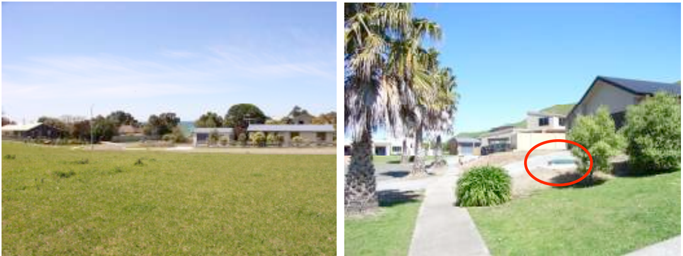
Figure 7 New housing developments inland directly off the main beach-access road. Each house has an on-site water capture and storage, with drinking water storage of new houses usually located under the house. Each property has an individual on-site wastewater treatment system. Septic tank systems are often in front yards (top right red circle, and Figure 7), which leaves little room for the system's drainage field. Thus, new coastal developments will increase effluent drainage down the natural gradient to towards the increased population density along the beachfront housing.
