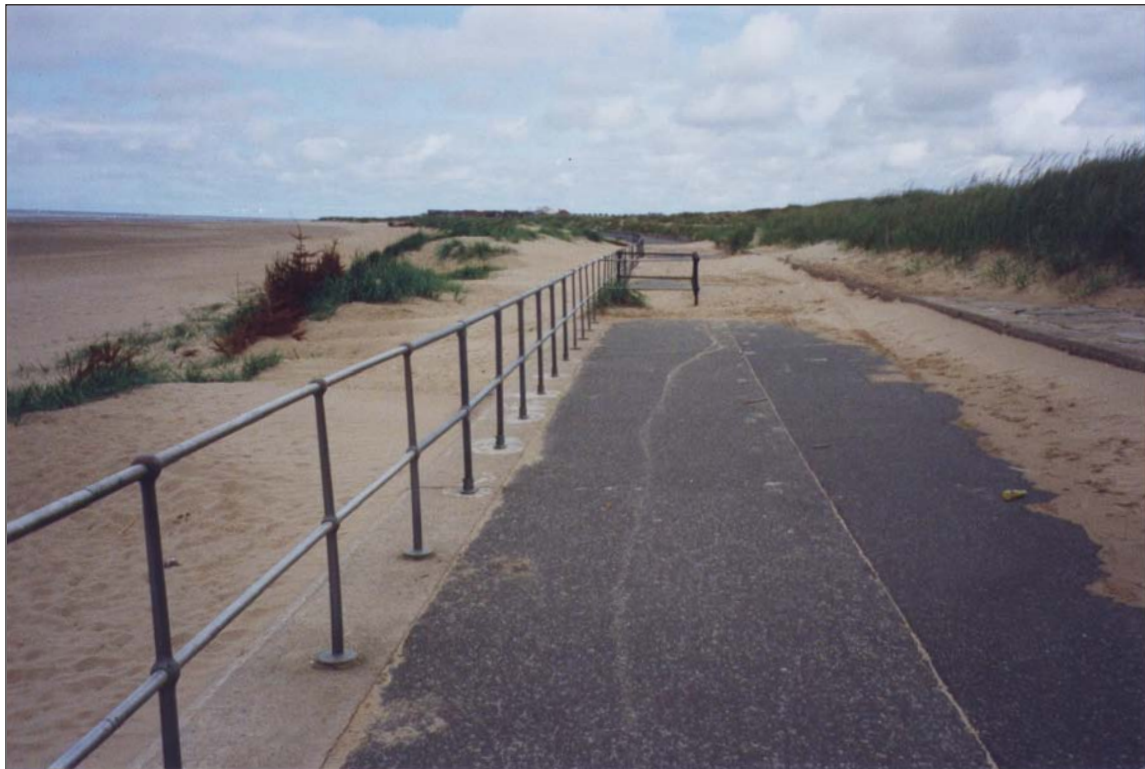
Plate 1.9 Accumulation of blown sand on the promenade at Crosby, northwest England. Sand invasion poses a significant problem to properties located to the right of the picture.
