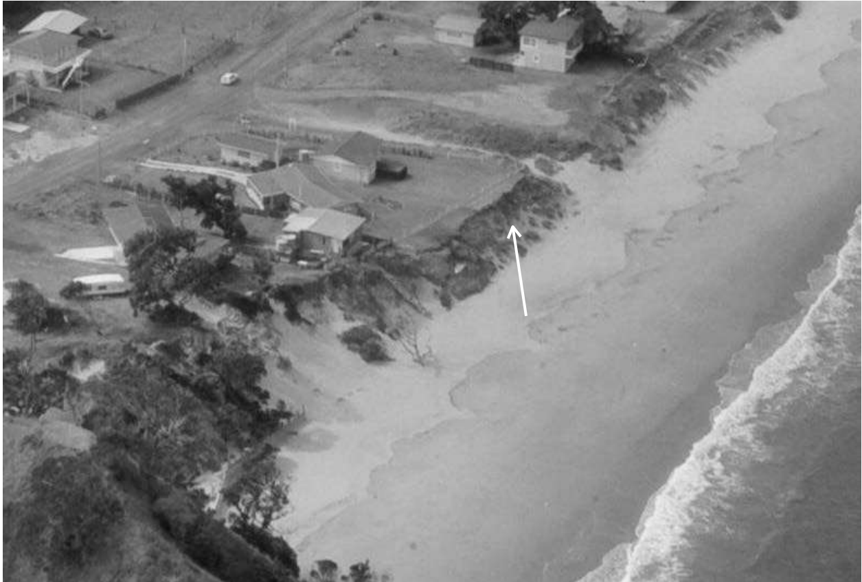
Figure 11: Photograph of south end of beach taken in April 1976. Note evidence of recent dune face erosion (arrowed). The subsequent July 1978 event extended erosion within some of the property boundaries in this area and also partly undermined the house nearest the bank (see Figure 9). The properties in the area of the arrow (14-18 Whangaumu Road) were levelled at or shortly after subdivision in the early 1960's, extending the flat grassed areas seaward over an earlier erosion scarp. So there were earlier erosion events that extended further landward than shown. The vegetated dune face (i.e. absence of recent erosion) at the extreme western end (bottom left of photo) reflects protection then provided by a wooden sea wall. (Whites Aviation photo WA72365F, Alexander Turnbull Library).
