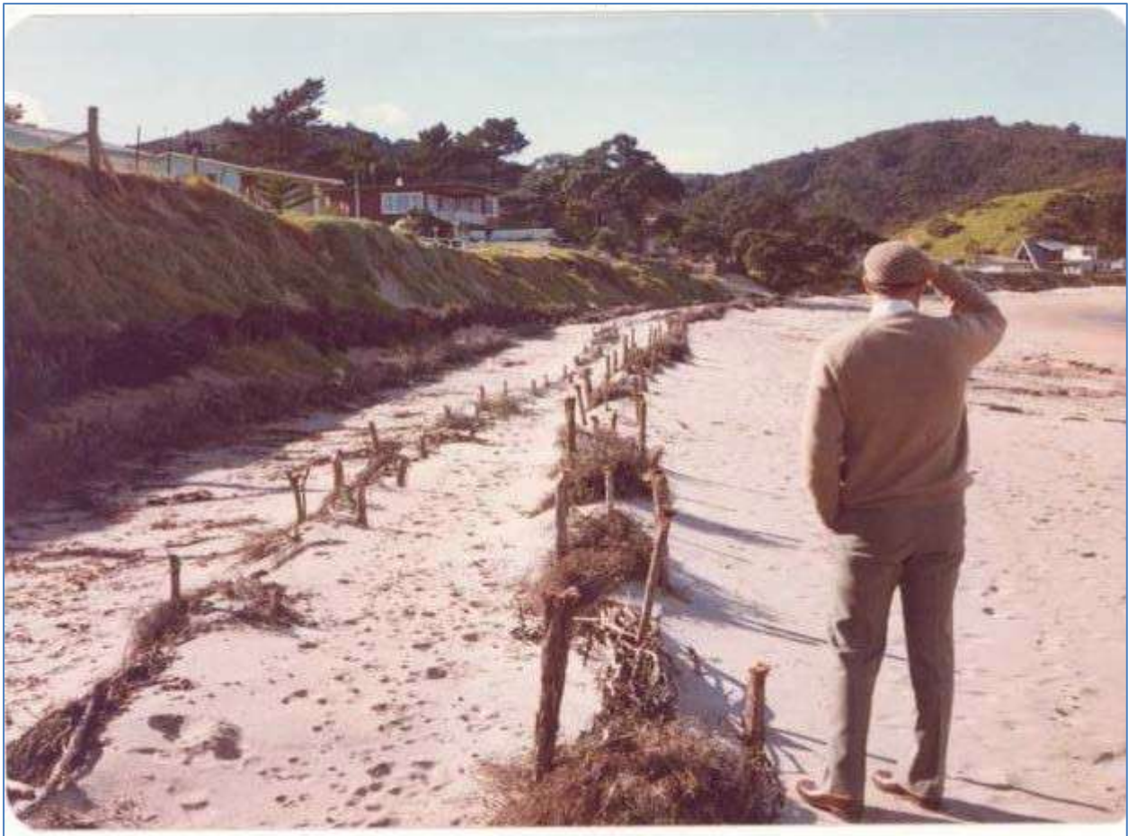
Figure 9: Severe dune erosion caused by storm of July 1978. The fencing (top photo), vegetation recovery on dune face (bottom photo) and the build-up around the brush dune fence (bottom photo) indicate the erosion occurred sometime before these photos were taken (Northland Regional Council photographs – believed to date from June 1979).
