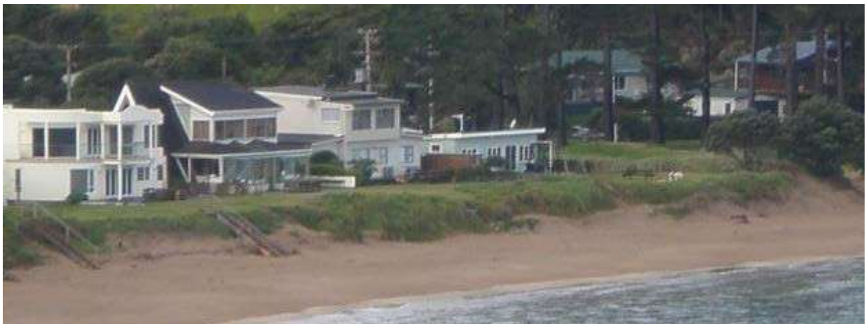
Figure 5: View of high dunes and rock revetment at western end of the beach (top) and dunes in central (middle photo) and eastern (bottom photo) ends of the beach
