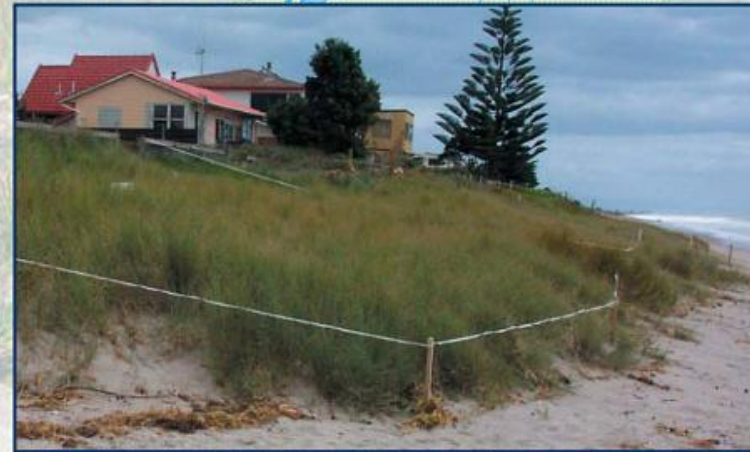
March 2004 Inexpensive planting of native dune species has re-created an accreting front dune, by Papamoa Coast Care helping to solve the erosion problems. This photo was taken the day after the impact of 10m waves from Cyclone Ivy.
