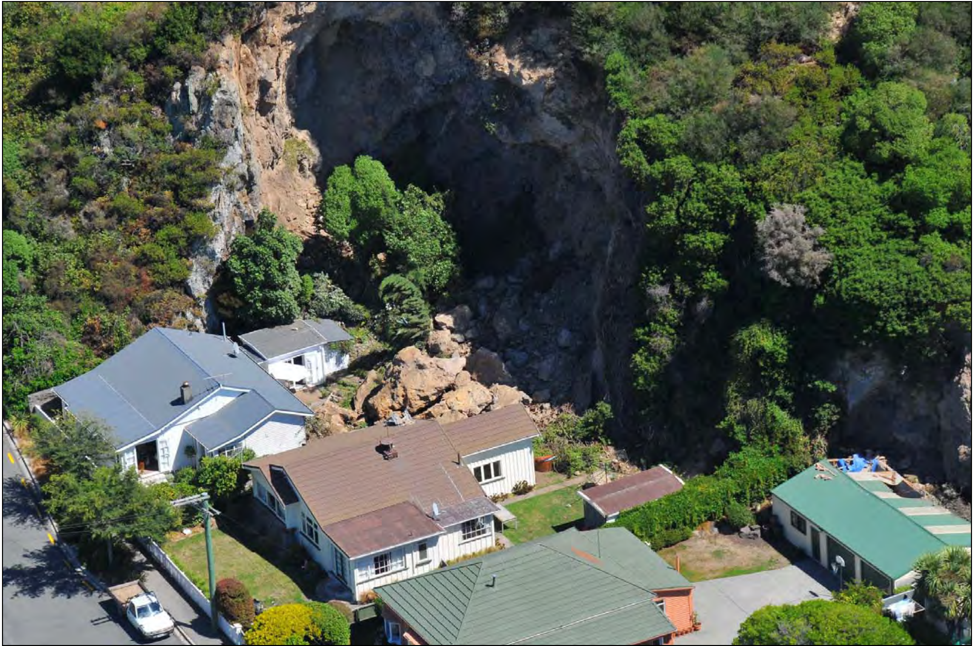
Photo 9. Fall of large boulders at the back of damaged houses at 11 (left) and 9 (centre) Richmond Hill Rd, Sumner ( GNS Photo-GTH_5727 ).
