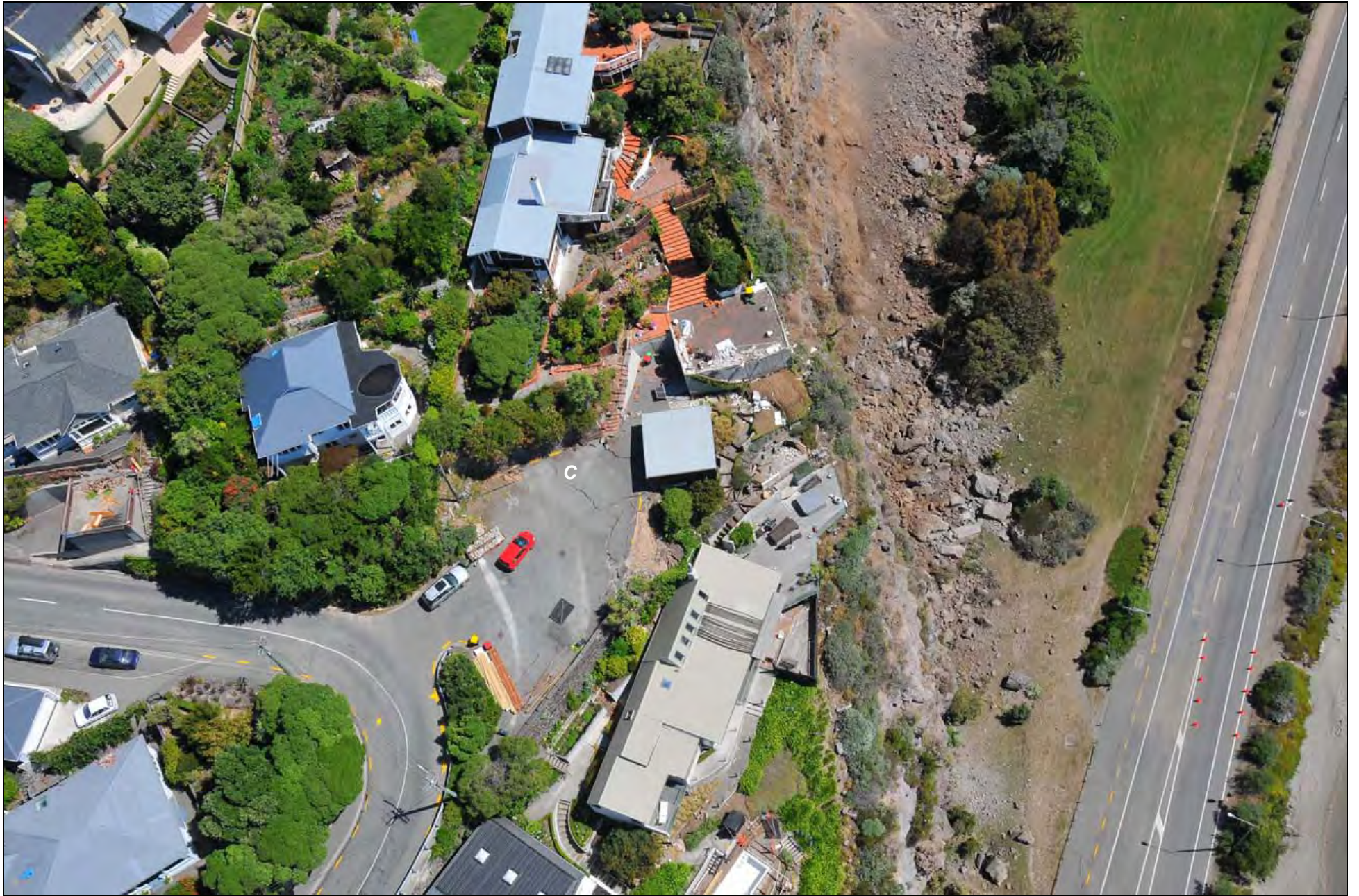
Photo 15. Rock falls and cracking (C) in Kinsey Tce, Moncks Bay (GNS Photo-GTH_5775).
