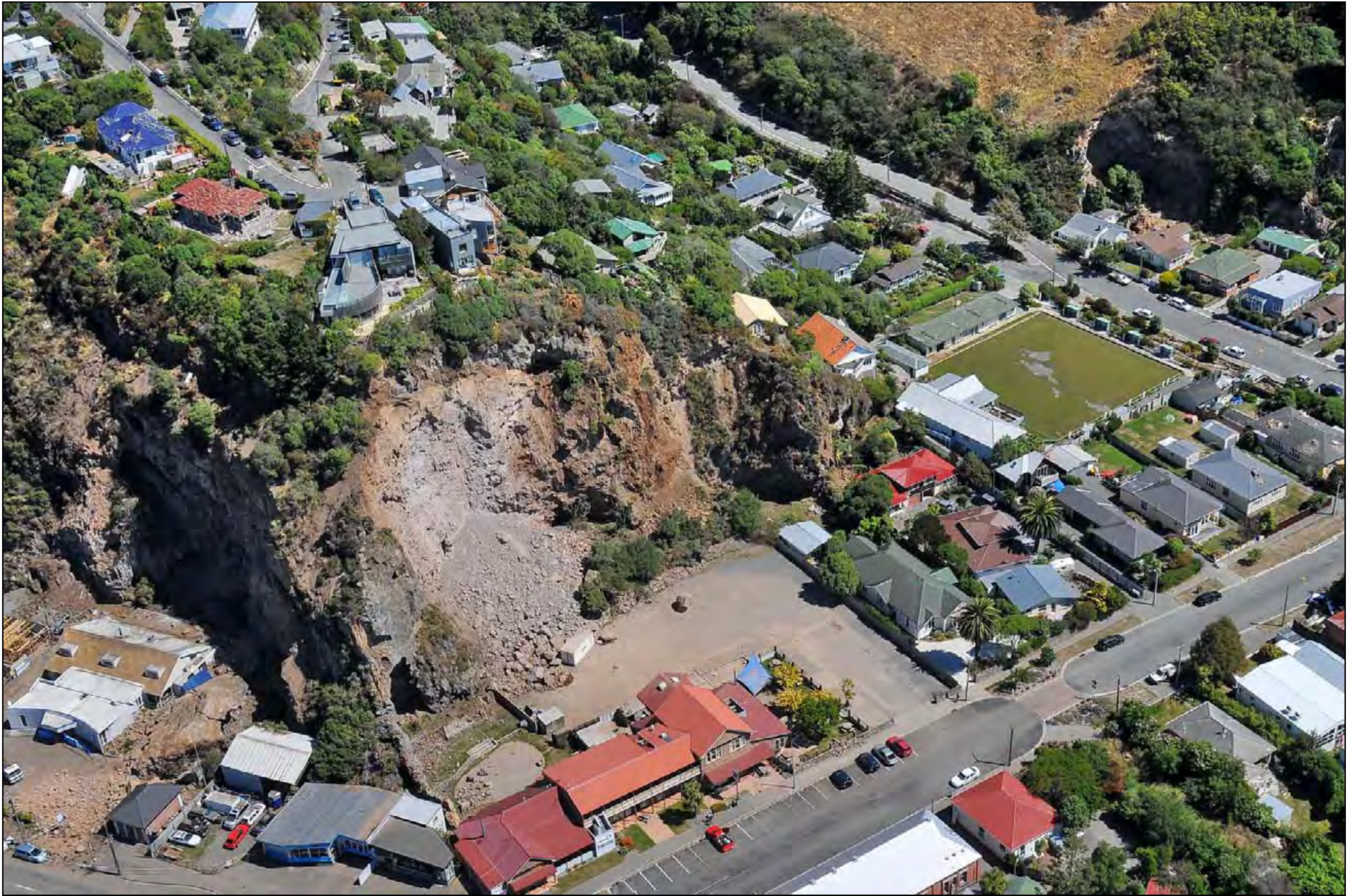
Photo 8. Rock falls at RSA and Marine Backpackers site, Sumner ( GNS Photo-GTH_5714 ). Note badly damaged houses top left (see Photo 8a - same location as Photo 8 ).
