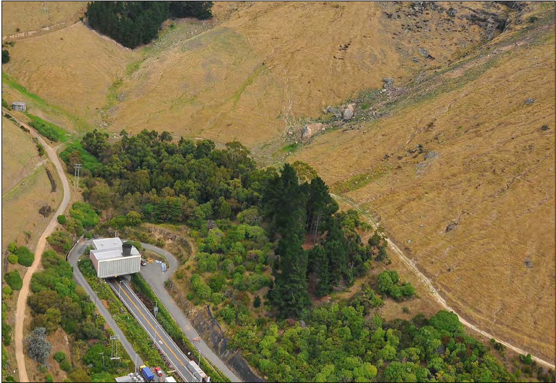
Photo 33. Large boulders from rock falls on Castle Rock (mainly during the 4 September earthquake) near west Tunnel Portal ( GNS Photo-GTH_6084 ).
