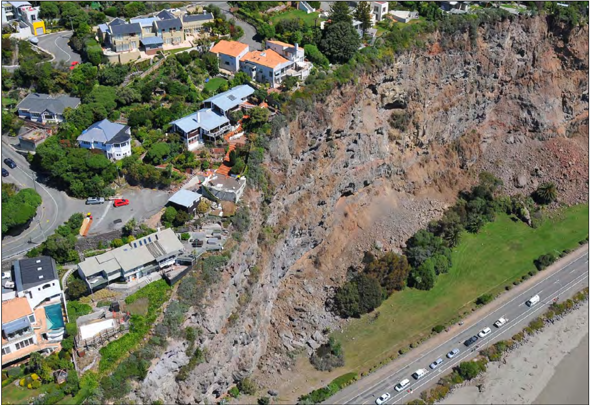
Photo 11. Rock falls on cliff face below Kinsey Tce on to 'Peacocks Gallop' reserve along Main Road between Sumner and Moncks Bay ( GNS Photo-GTH_5745 ).
