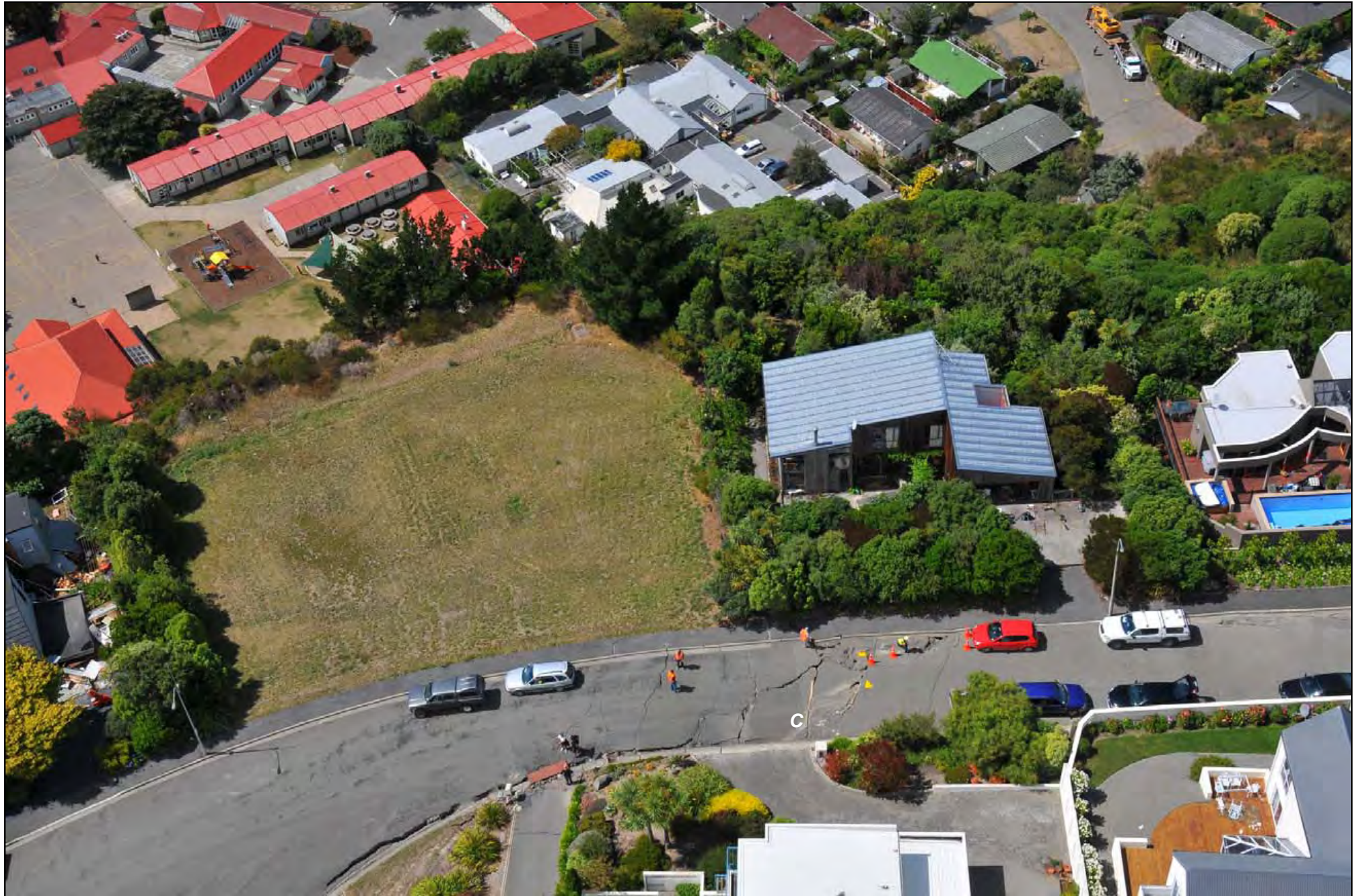
Photo 23. Cliff-top cracking (C) in Glendevere Terrace, Redcliffs ( GNS Photo-GTH_5819 ).
