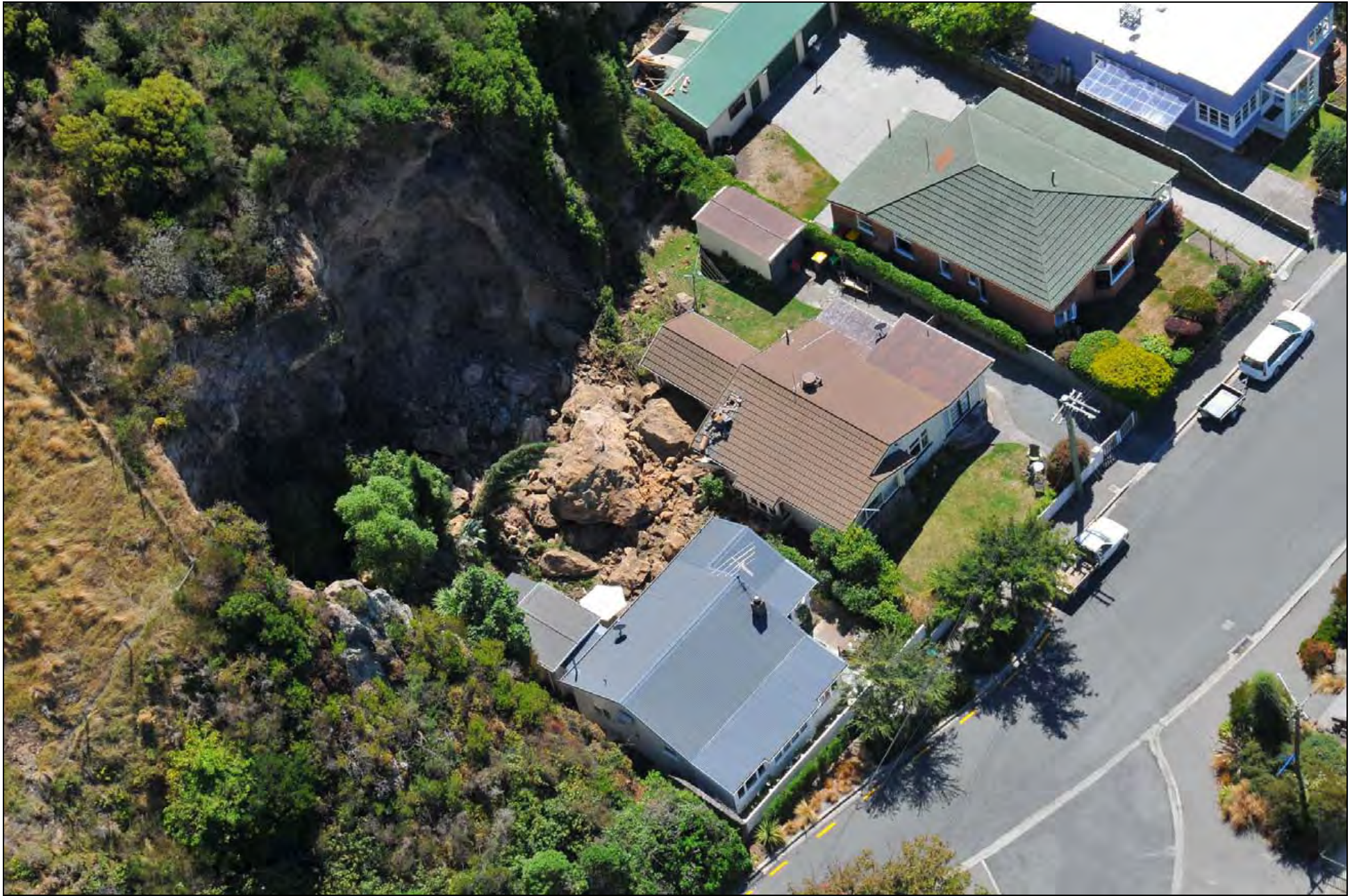
Photo 10. Fall of large boulders at the back of damaged houses at 11 (bottom) and 9 (centre) Richmond Hill Rd, Sumner ( GNS Photo-GTH_5736 ).
