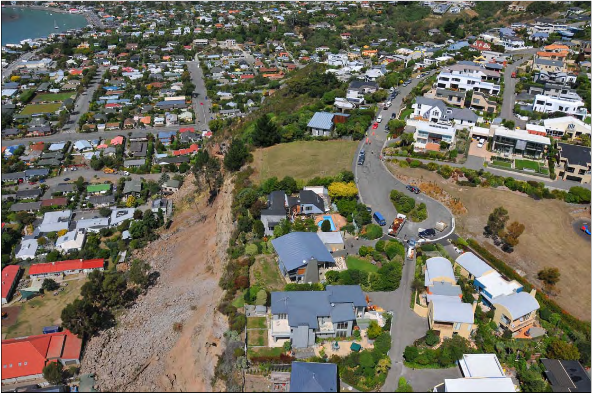
Photo 21. Rock falls on cliff behind Redcliffs School below Glendevere Terrace at Redcliffs ( GNS Photo-GTH_5814 ).
