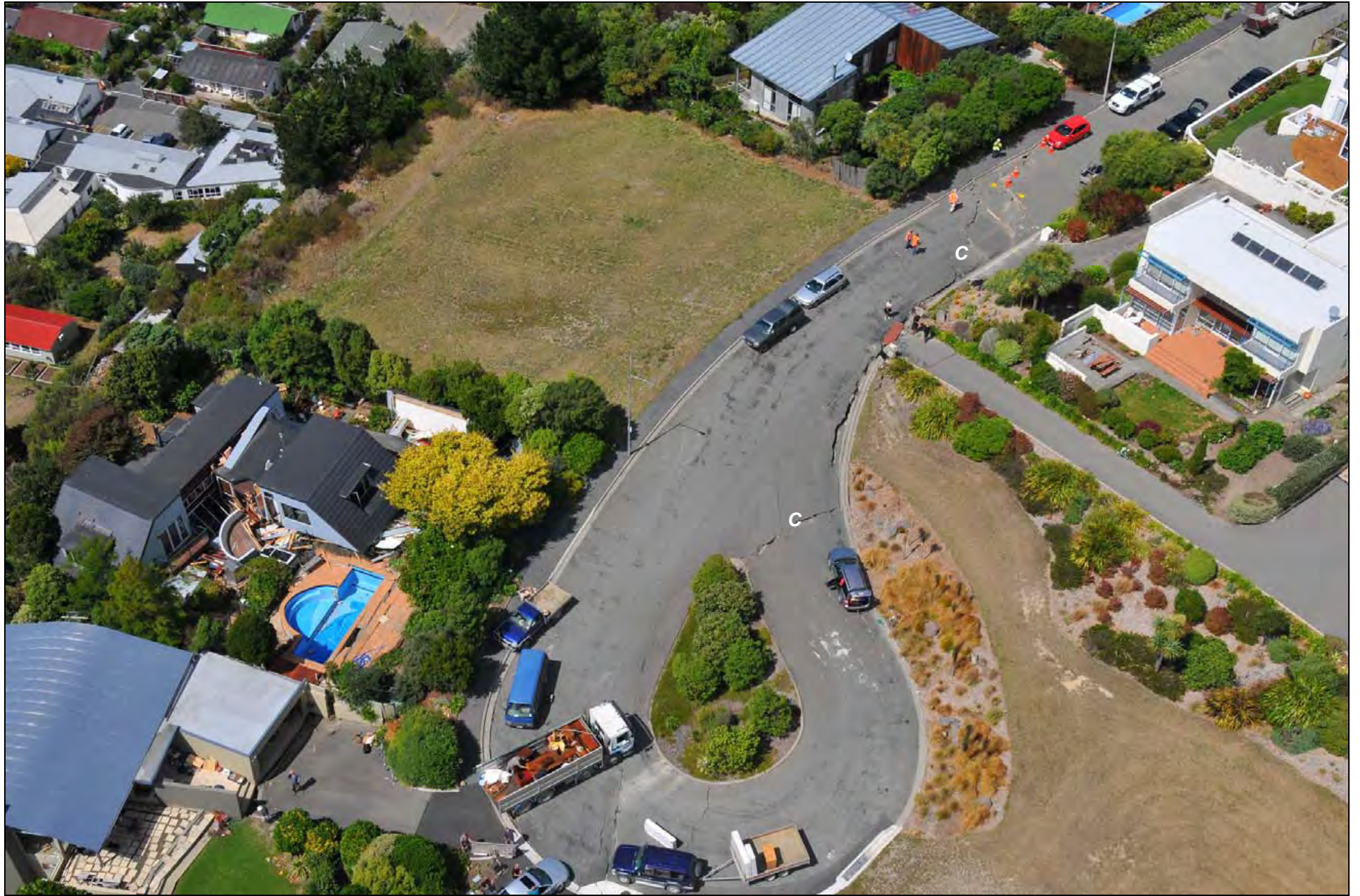
Photo 22. Cliff-top cracks (C) in roads and affecting properties in Glendevere Terrace, Redcliffs (GNS Photo-GTH_5816).
