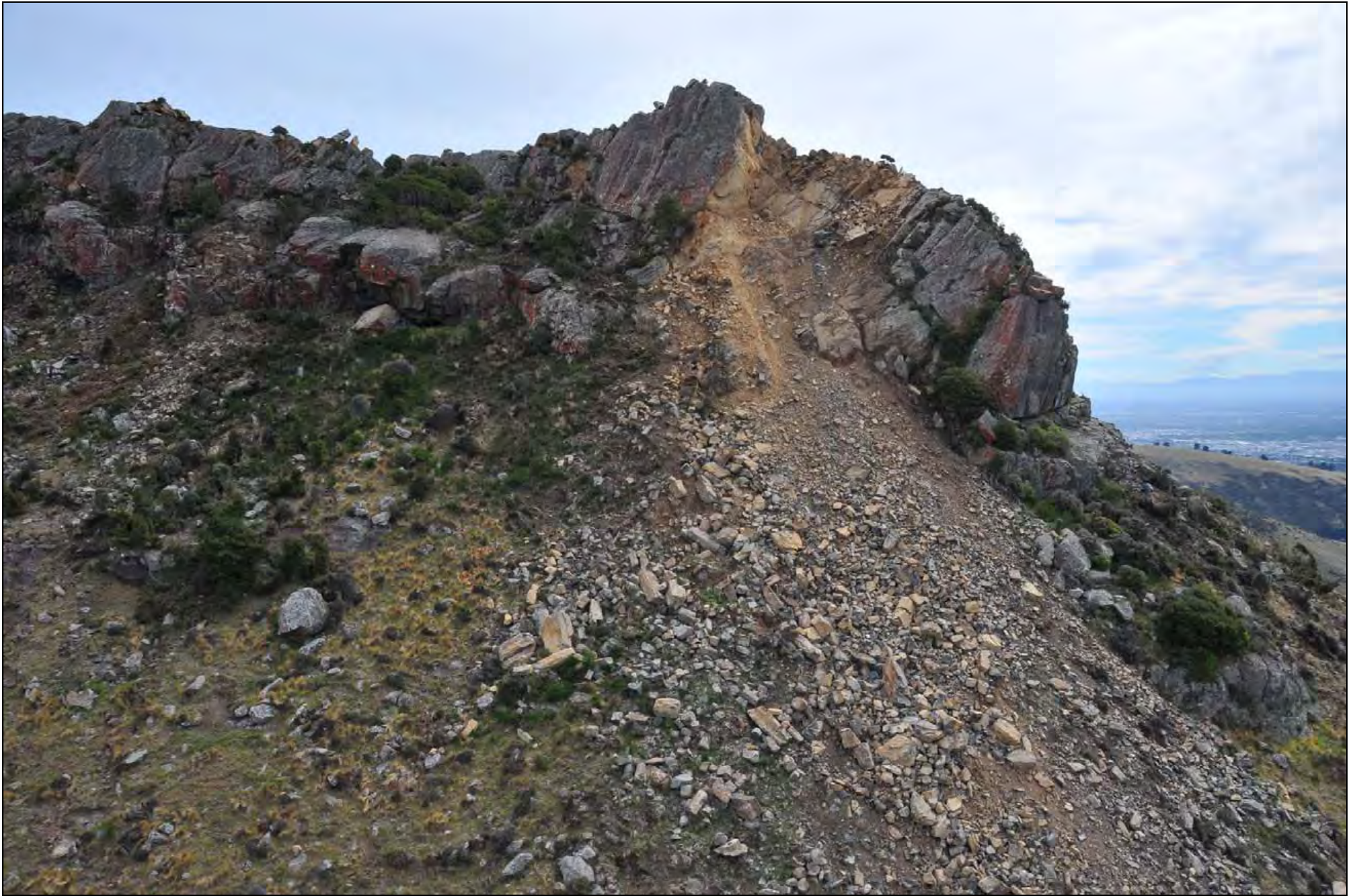
Photo 32. Rock falls from Castle Rock on to old talus slope. Most are from the 4 Sep 2010 earthquake, with some from the 22 February event ( GNS Photo-GTH_6017 ).
