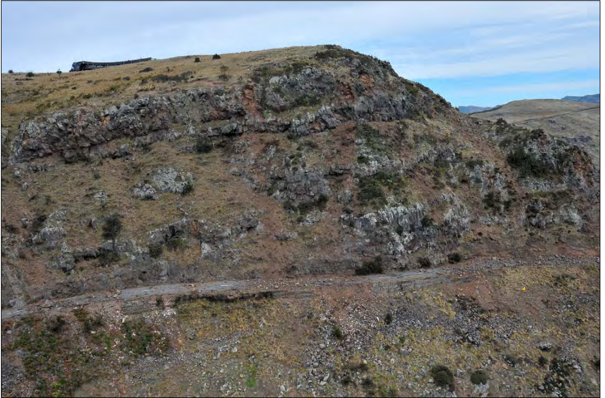
Photo 30. Numerous small rock falls from lava bluffs on to Summit Road near the Gondola Building ( GNS Photo-GTH_5993 ).
