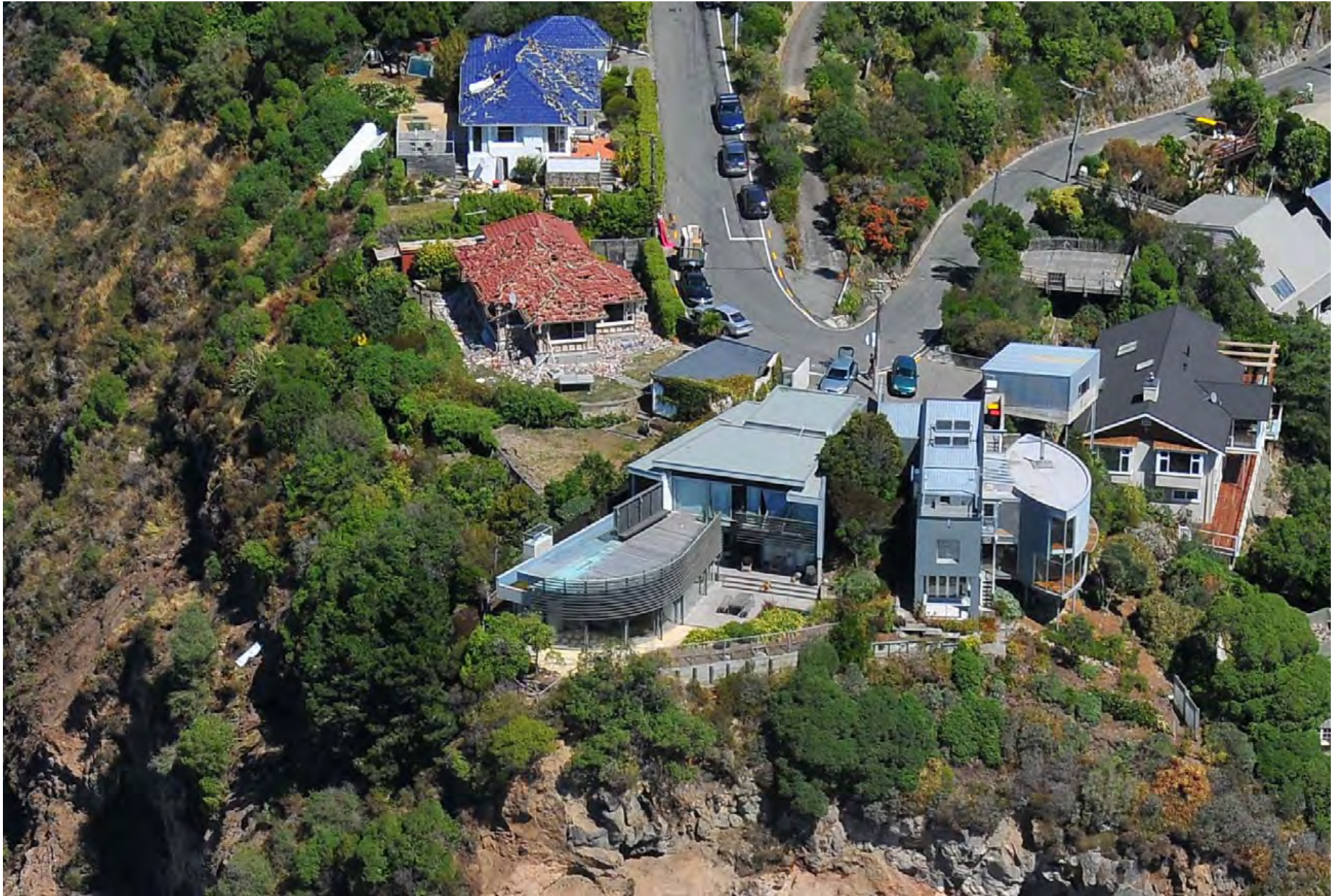
Photo 8a. Houses on Richmond Hill Road badly damaged by strong shaking at top of 50 m high cliff above RSA building at Sumner ( GNS Photo-GTH_5723 ).
