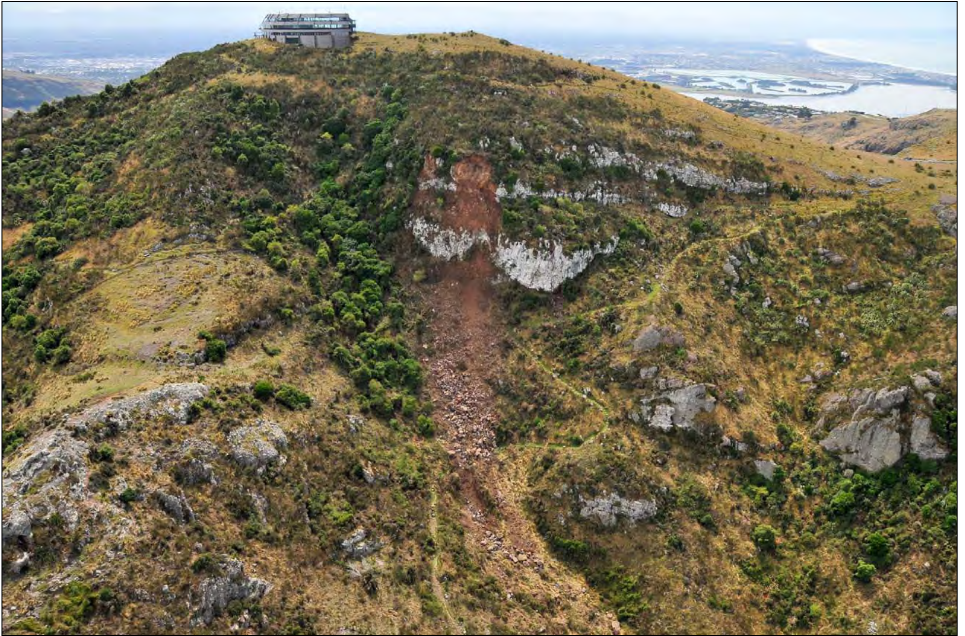
Photo 29. Rock fall on slope and walking track below Gondola Building (possible fatality site) ( GNS Photo-GTH_5933 ).
