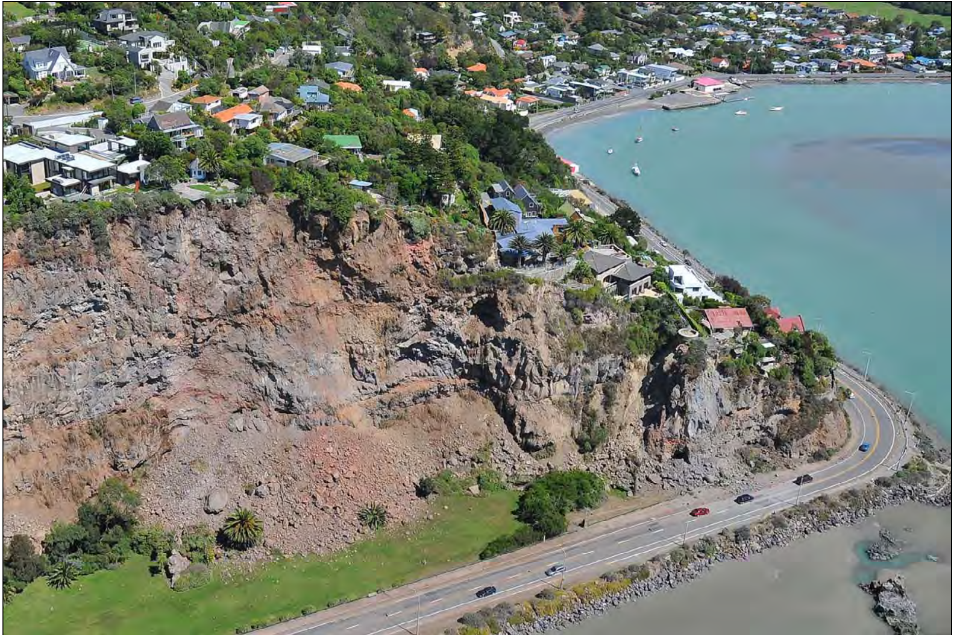
Photo 12. Rock falls on cliff (a former quarry site) below Kinsey Terrace on the Main Road between Sumner and Moncks Bay (right). (GTH_5749).
