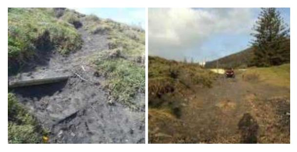
Photograph 14: Concrete telephone poles showing through eroded areas of sand dune below the car park Photograph 15: Vehicle access to the beach at the southern end covered in debris washed in from storms.
