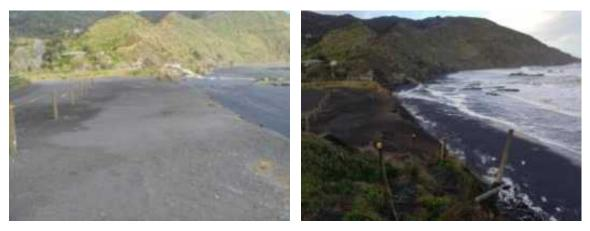
Photograph 6: Failing car park edge looking south (low tide). No pedestrian access to the beach available from this car park now. Photograph 7: Failing car park edge looking south (high tide). No pedestrian access to the beach available from this car park now.
