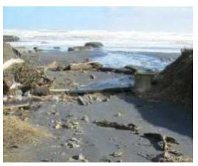
Photograph 12: Site visit in 2014 showing stormwater culvert being covered by further sand.
